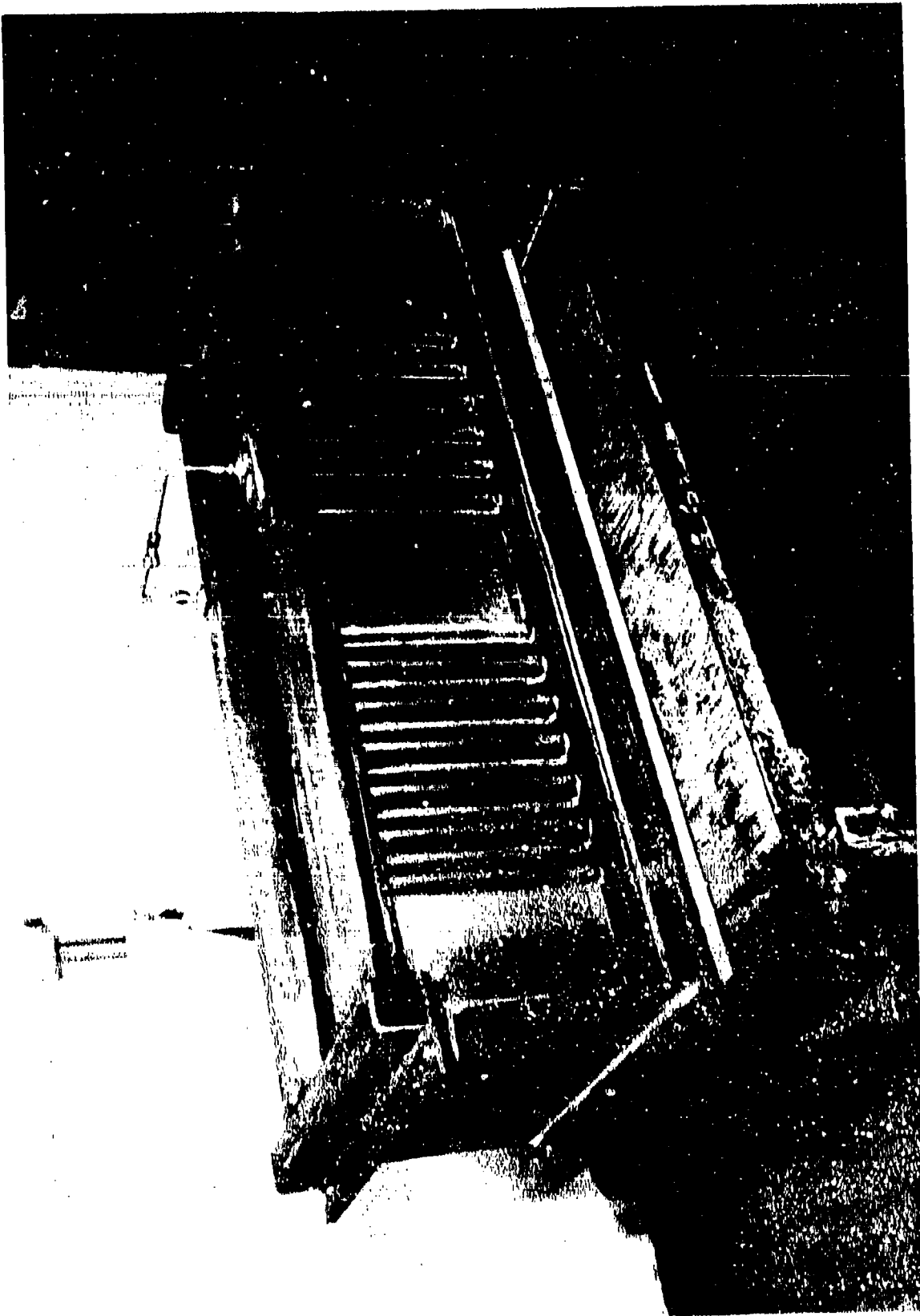
Figure 40. 40-Inch Box Beam Element 1 in Final Cure Assembly with Manifold
