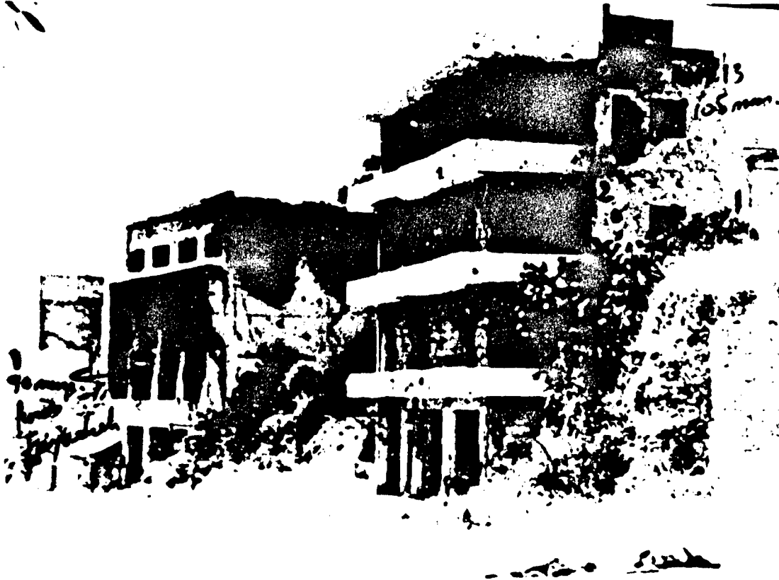
Weapons' effect on building at Tel Zaatar. Front of building damaged by 90mm cannon on Panhard fired from Fayadiyeh. On side of building top larger hole created by AMX-13 105mm cannon, lower hole by 40mm cannon on M-42.
