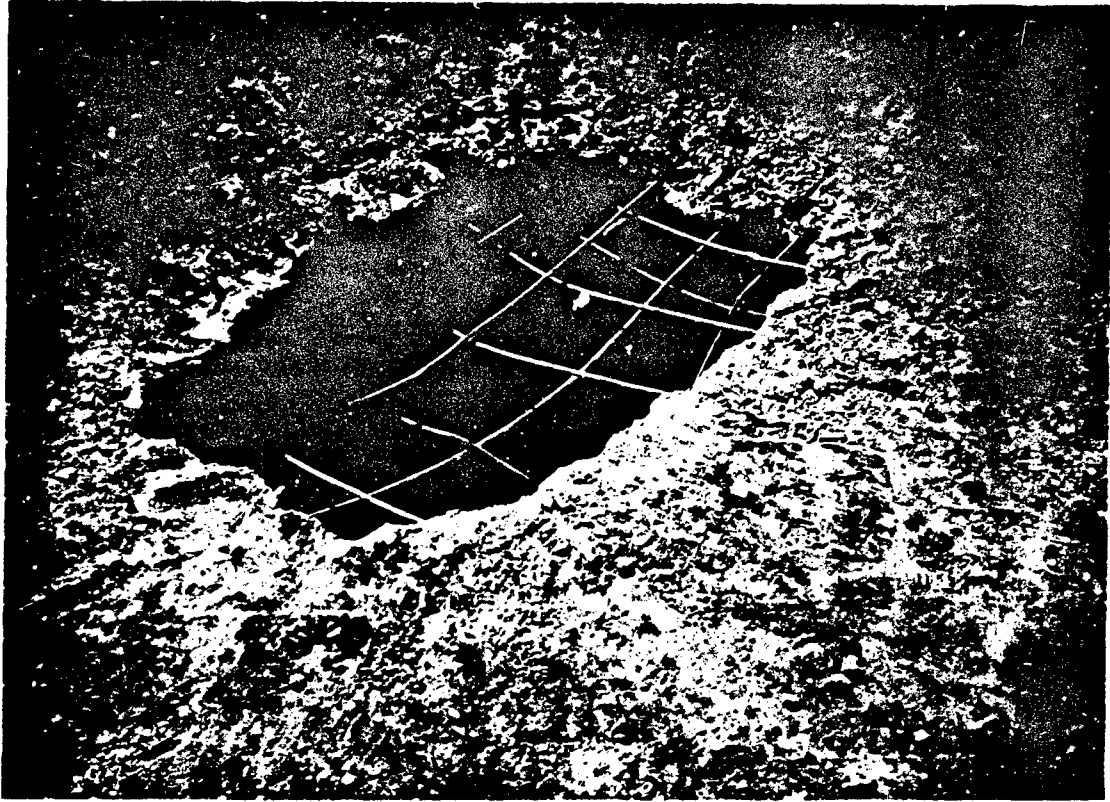
Hole created in roof top by 122mm shell (Syrian)
