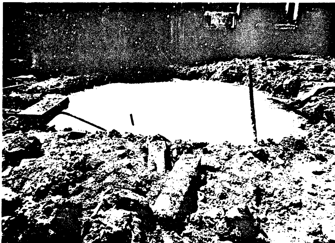
Crater filled with water as a result of 160mm mortar shell hitting water main in Ashrafiyeh.
