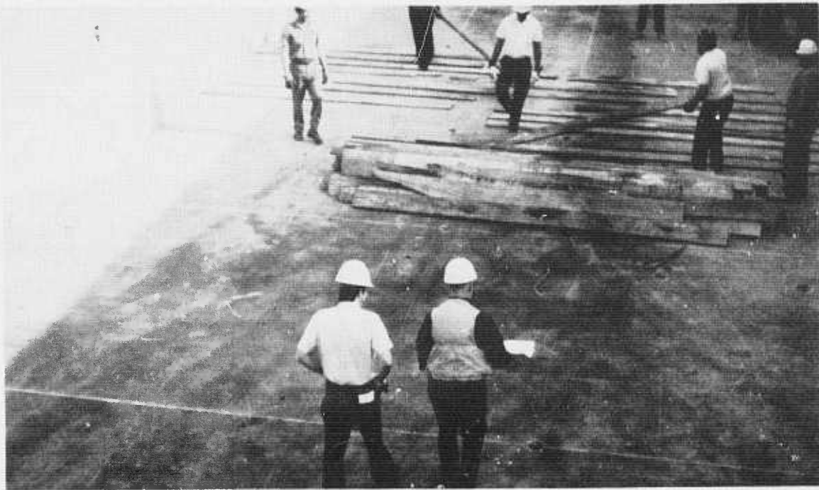
Figure 8. "Floating" Deck Being Laid Athwartship.
