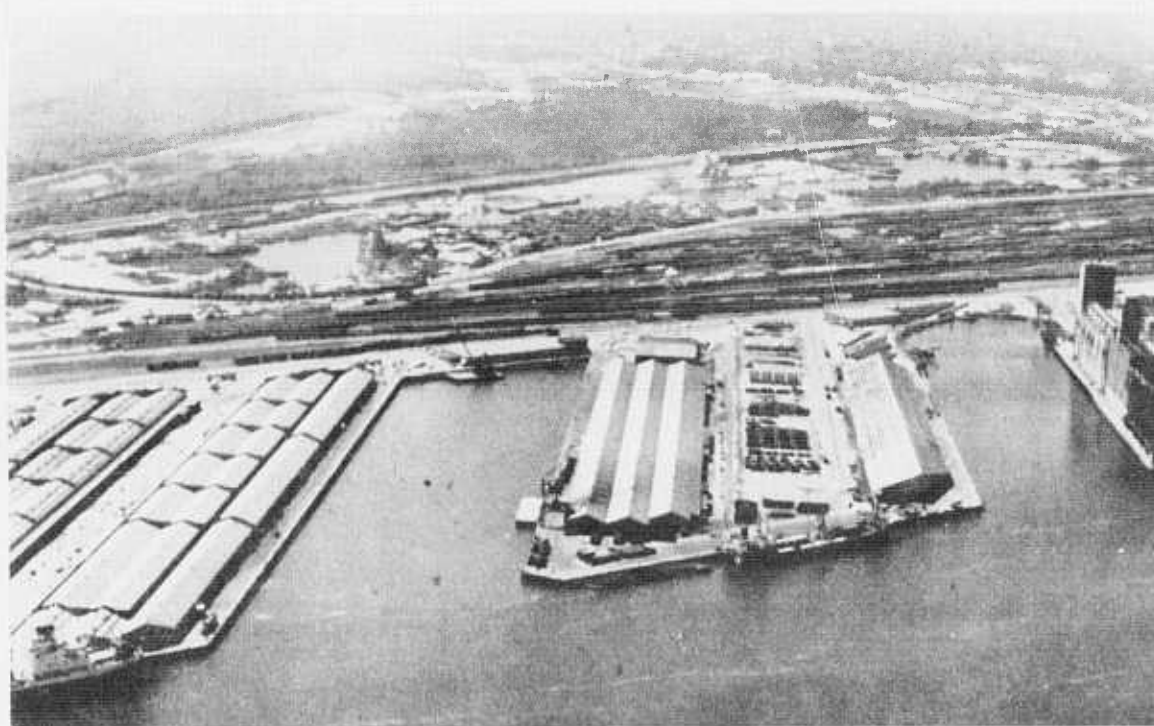
Figure 3. Pier C, Alabama State Docks.
