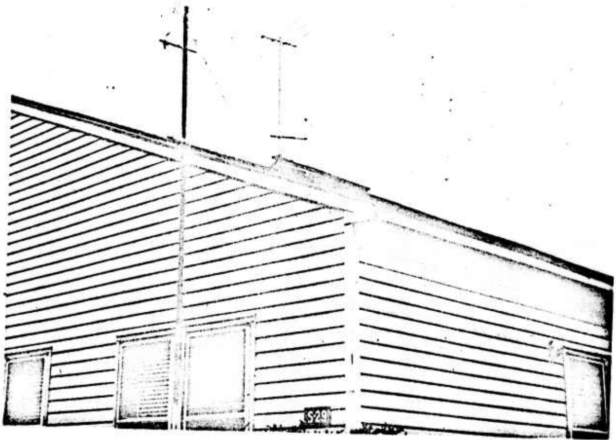
Fig. 4. TV antenna on Bldg. S-29, Evans Area.
