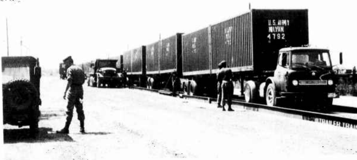
Figure 6-7. MILVANS and Chassis Loaded on Trailer-on-Flatcars.
