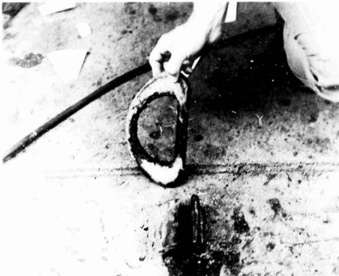
Figure 8-64. Defective "D" Ring on the Main Deck GTS Callaghan .
