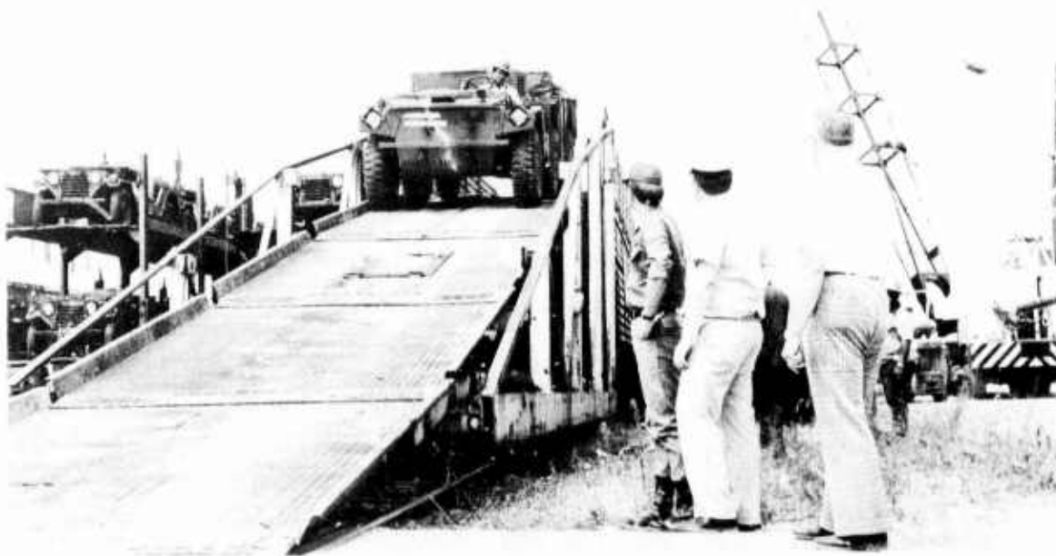
Figure 8-21. Bilevel Railcars Unloading Utilizing Mobile Ramp Provided by the Norfolk & Western RR.
