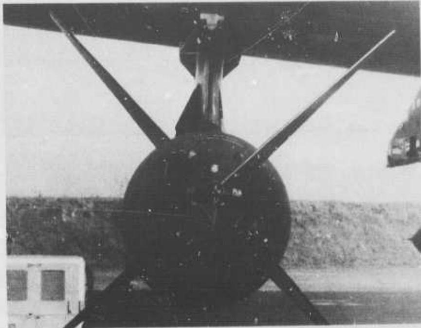
Figure 11. Metal ballast installed
