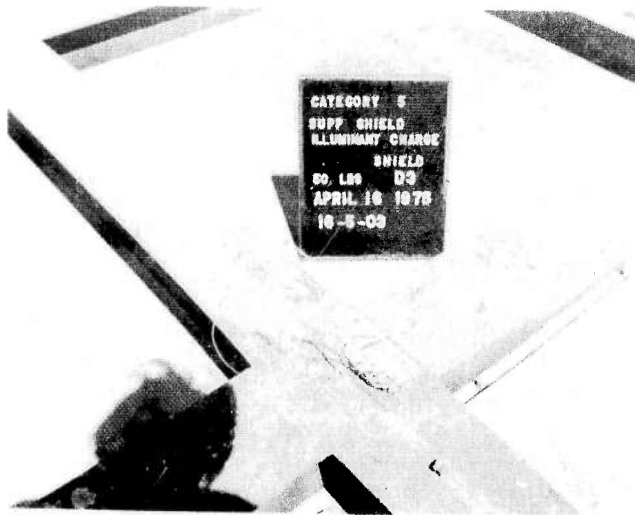
Figure 23. Post Test Exterior Roof View.
