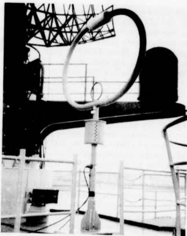
Figure 13. MLA-1 Miniloop installed aboard USS BRADLEY (DE 1041).
