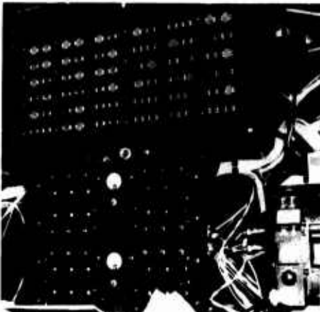
Fig. 2.9 Selector Panel, Aft Crew Compartment, B-36
