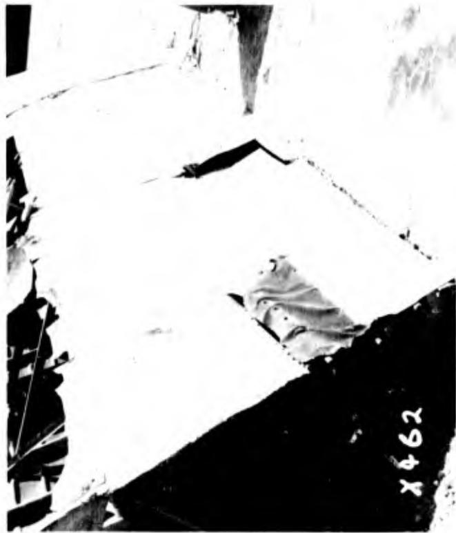
Fig. D. 57 B-36 Wing Section Range 4800 ft (5.7 psi), Shot 9, Showing General Skin Damage at Outboard Extremity
