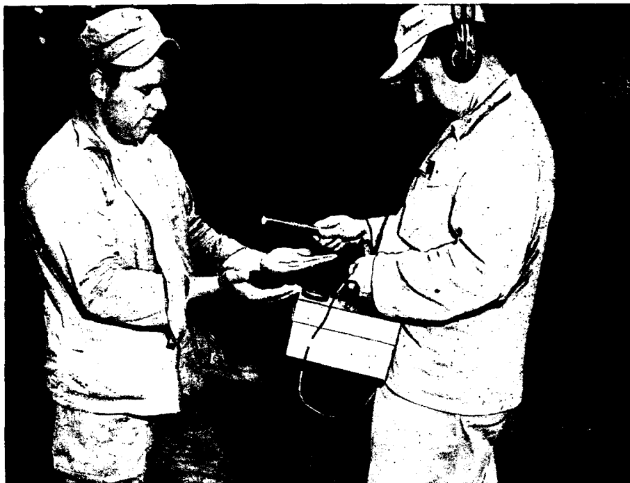
Figure 46. Checking hand contamination.
