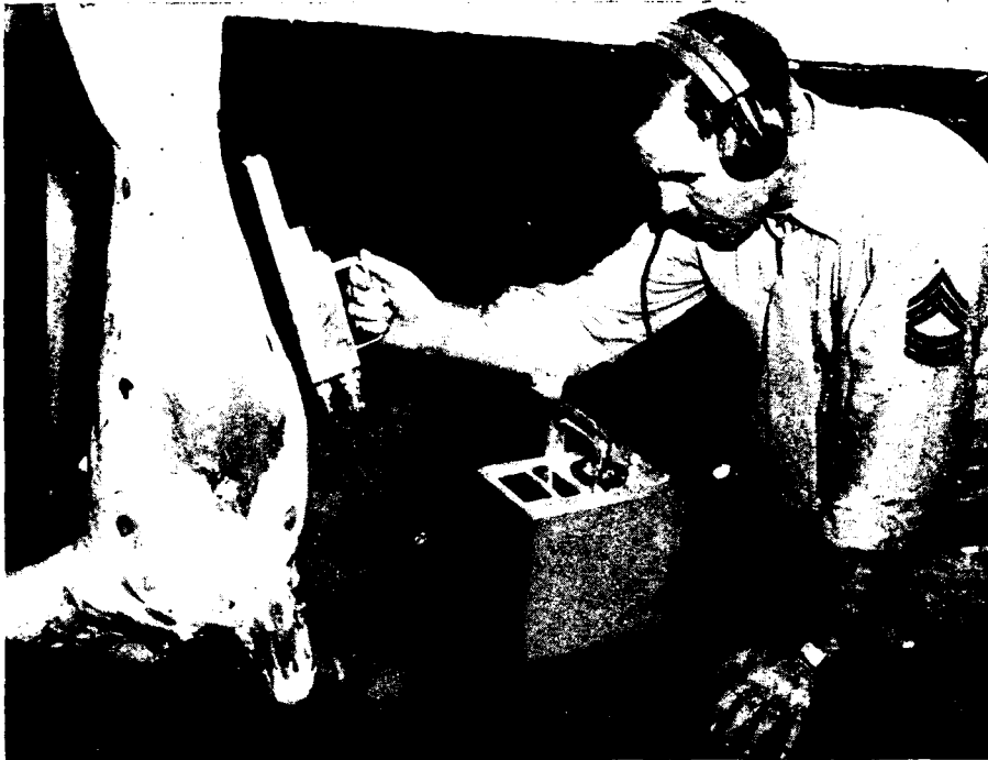
Figure 40. Checking meat for alpha contamination with a poppy-type portable proportional counter.
