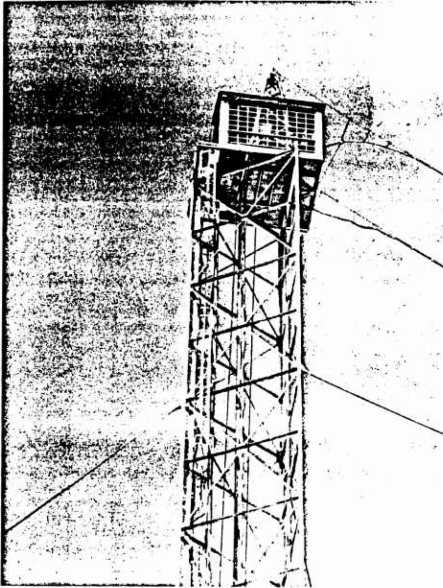
Fig. 39—Typical catenary installation.
