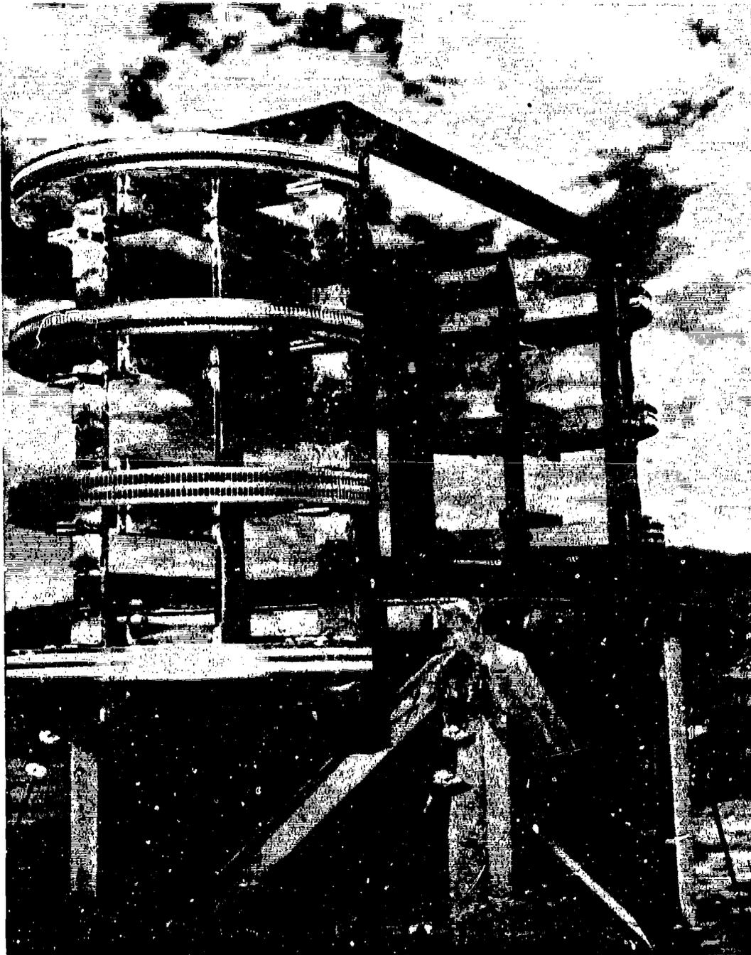
Fig. 2.8 - Field Installation of Cosine Law Attenuator Calorimeter,
