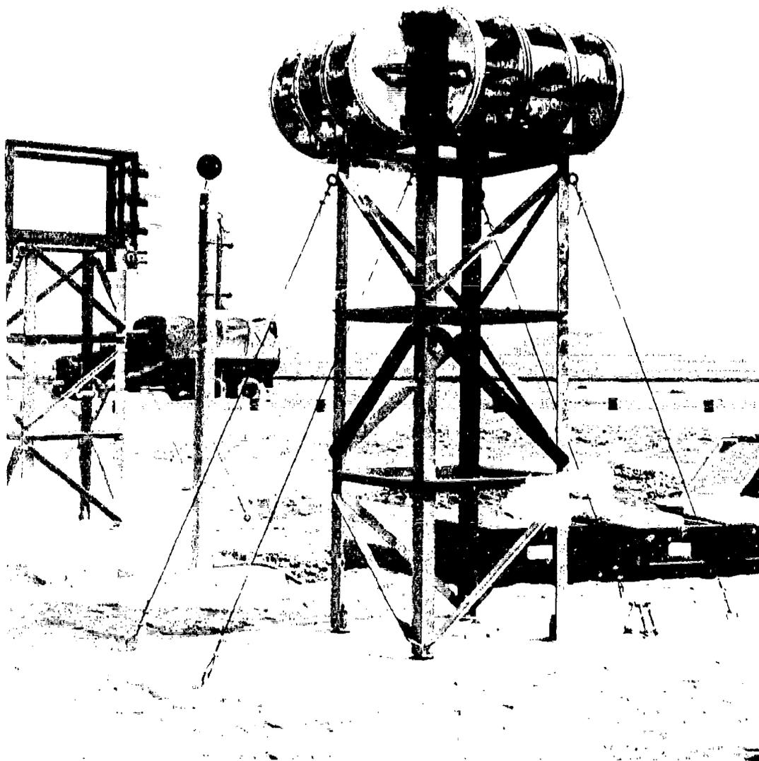
Fig. 2.9 - Field Installation of Cosine Law Attenuator Calorimeter,
