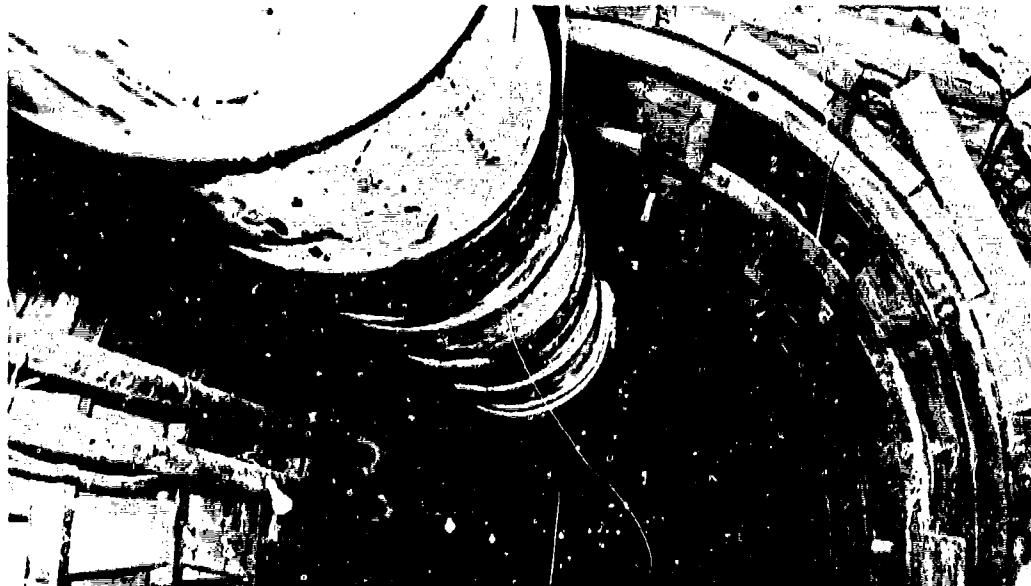
Figure No. 6. Steel Supports in Side Drift U-12e.05
