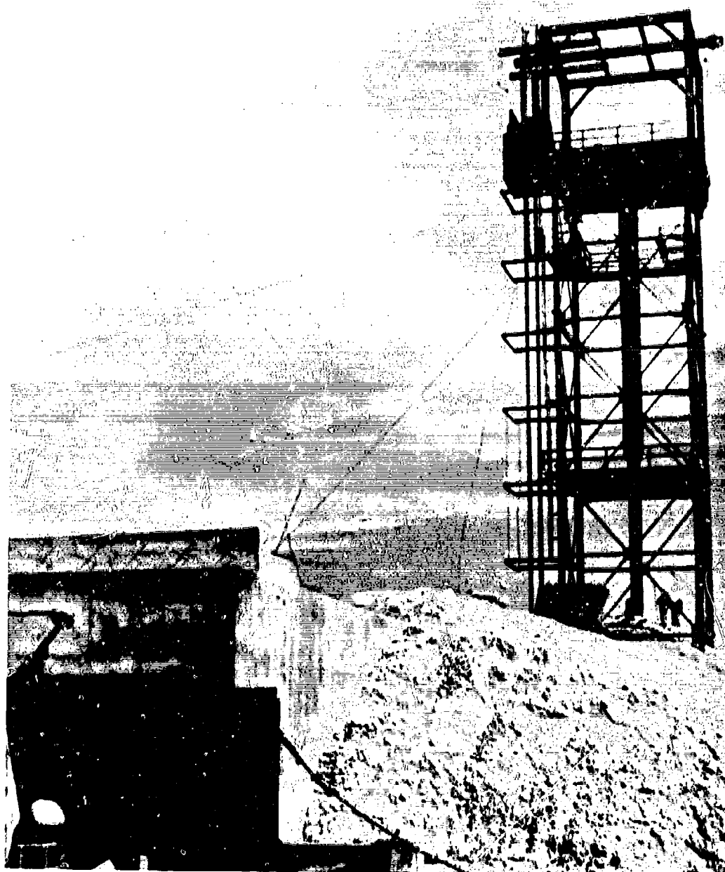
Figure No. 12. Tower Station T-7c and Base Structure Station 7-313
