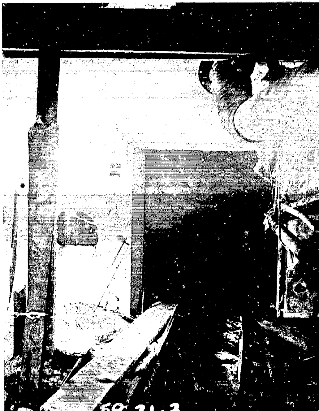
Figure No. 23. Concrete Encasement for Blast Door in Side Drift U-12b.02
