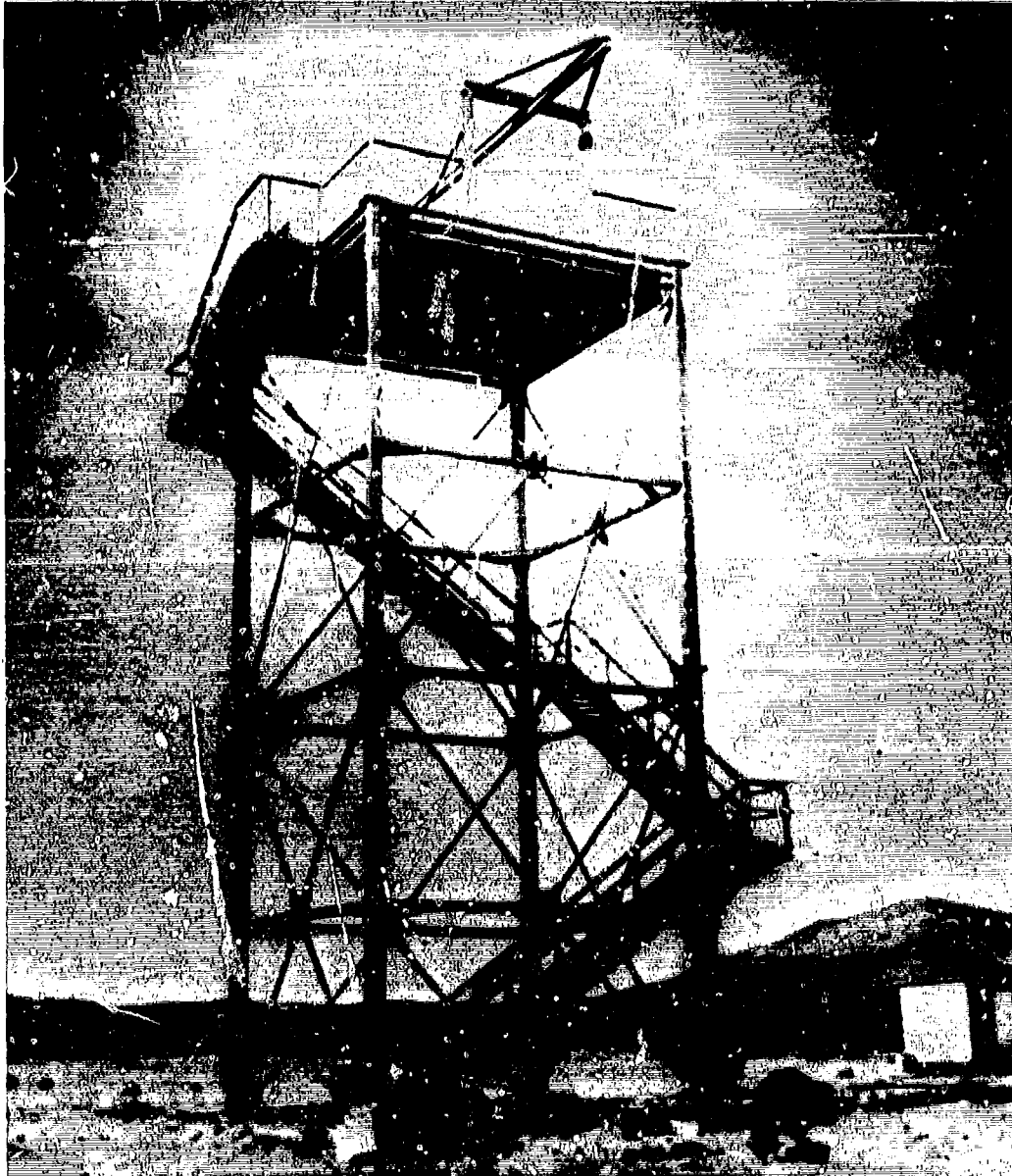
Figure No. 19. Station T-9d Prior to Installation of Prefabricated Cab
