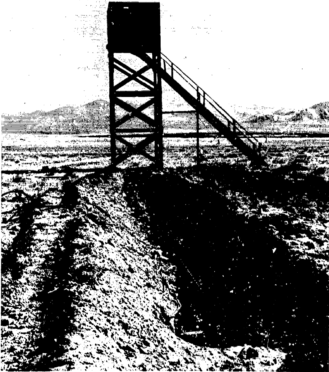
Figure No. 15. Station T-8c Showing Power Cable Trench from Transformer to Tower
