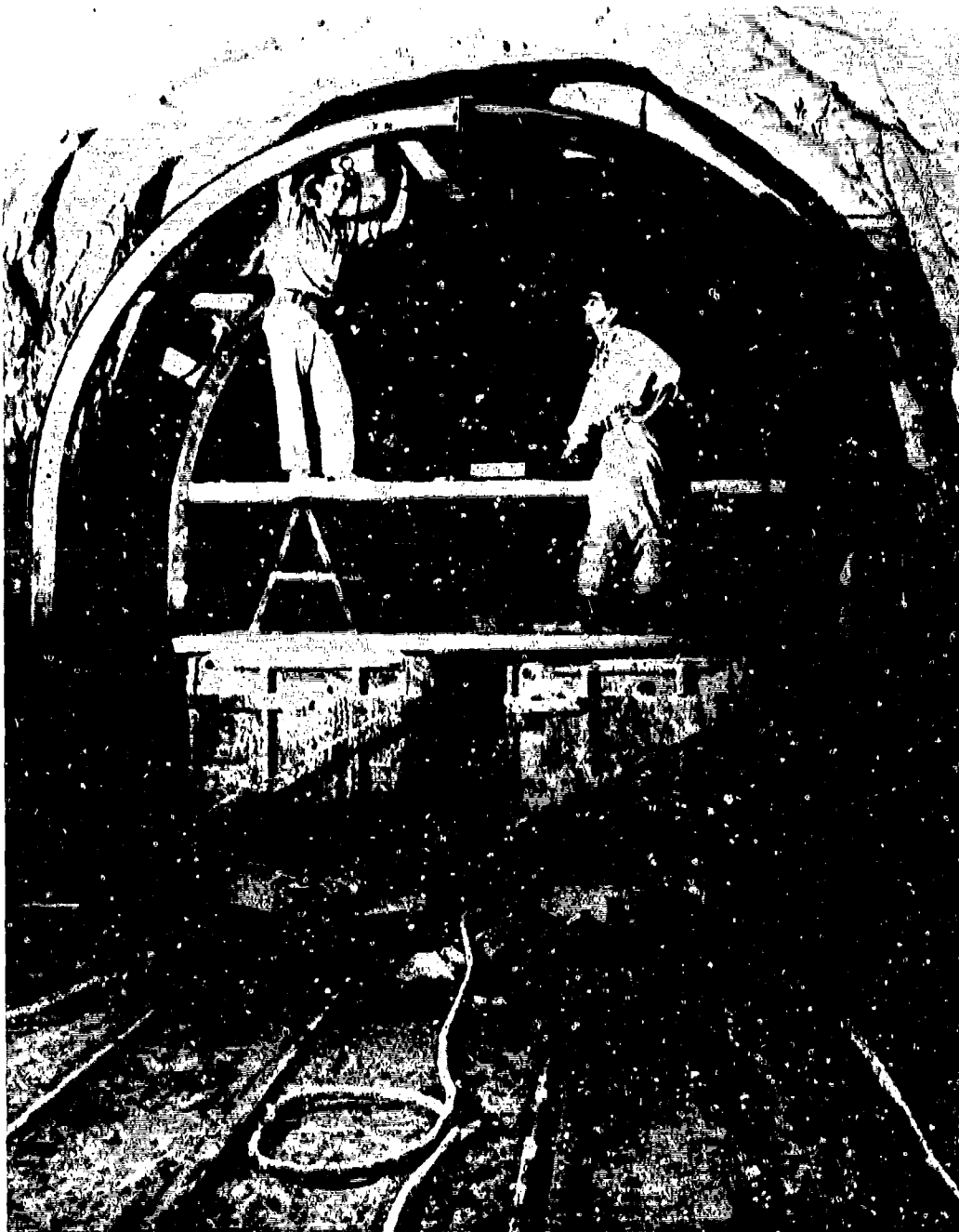
Figure No. 26. Steel Sets at Station 12 + 17 — Tunnel U-12e
