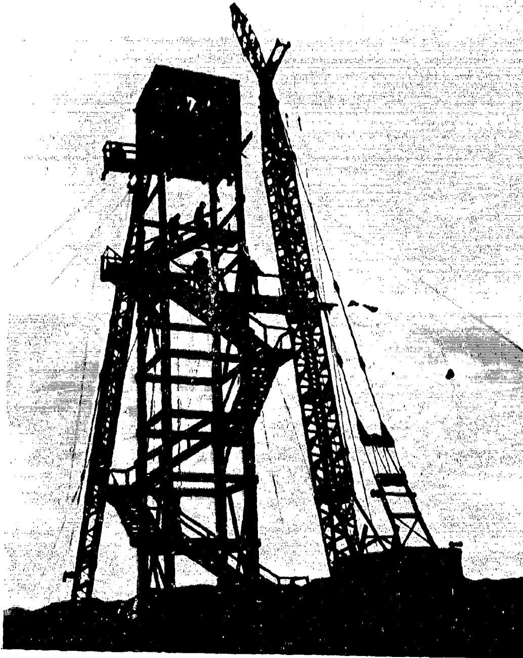
Figure No. 8. Station T-3t — 90% complete
