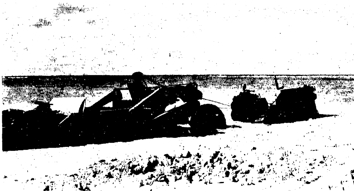
Figure 2-151. Recovering Fill Around Man-Made Island No. 3
