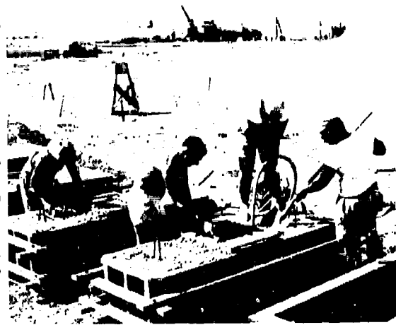
Figure 2-92. Prefabricating Footings for Stations 1811 and 1812
