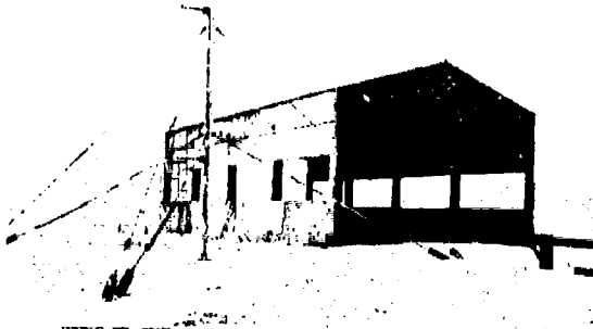
Figure 2-56. Stations 311.03 with 313.06 in Foreground
