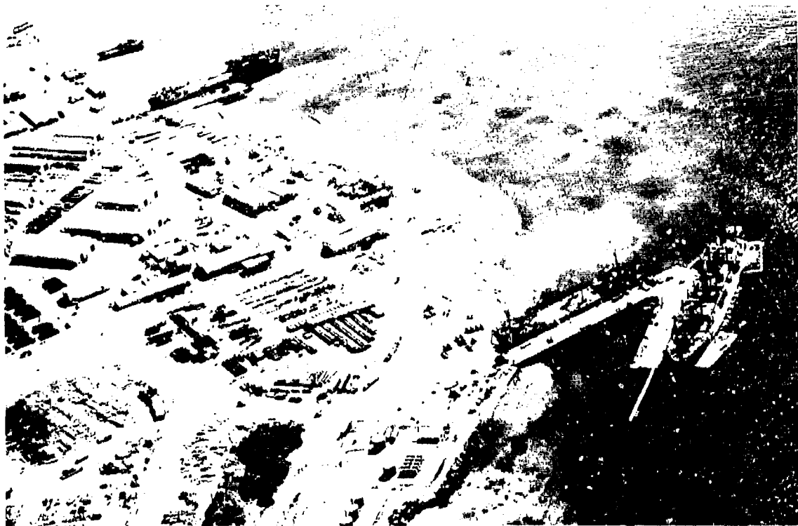
Figure 3-12. All Off-Loading Berths Occupied
