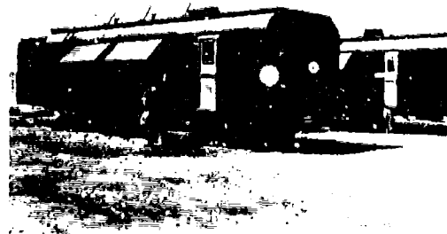
Figure 4-18. 600 KW Generators - Under Load Test
