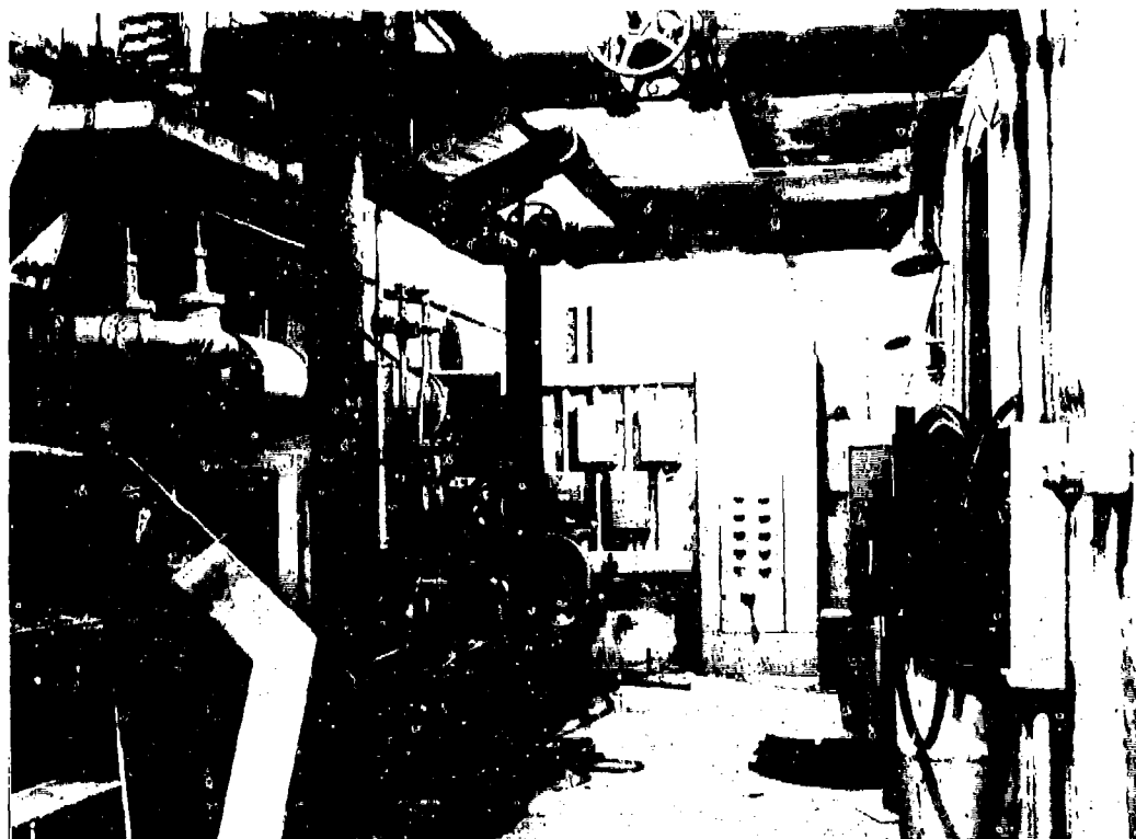
Figure 2-98. Station 2201 - Utility Room
