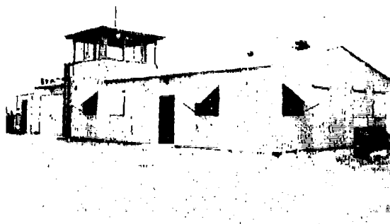
Figure 2-138. Operations Building - Nan Airport
