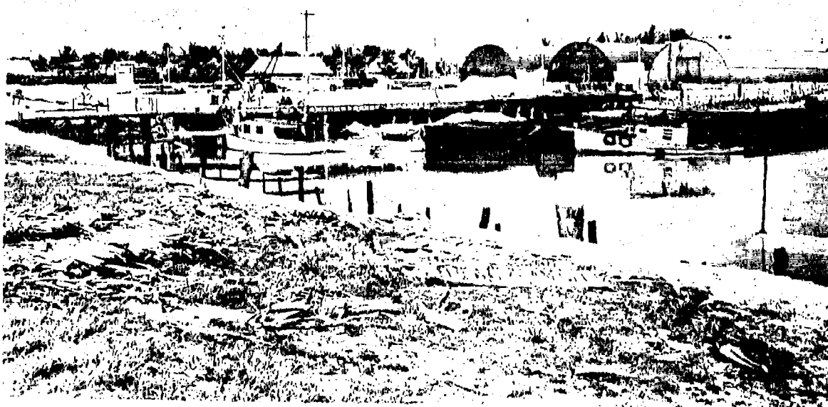
Figure 2-180. Pier Facilities - Betio Island, Tarawa
