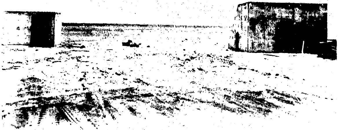
Figure 2-43. Station 75.01 (Right) - 65% Complete - Old Station (Left)
