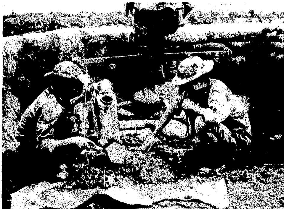
Two CIDG dependents at Duc Lap CIDG Camp mix concrete to cap the bunker in the background. Cement, like all other items, was supplied to many CIDG camps by airlift, the sole source of outside supplies.
