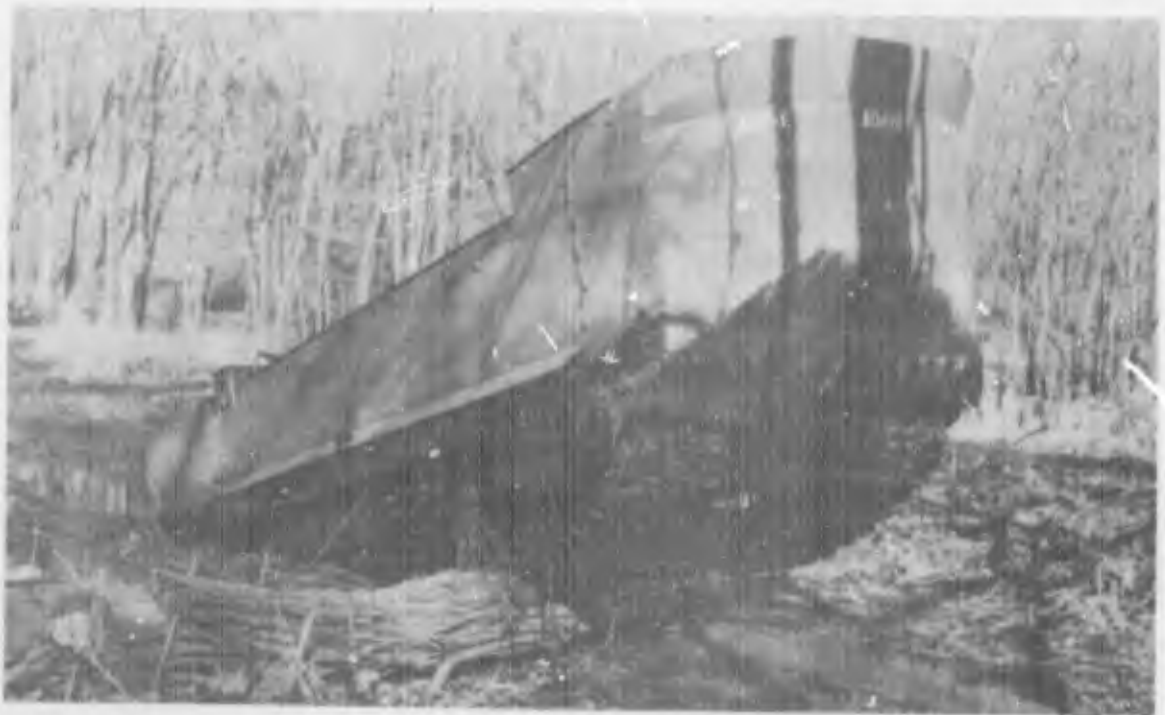
FIGURE F. The M29C Cargo Carrier going over the same log shown by Figure E.
