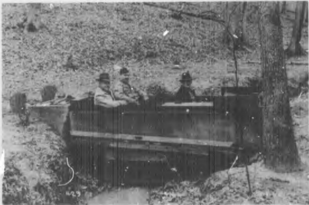
FIGURE H. The M29C Cargo Carrier in the same ditch shown by Figure G.
