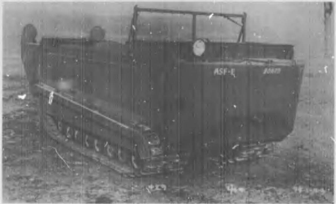
FIGURE A. The M29C Cargo Carrier prepared for land operation with rudders up and front splash shield back.
