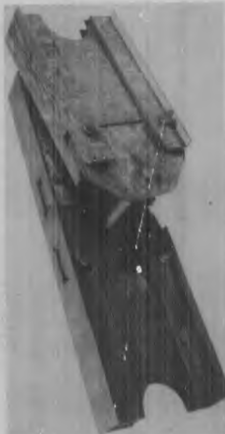
Special hinge panel attached to balk to form a hinged joint.
