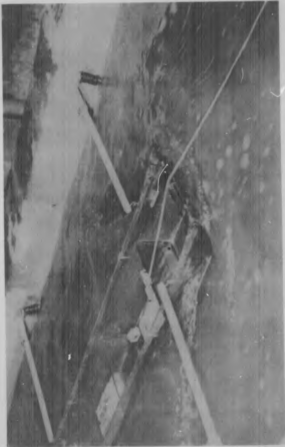
FIG. 87. FLOW CONDITIONS FOR AMERICAN 25-TON PONTON. Average freeboards for velocity of 7.3 feet per second and 10-inch loading. Bow - 4.25 inches; side - 7.50 inches.
