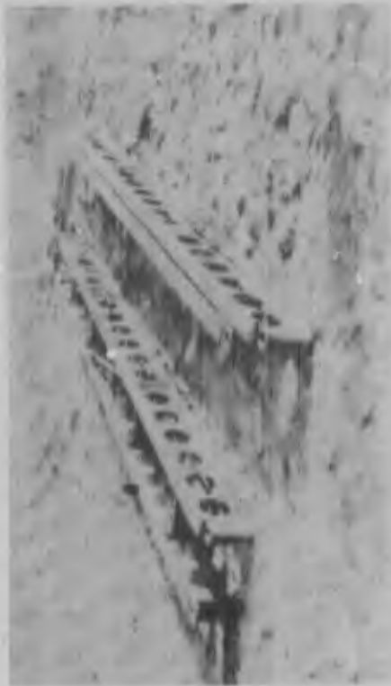
Balk ready to be placed in bridge superstructure. Each end of the balk has a male and female joint.
