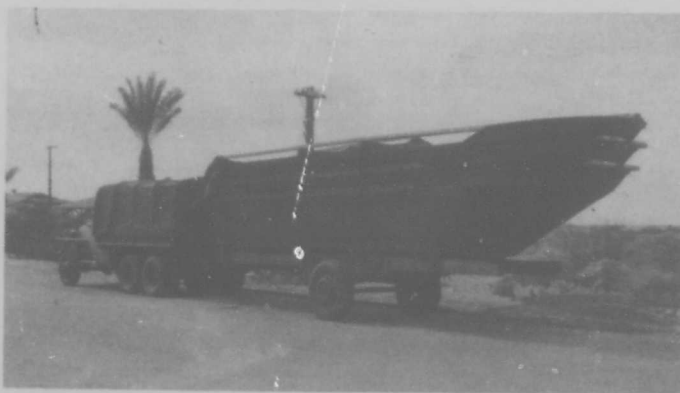
FIG. 8. TRANSPORTATION OF THREE HALF-PONTONS
