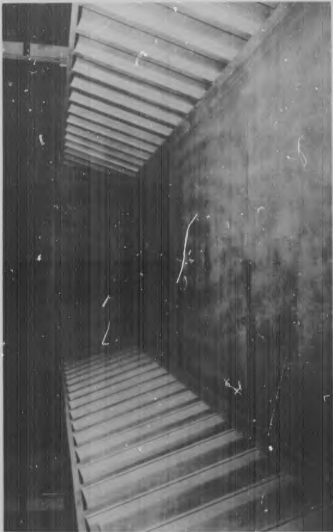
FIG. 41. INTERIOR VIEW OF PLYWOOD PONTON SHOWING FLOORING. Interior of a plywood ponton fabricated in the Engineer Bcard shops. Note the floor, which is watertight except at the sides. This feature adds greatly to the control of free water and the stability of the ponton when water is present inside.
