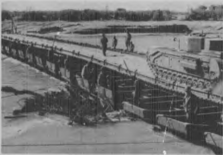
Debris passing under properly anchored bridge as 45-ton tank passes over bridge. Note bridle lines and shore guys.
