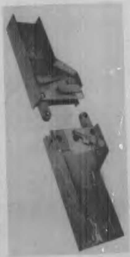
Locking pins and shear lugs have been removed and balk are separated longitudinally without turning links into balk ends. Links are tapered to aid in making a connection.
