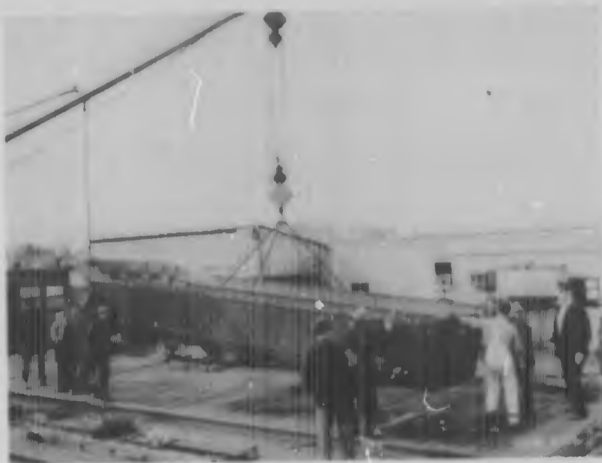
FIG. 67. METHOD OF LIFTING PONTON. Lifting a plywood ponton weighing 1,691 pounds using a 4-part bridle around the four cleats in the boat. This is a satisfactory method of lifting providing the cleat bases are stiffened somewhat.
