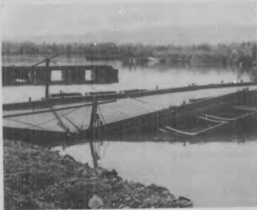
Improper trestle footing caused failure.
