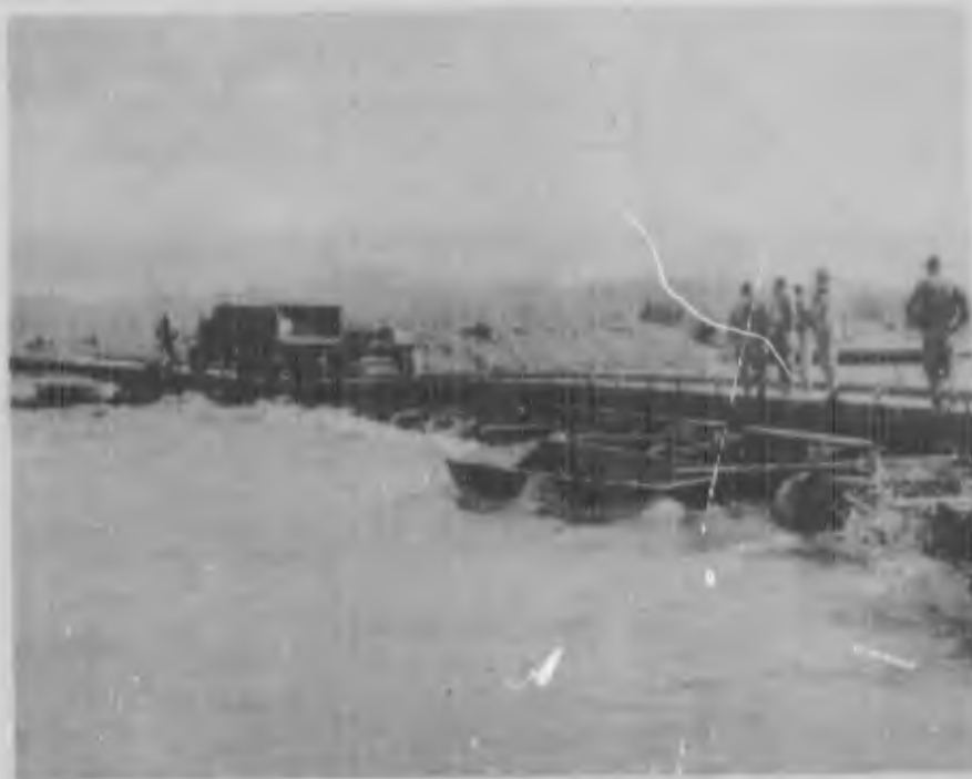
Lack of shore guys caused failure.
