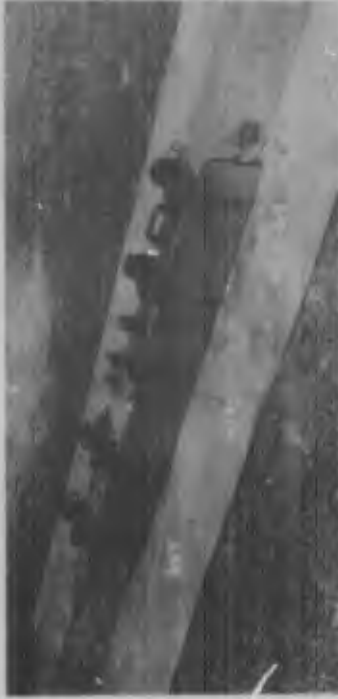
Two ponton balk inserted in connector to form a continuous beam.
