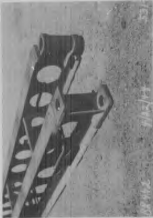
Balk ready to be placed in bridge superstructure. Each end of the balk has a male and female joint.
