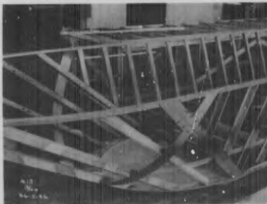
FIG. 36. BOW FRAMES. Another view of bow framing.
