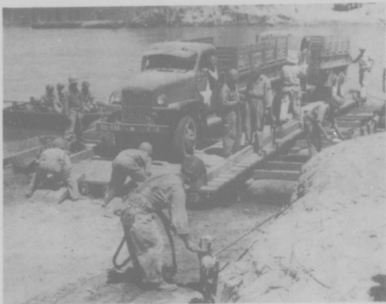
Proper use of holdfasts during ferrying operations.
