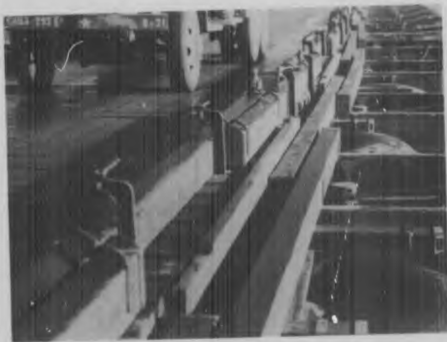
Placing chews on edge between outside balk and floor prevents deck chess from moving sideways.
