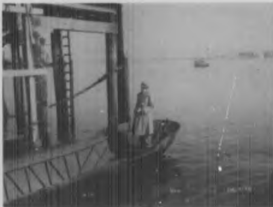
FIG. 70. GENERAL VIEW OF CONNECTOR TEST. Another general view of the bow of a ponton during connector tests. The ponton has a displacement of 32,000 pounds as shown.
