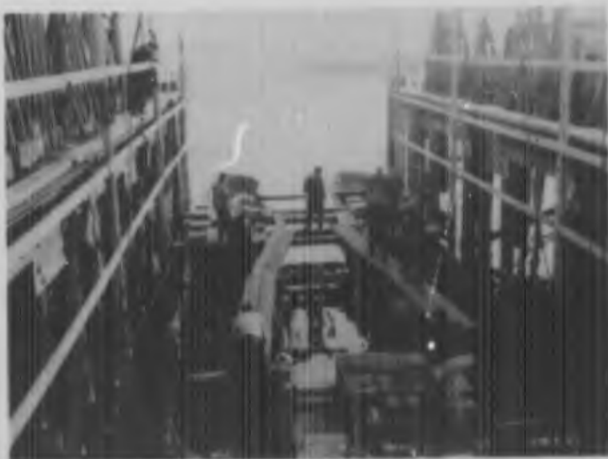
FIG. 68. LOADING TEST. General view showing loading test applied to Sparkman and Stephens ponton at the yard of Henry B. Nevins on 28 February.
