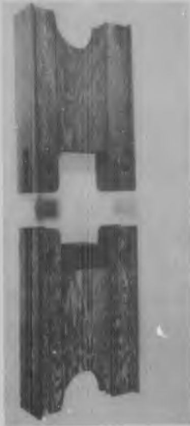
The moment panel has been turned back into the balk and the three pins inserted to secure the panel in place.
