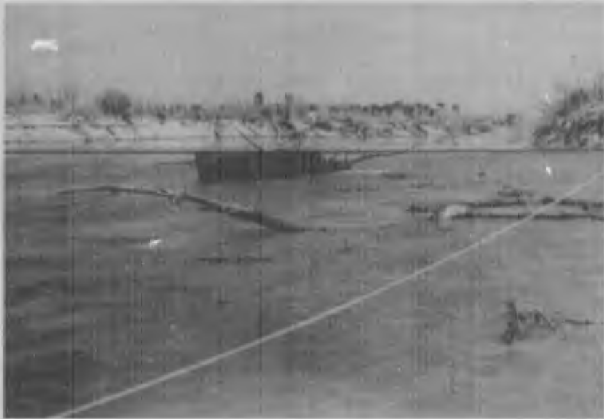
Pontons anchored upstream with one rope on five anchors must have men in them to clear lines. This ponton had none.
