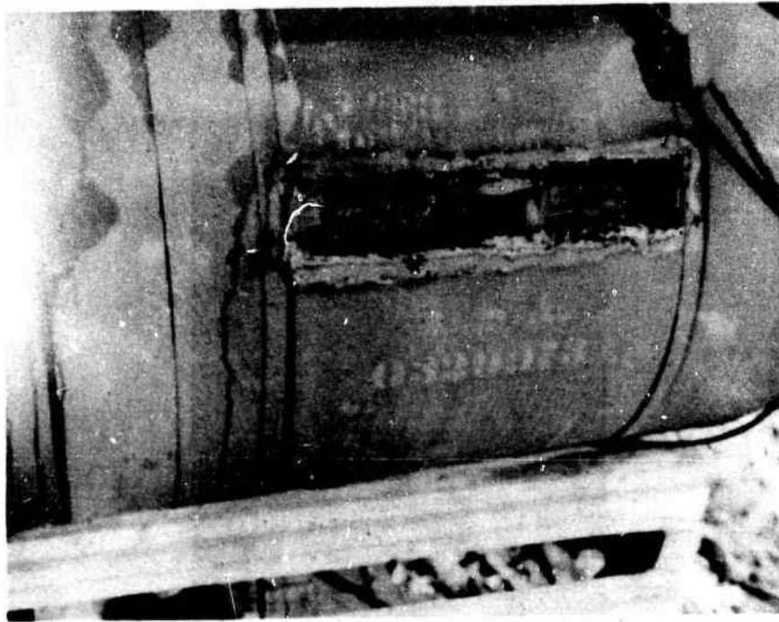
FIG. 161 JACKET AND ASBESTOS INSULATION CUT AWAY AND HOOK EYE WELDED TO TANK PROPER
