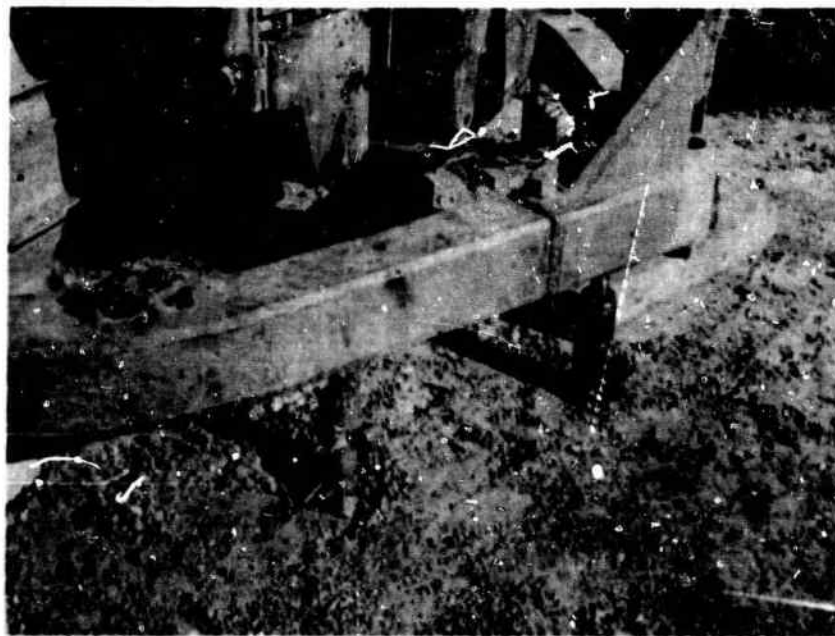
FIG. 2. DOZER YOKE, WHICH HAS BEEN CUT, REMOUNTED ON TRACTOR AND JACKED INTO PLACE FOR REWELDING.
