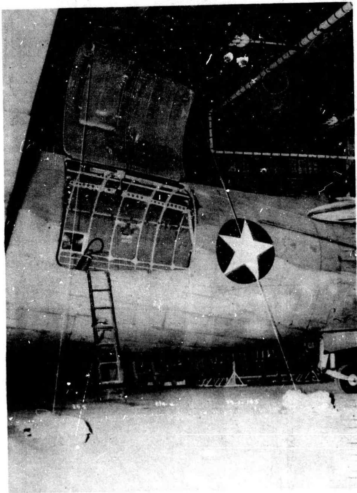
FIG. 10. CARGO DOOR IN POSITION FOR LOADING WITH SHEARS. Front view.
