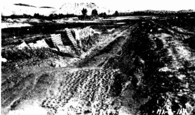
FIG. 9. ROADWAY OF PIERCED PLANK LANDING MAT ON PBS AFTER 877 TRIPS. Note position of the 5-foot lengths of plank. Foreground: 15-foot width section; Center: The 10-foot width on PBS; Background: Longitudinal plank in trackway.
