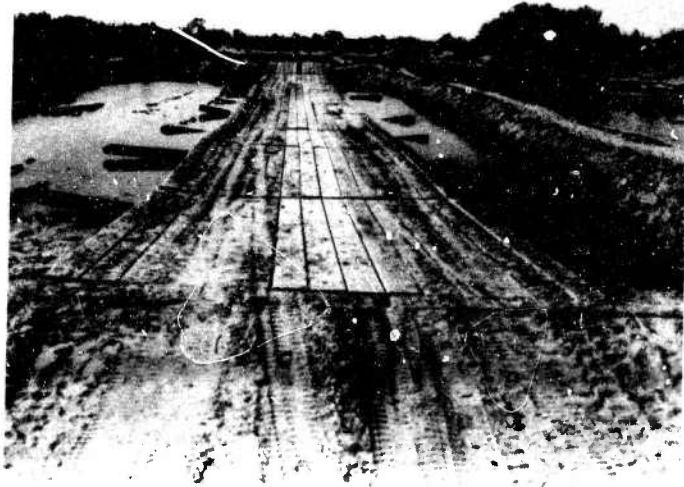
FIG. 7. ROADWAY OF DECK BALK FROM FLOATING BRIDGE, M4, AFTER 271 TRIPS. The outside row and the sixth row from each edge are pinned to the gunwales.
