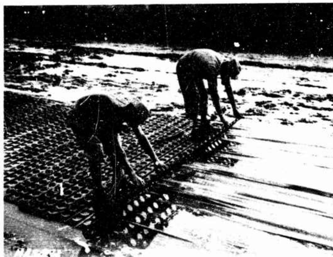
FIG. 11. LAYING PIERCED PLANK LANDING MAT ON UN-TREATED BURLAP.
