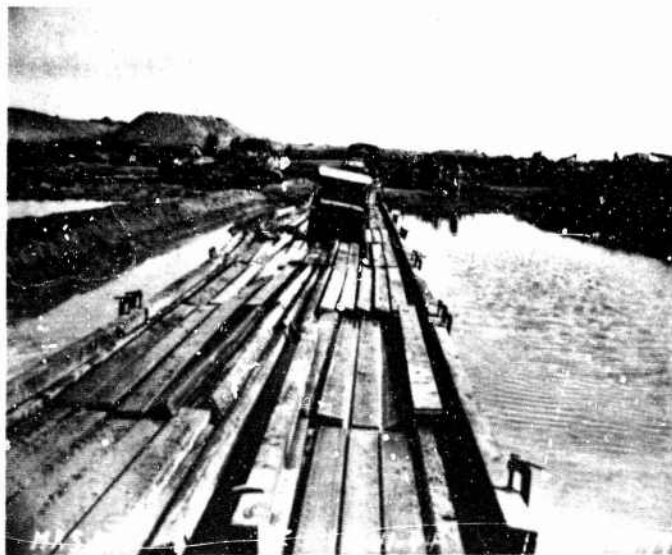
FIG. 6. DECK BALK FROM FLOATING BRIDGE, M4, (UNPINNED TO GUNWALES). AFTER 6 TRIPS OF THE CONVOY. The balk in the foreground are floating.
