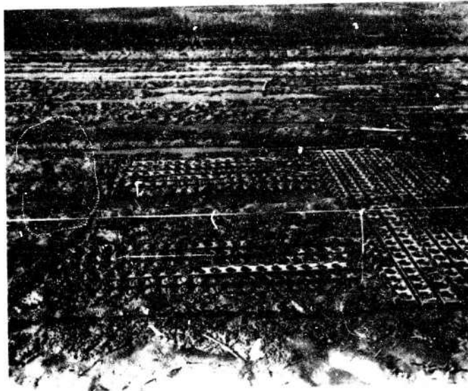
FIG. 13. PIERCED PLANK LANDING MAT PLACED ON LONGITUDINAL PLANK (2 PLANK WIDE) IN THE TRACKWAY.
