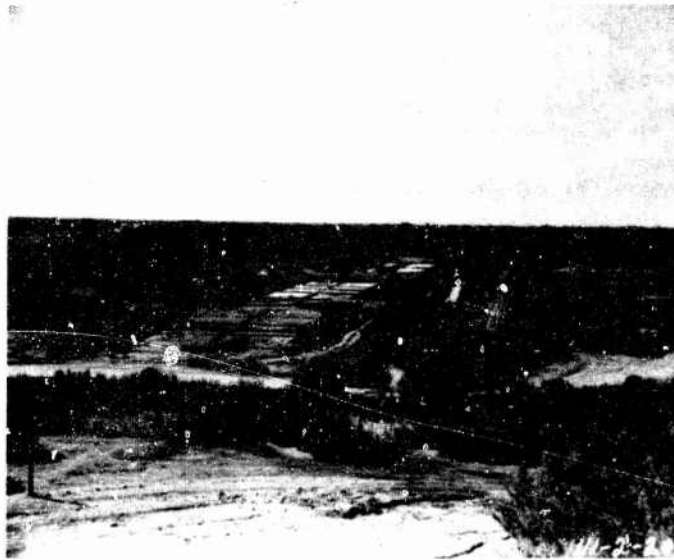
FIG. 1. GENERAL VIEW OF THE TEST AREA CONSTRUCTED TO SIMULATE RICE PADDY FIELDS.
