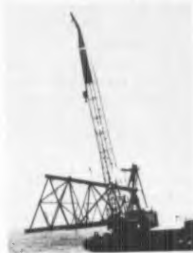
▲ Swinging the jacket around the stern of the derrick barge.
