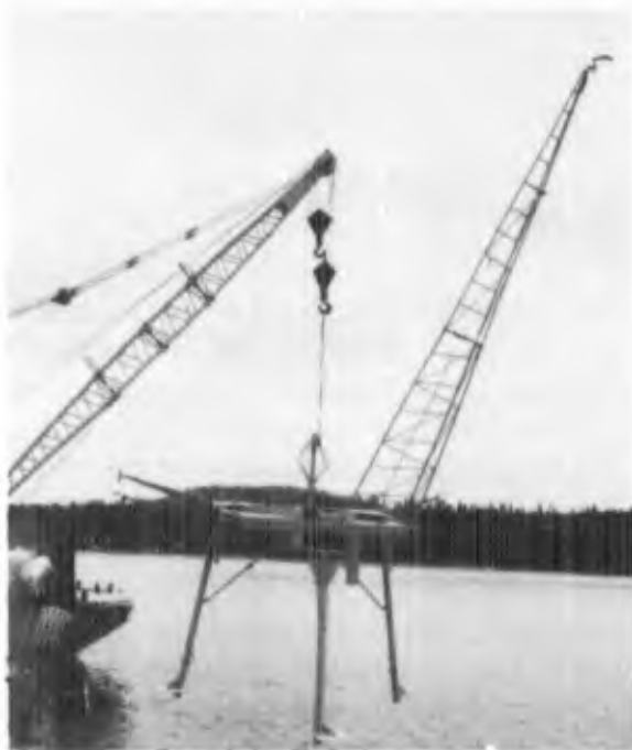
A typical underwater structure, or array, extended to its full length, being overboarded.
