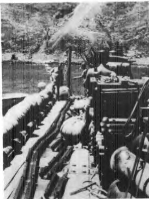
Applying split pipe to cable on the amphibious causeway.
