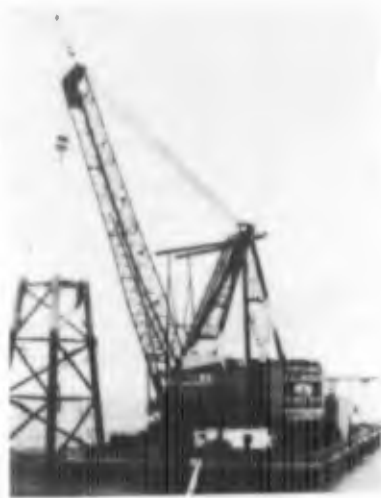
▲ Swinging the jacket around the stern of the derrick barge.
