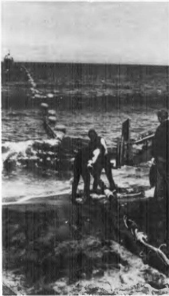
Cable being secured from a cable ship offshore.
