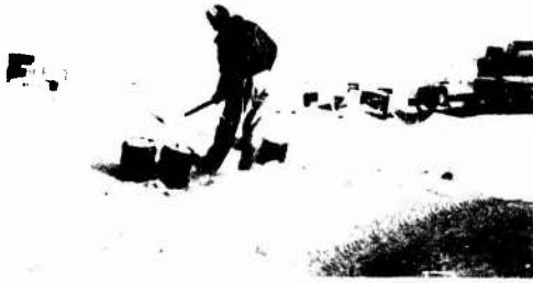
Figure 39. A cook at one of the DEW Line construction camps getting two buckets of snow in order to wash dishes.
