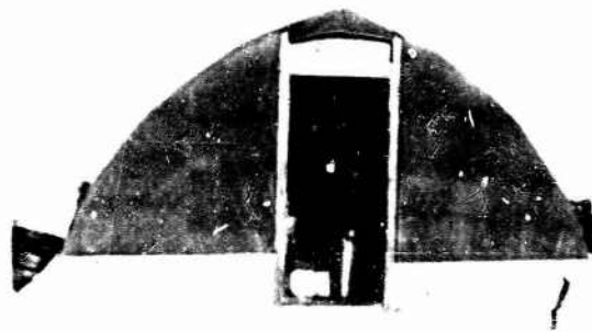
Figure 53. Tent for ice storage showing plastic bag and cardboard container.
