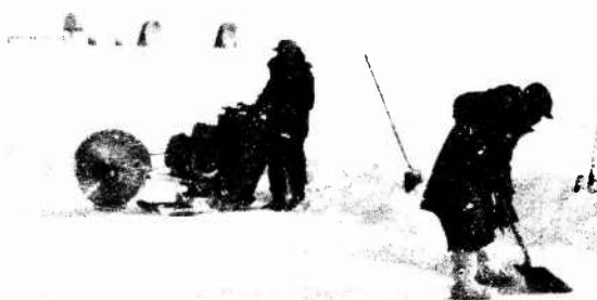
Figure 33. Eskimo laborers sawing lake ice and scraping off the "ice dust."
