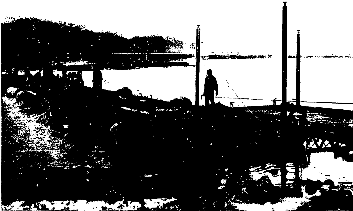
Engineers of Tenth Army build a heavy ponton bridge under fire on Okinawa.
