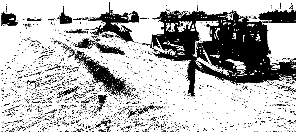
Engineer bulldozers extend a sand causeway from Okinawa beachhead to expedite unloading of LST's.
