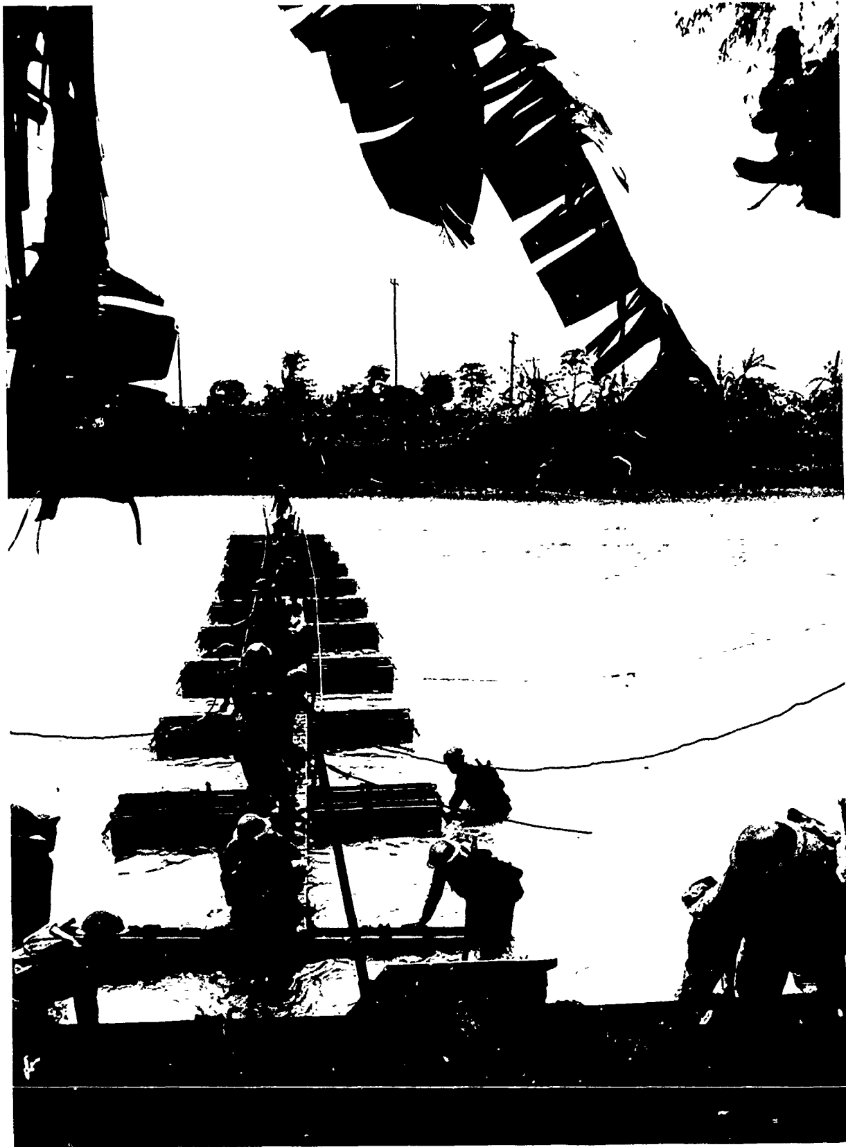
July 1941. Troops of the 14th Engineers, the only trained combat engineer unit in the Philippines at the time of the formation of USAFFE, executing a bridging problem.
