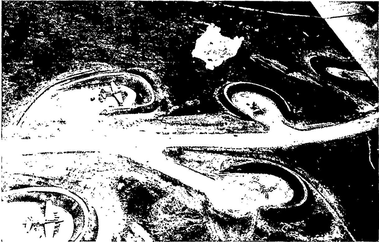
Plane pen construction which required large expenditures of engineer equipment, materials, and manpower.
