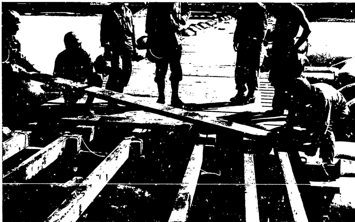
Engineers place chess on a ponton bridge built in Okinawa prior to the assault against Machinto.
