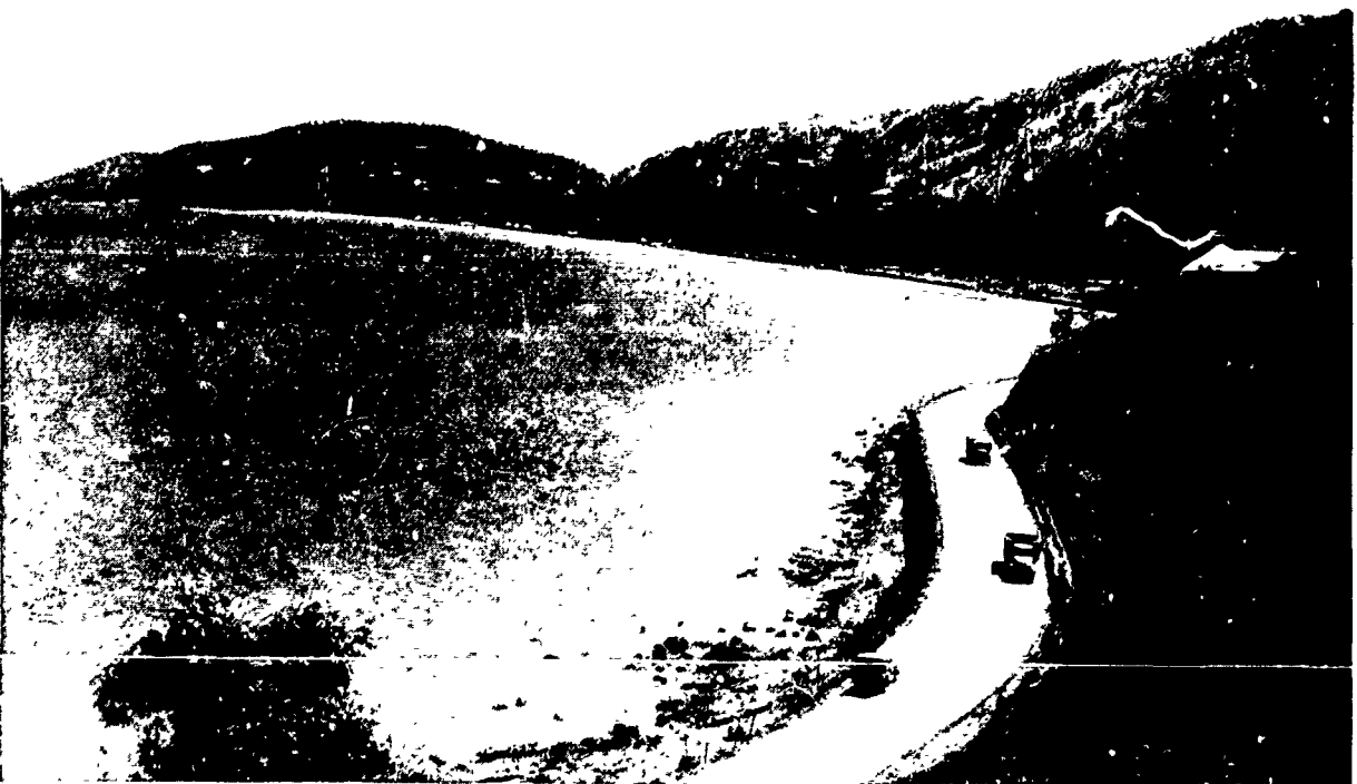
Engineer-constructed road in the Port Moresby area to facilitate expansion of base facilities.
