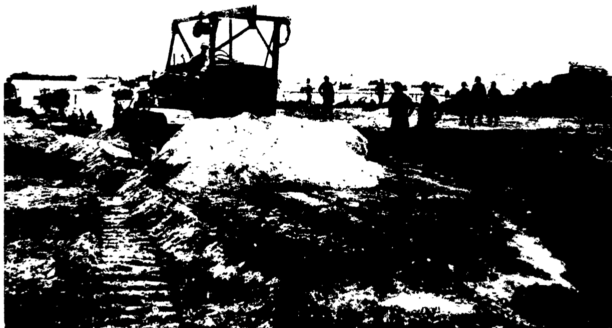
On D Day, Engineers exit from beach to site of Kamiri Drome, Noemfoor Island.
