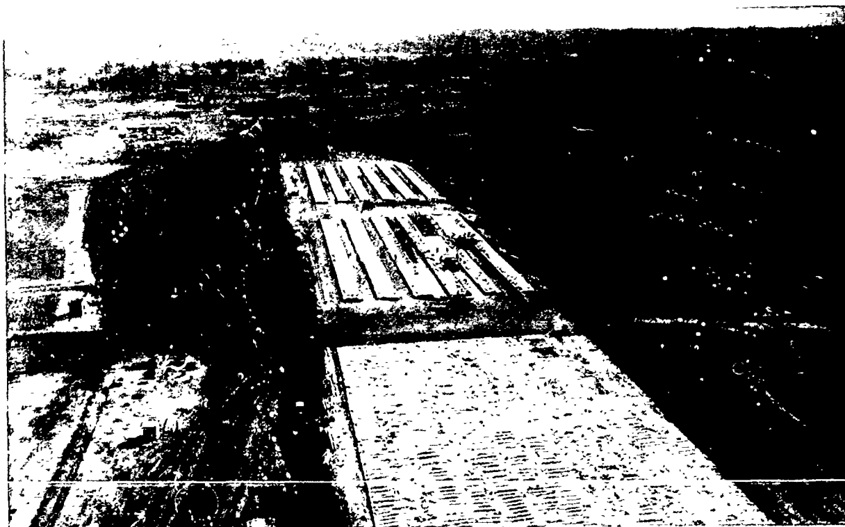
Engineers have just completed this 5,000-foot runway on one of the occupational air bases in Japan, straw has been placed on the still wet concrete to keep it from freezing.
