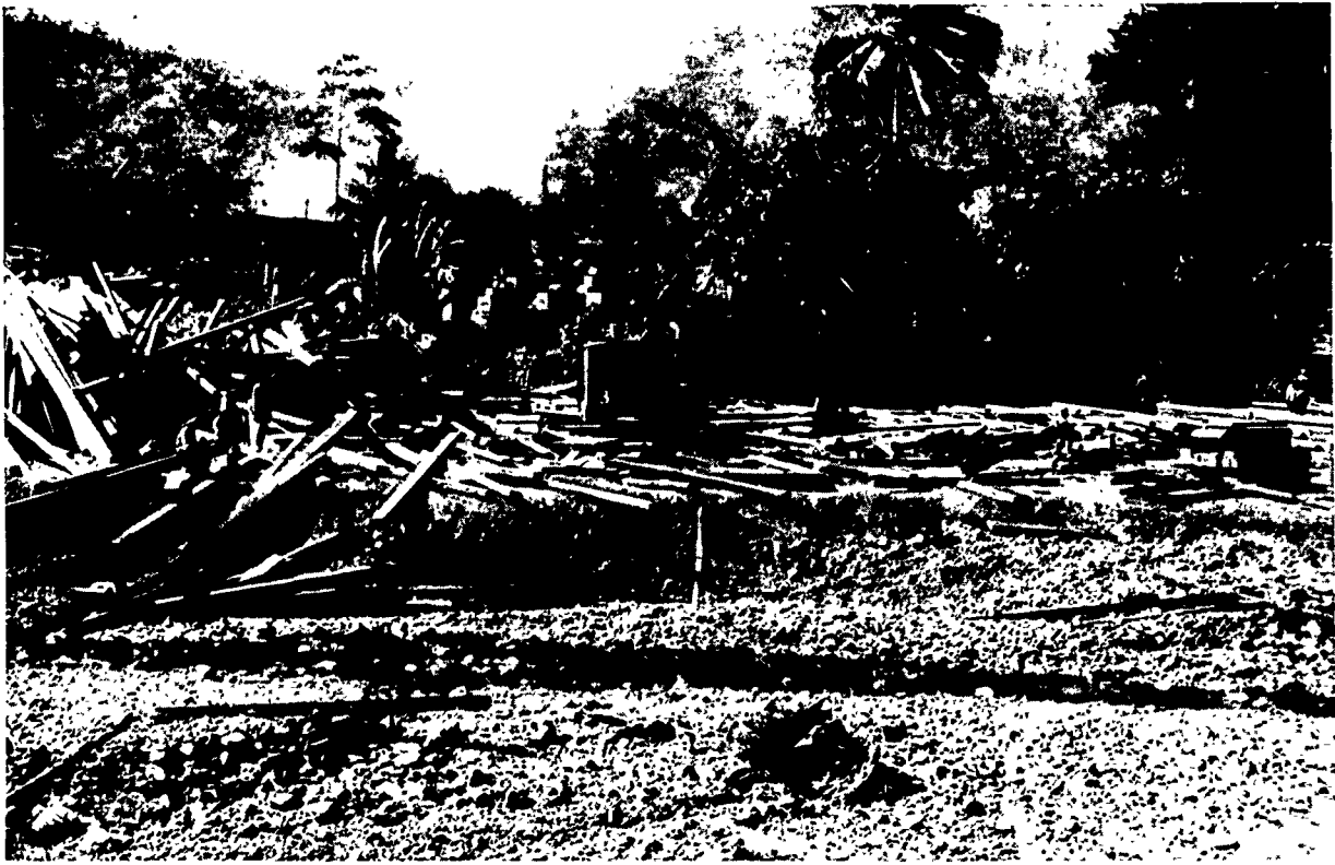
Unsatisfactory condition of lumber stocks, Engineer Depot, Base A, Milne Bay, New Guinea.
