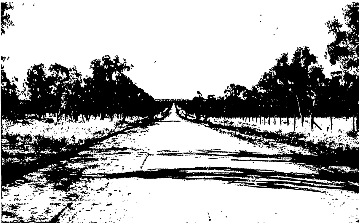
Another section of the Inland Defence Road constructed when the Japanese threatened to cut rail and highway communications along the east coast of Australia.
