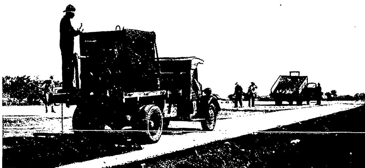
Australian civilians apply bitumen to an airfield runway on the continent.
