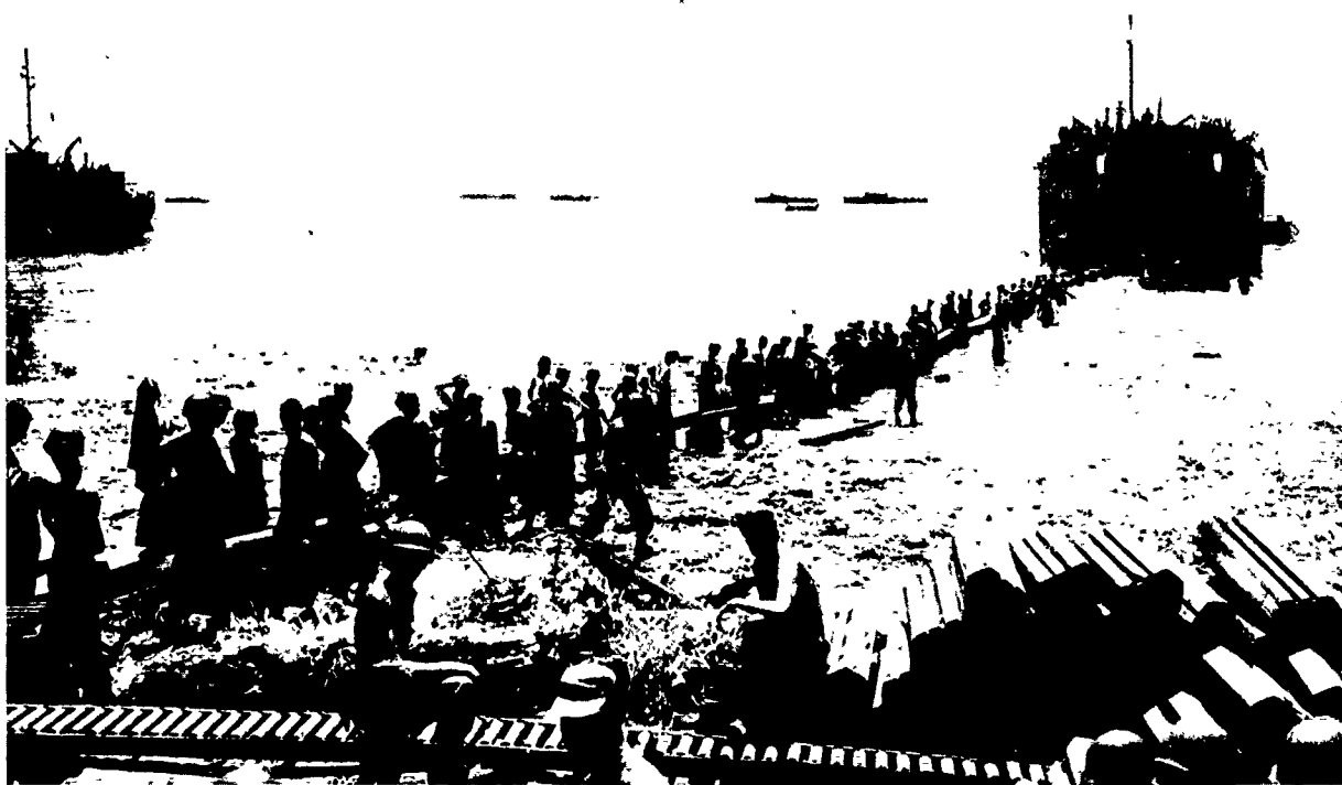
Roller conveyors, operated by an Engineer Shore Battalion, played an important part in easing unloading difficulties at both White and Red Beaches, Morotai Island.
