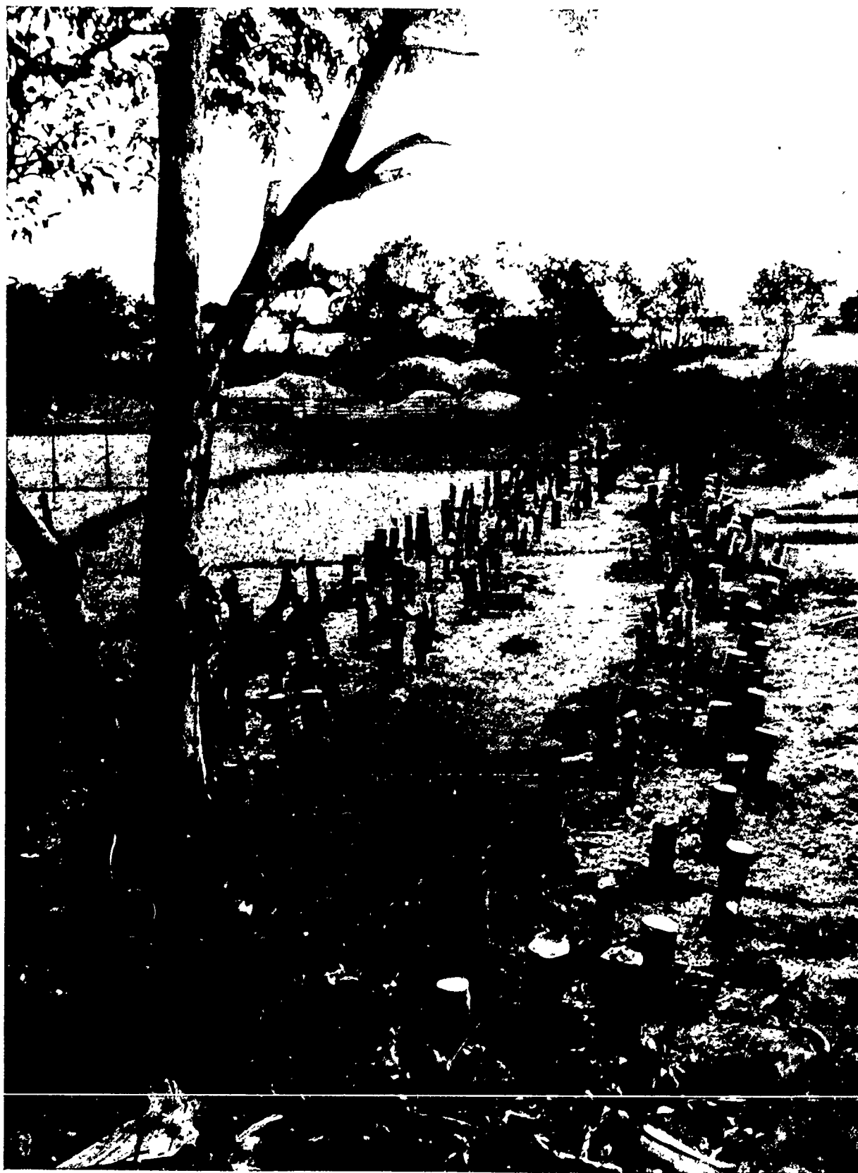
Engineer-constructed tank trap on Bataan. Shortages of engineer equipment, supplies, personnel, and time precluded the preparation of more adequate defenses.
