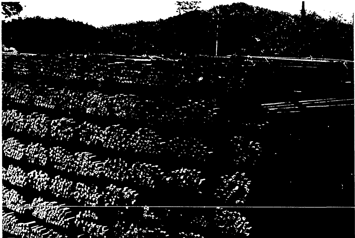
A portion of the same steel stock area after materials have been segregated, rebundled, and restacked by type and length.
