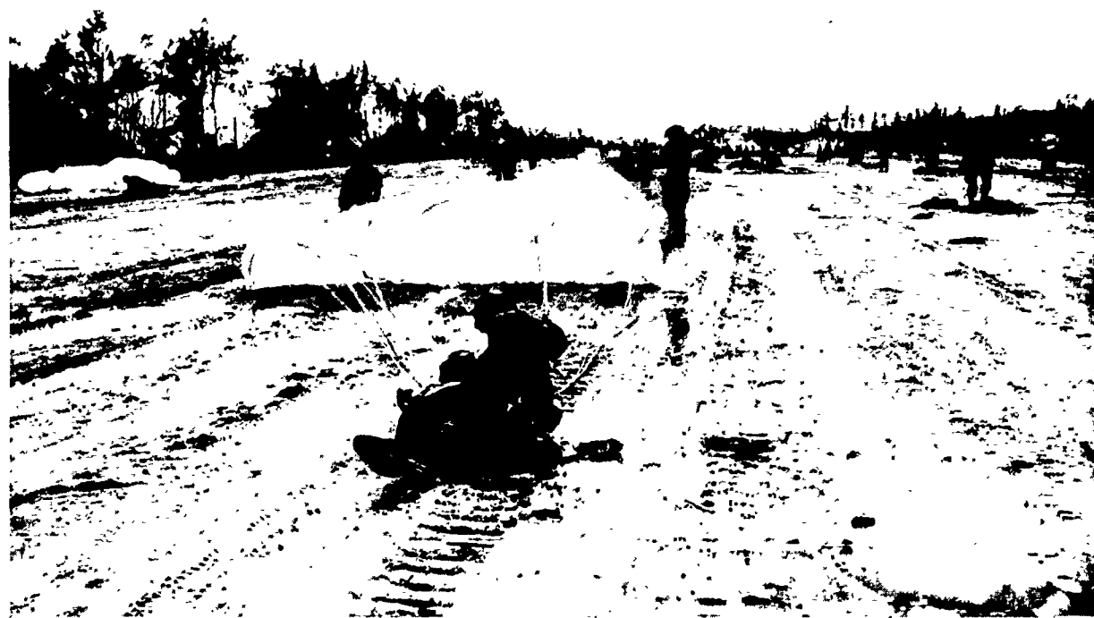
Elements of 503d Infantry (Parachute) land at Kamiri Drome on D plus 1 where Japanese-constructed runway is being improved and extended.
