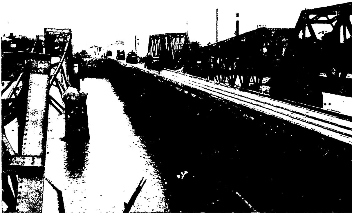
Effectiveness of 1941 engineer demolition of two Calumpit bridges is verified by photograph taken in 1945 after liberation of Luzon. Japanese occupation forces never attempted repairs. The bridge in use was constructed by U. S. Engineers in 1945.
