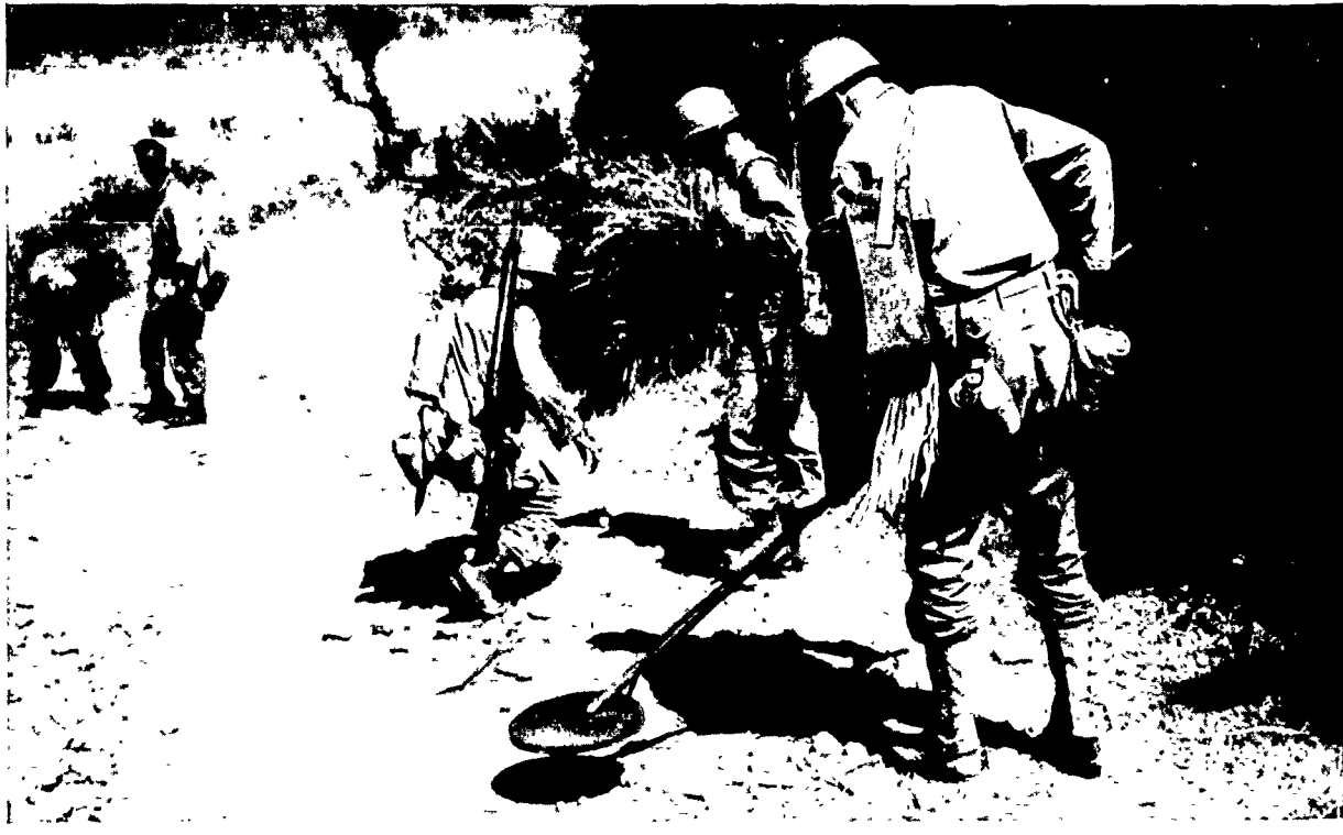
Engineer squad using mine detectors to locate the many mines planted along the Luzon roads by the retreating Japanese.
