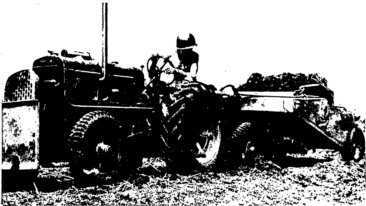
Engineer airborne equipment that reached Nadzab, New Guinea, by air transport for airfield construction.
