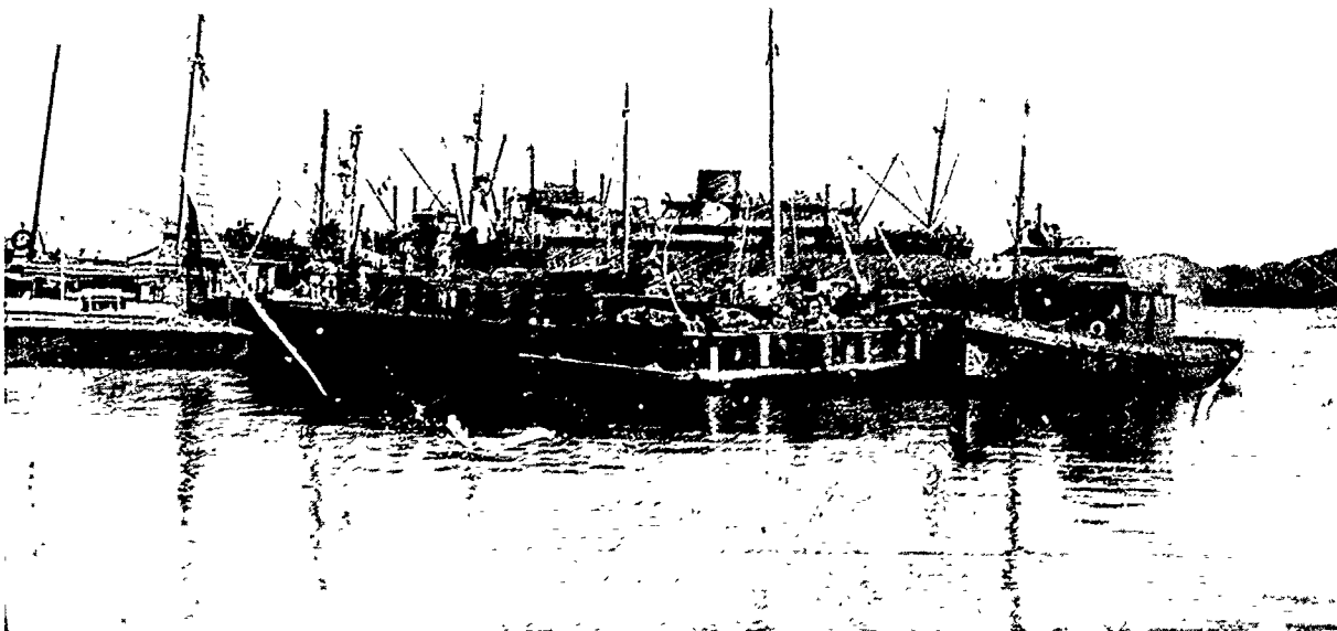
Unloading problems in 1942 at U. S. Advanced Base, Port Moresby, New Guinea, requiring handling supplies from ship to barge to shore.
