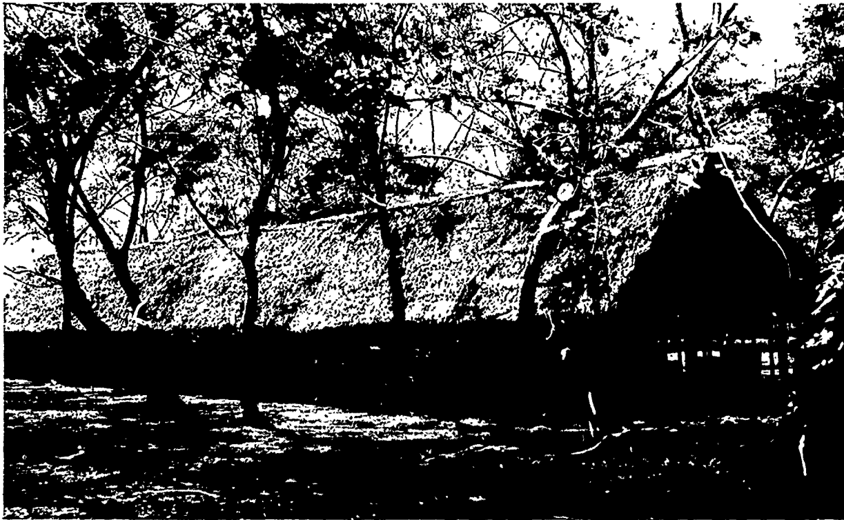
Native-style headquarters structure established through maximum use of local supplies and a minimum expenditure of troop labor.
