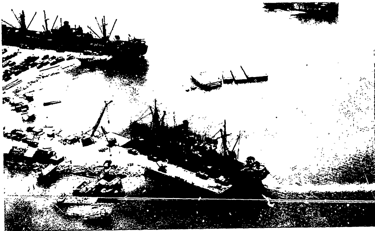
Unloading piers at Tatana Island constructed by U. S. Army Engineers.
