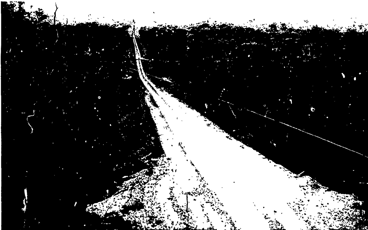
Elevated section of the Inland Defence Road sweeping through thickly wooded, unimproved country between Duaringa and Charters Towers, Australia.
