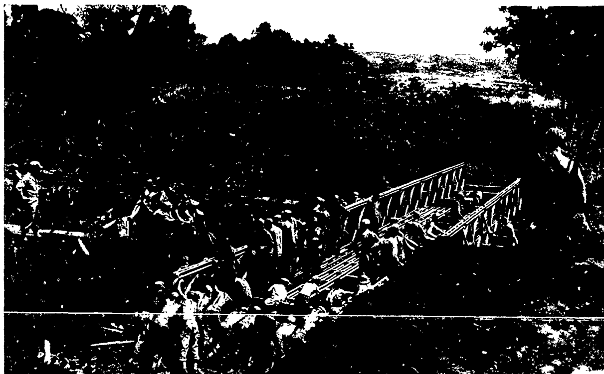
Engineers launch a Bailey bridge over a stream near Valencia, Mindanao.
