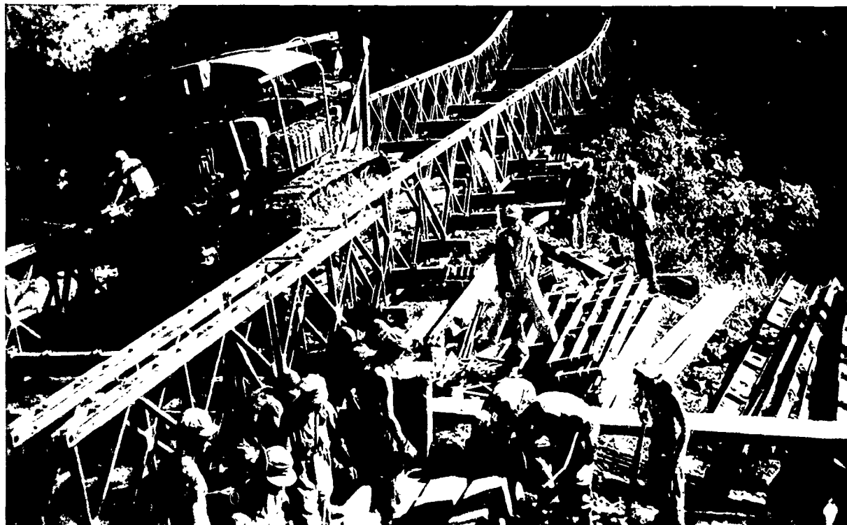
Engineers have removed the blade and are using this bulldozer as a counterbalance in launching a Bailey bridge along the Sayre Highway, Mindanao.
