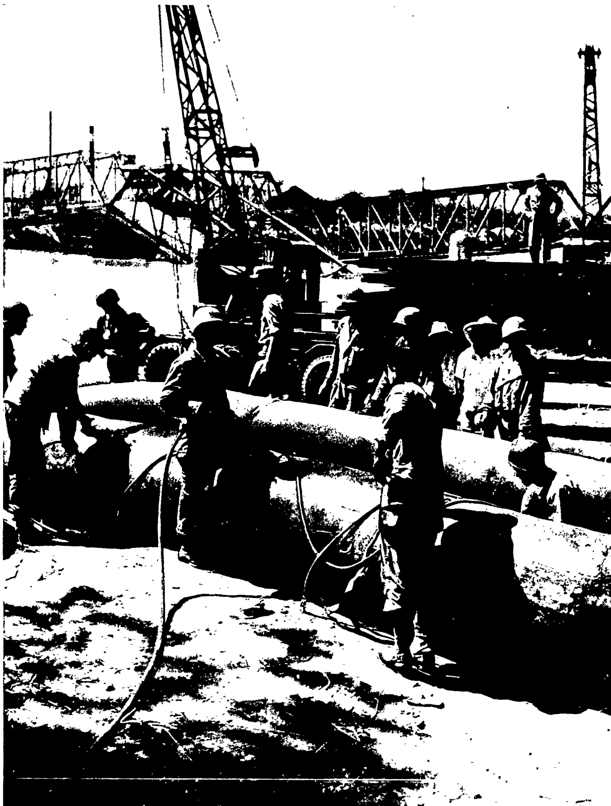
Engineers assembling pontoons to be used in bridging the Pampanga River during the operations on Luzon.
