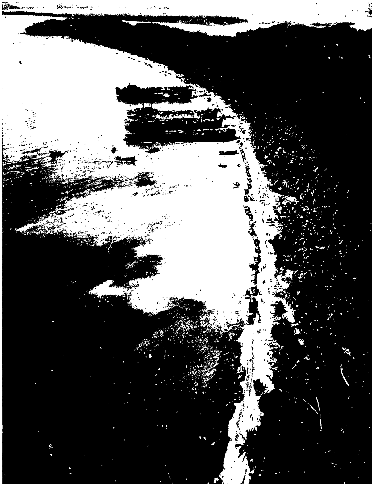
White Beach No. 2, Humboldt Bay, Hollandia, Netherlands New Guinea—Satisfactory landings by LST's and limited dispersal areas ashore.
