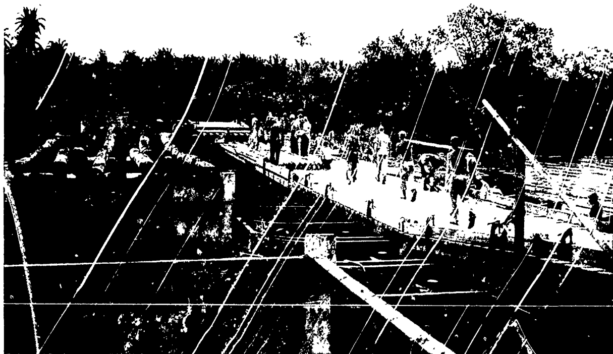
Ponton bridge at Pajo, Leyte, maintains the advance to the north-east.
