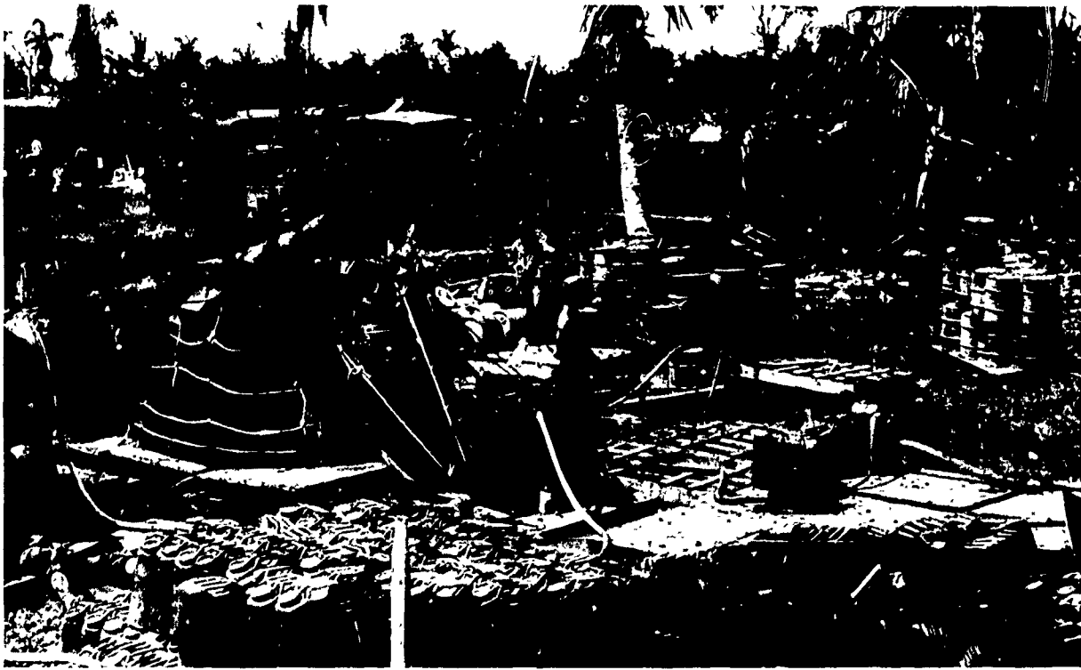
Engineer water purification unit and portable canvas reservoir are in operation on Leyte early on D plus 1.
