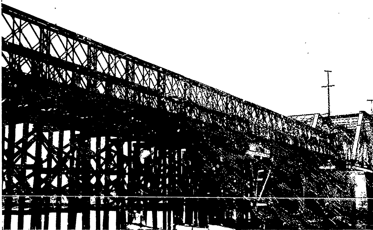
Photograph shows the timbe. piling and part of the Bailey bridge construction in the Pampana River bridge at Calumpit, Luzon.
