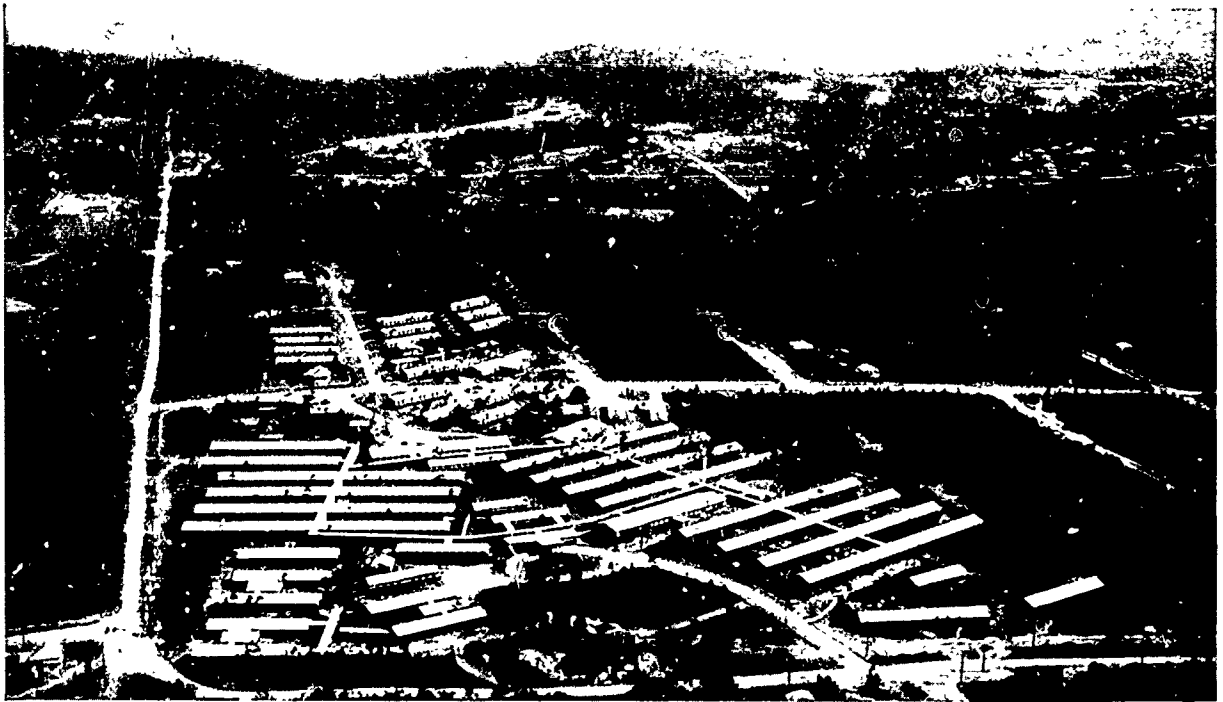
View of Ekibin Hospital, typical example of Engineer construction work in Base Section 3, Australia.
