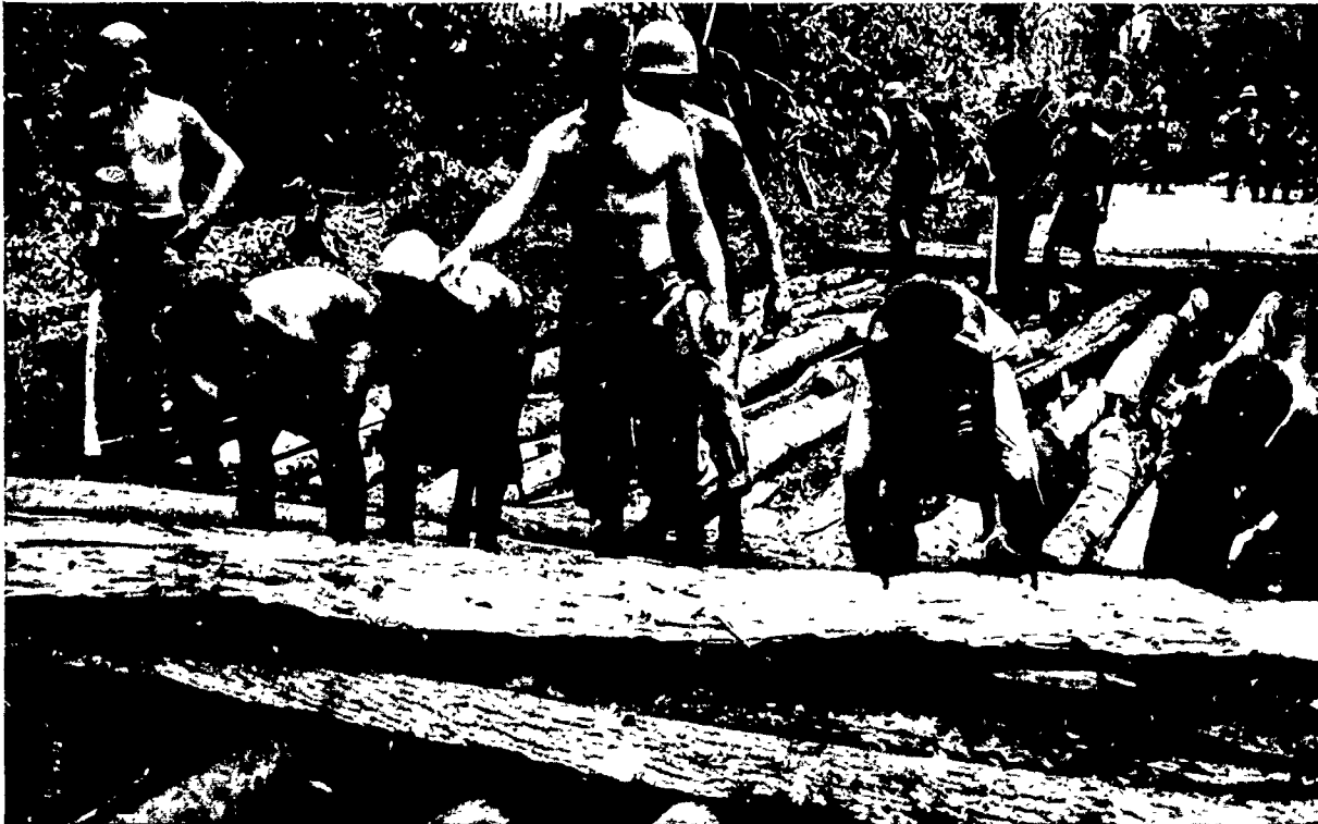
Recruited native labor assisting engineer construction of corduroy road through dense jungles of New Guinea.
