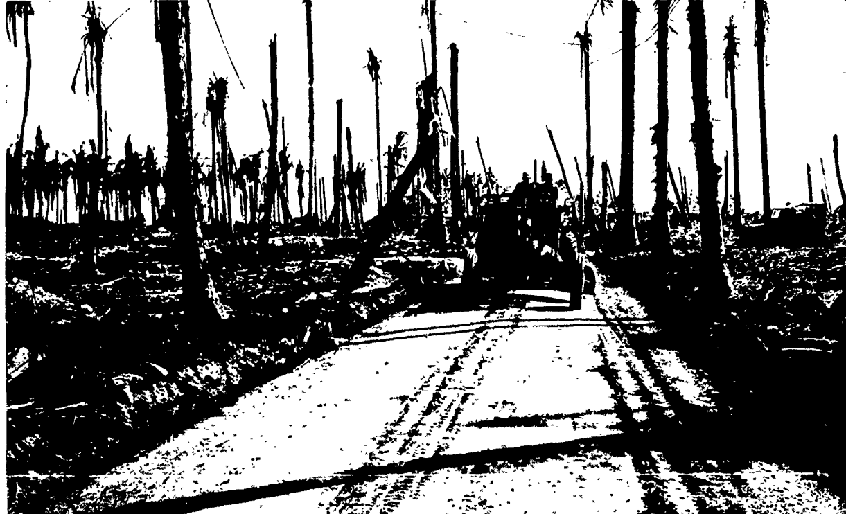
Engineer Shore Party typical white coral road construction on Wakde. Note communication wire strung along shattered tree trunks for protection from wheeled and tracked vehicles.
