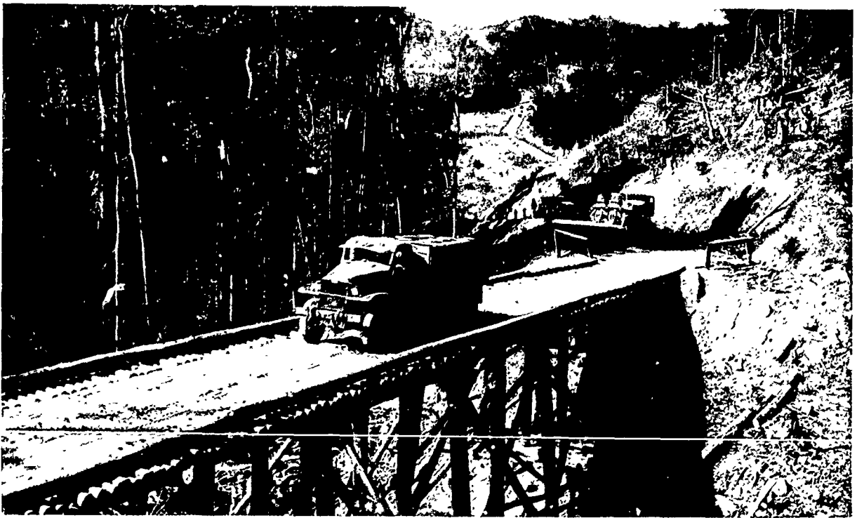
Supply convoy crosses a timber bridge along the newly constructed Oro Bay-Dobodura Road in New Guinea.
