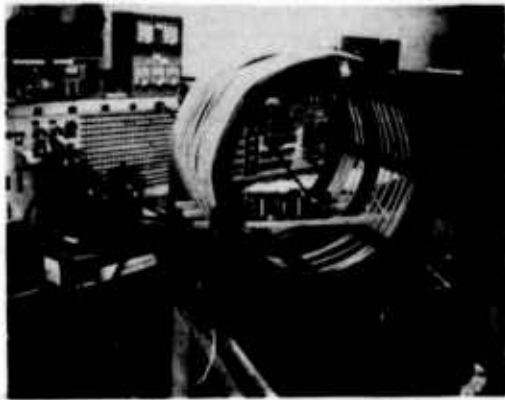
Figure 27a. P13-20 Autopilot Control Panel (in Coil). Servos on Test Bench at Left. Computer in Rack at Right of Coil
