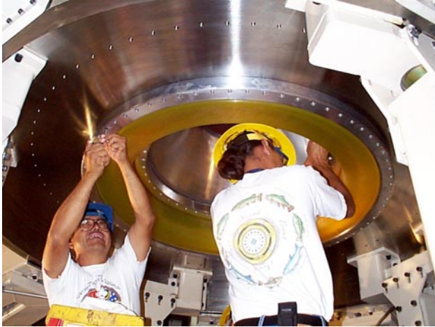
Figure 8 Bottom insulator installation
