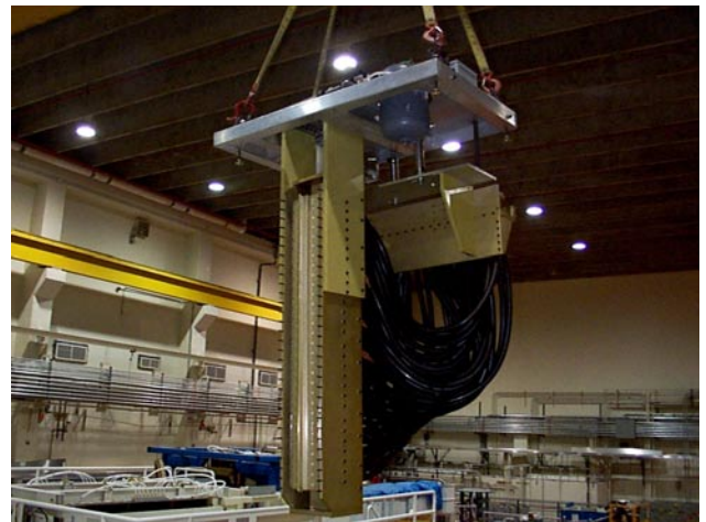
Figure 3 Cable header and load protection switch assembly
