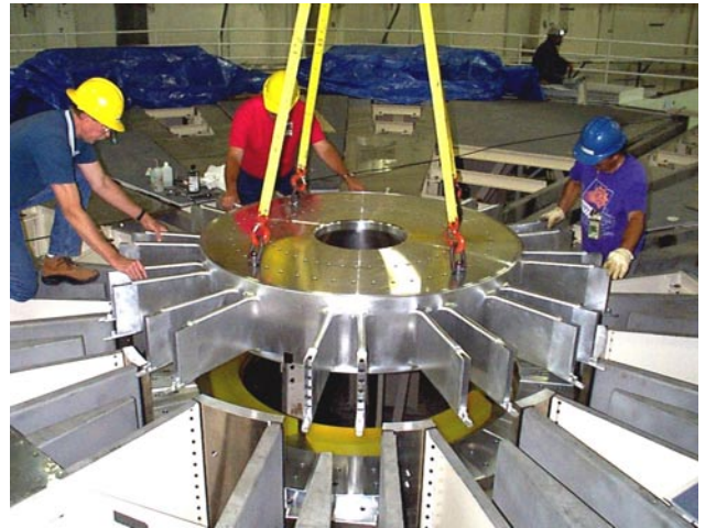
Figure 6 Transition high-voltage conductor installation
