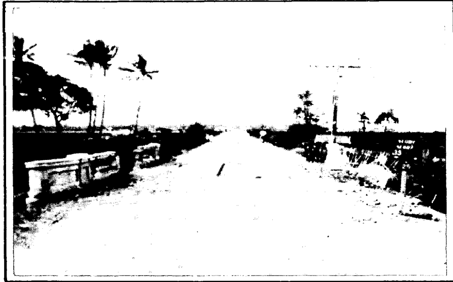
In some places on NEGROS partially demolished bridges could be repaired...
