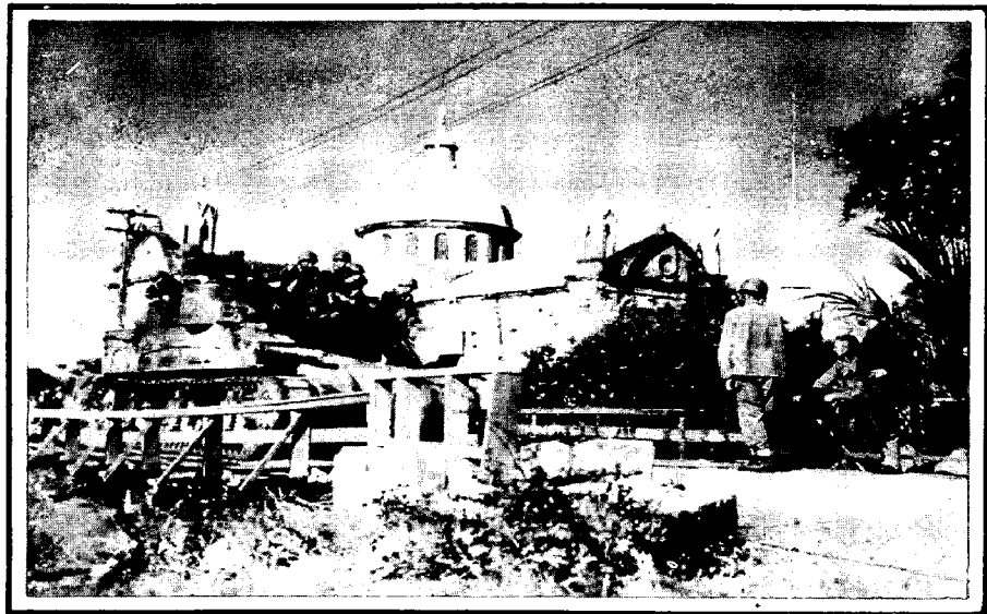
One of our self propelled 105mm howitzer (M-7) rumbles across a narrow wooden bridge on PANAY.
