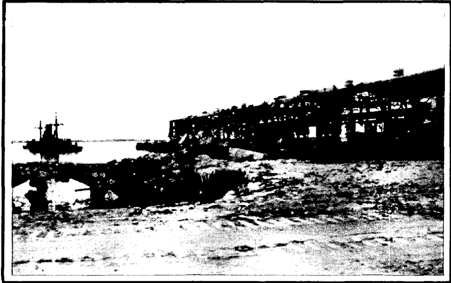
North side of damaged Pier No. 2 at CEBU CITY, showing sunken Japanese vessel.
