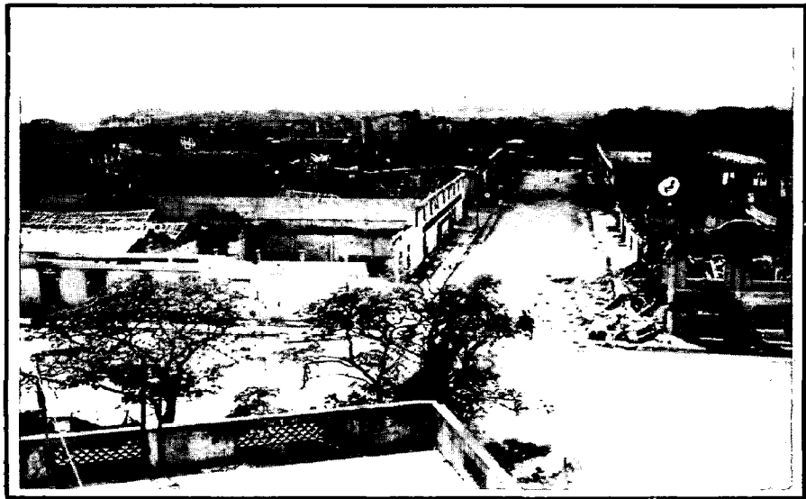
The destruction wrought throughout CEBU CITY by American bombings and Japanese demolitions is shown graphically in this view of the downtown section.
