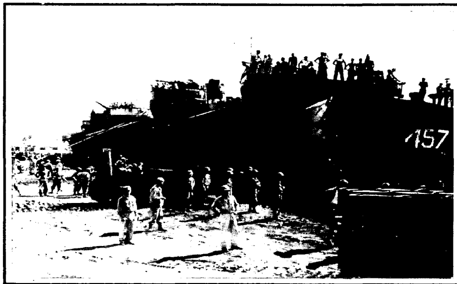
Landing Ships, (Tank) nose up to ramps built with concrete rubble which was available in great quantity in demolished CEBU CITY.
