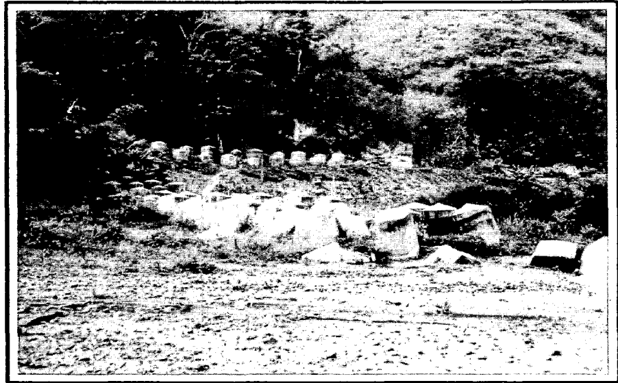
A "dragon's teeth" tank block constructed by the Japanese on CEBU. The concrete blocks are three feet high.
