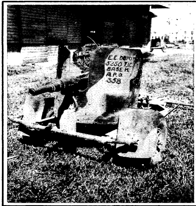
A dual-purpose Japanese anti-tank gun with base improvised from a truck axle and airplane wheels.
