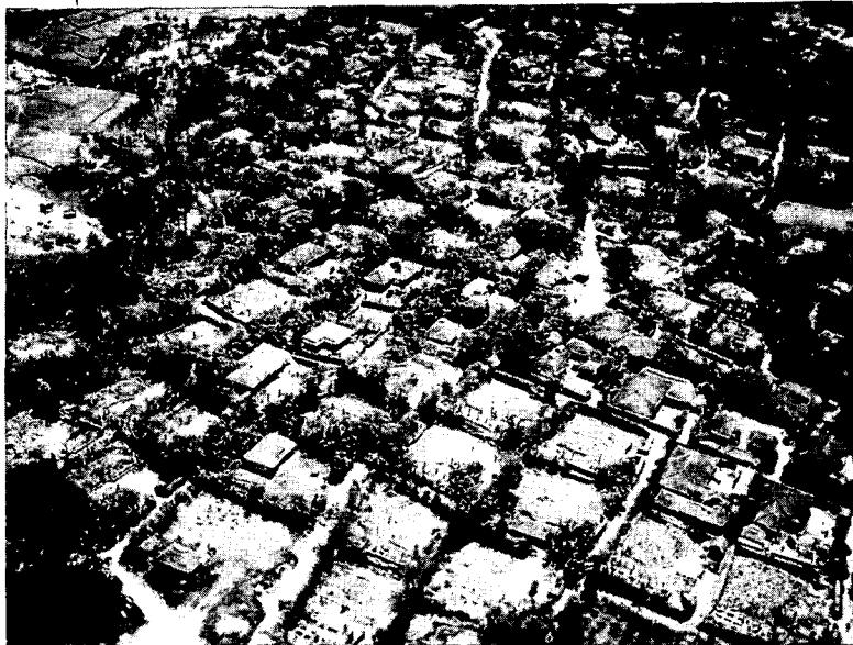
Two aerial obliques of the town of Hanza, near Yontan Airfield. Hanza is a typical Okinawan town. Scarcely more than a village, it is in reality a collection of small farms and stores. Houses are of wood construction with each house surrounded by a wall fringed with shrubbery.
