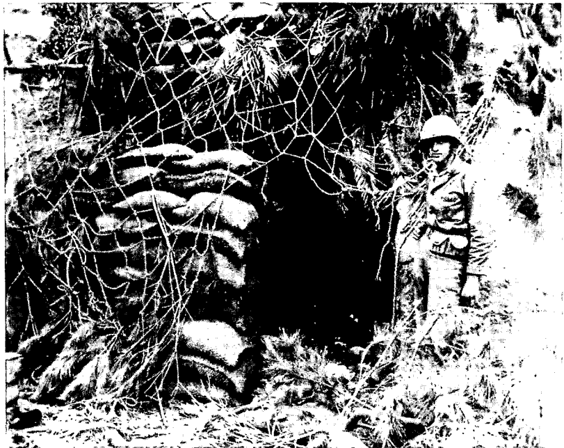
Sand-bagged and revetted personnel dugouts.
