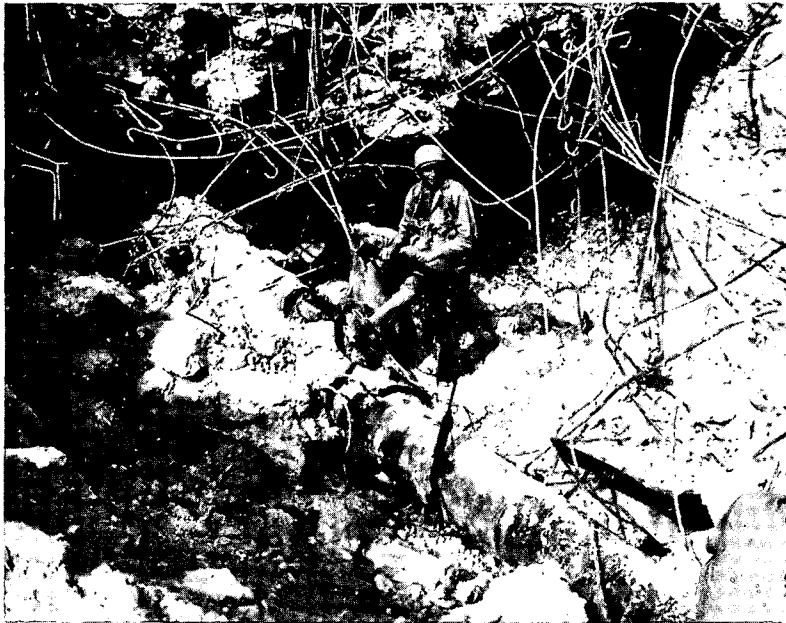
120mm coastal defense gun completely demol- ished by a direct hit.
