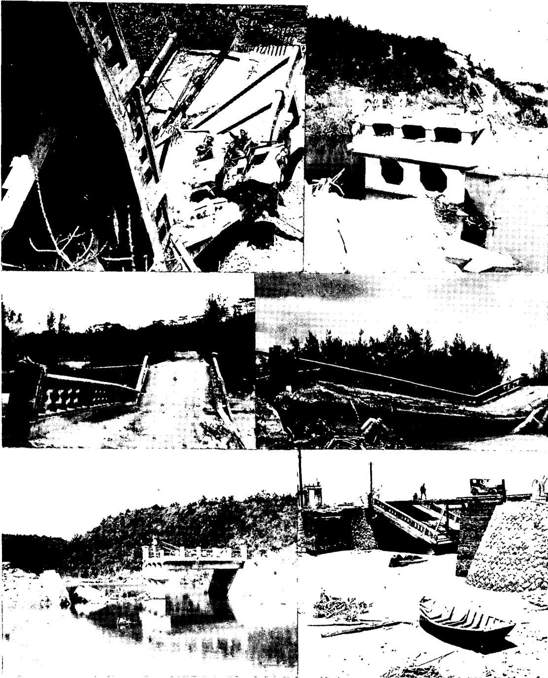
Above are five typical Okinawan bridges demolished by the enemy to impede the Sixth Marine Division advance. The success or failure of their demolitions will be immediately evident.
