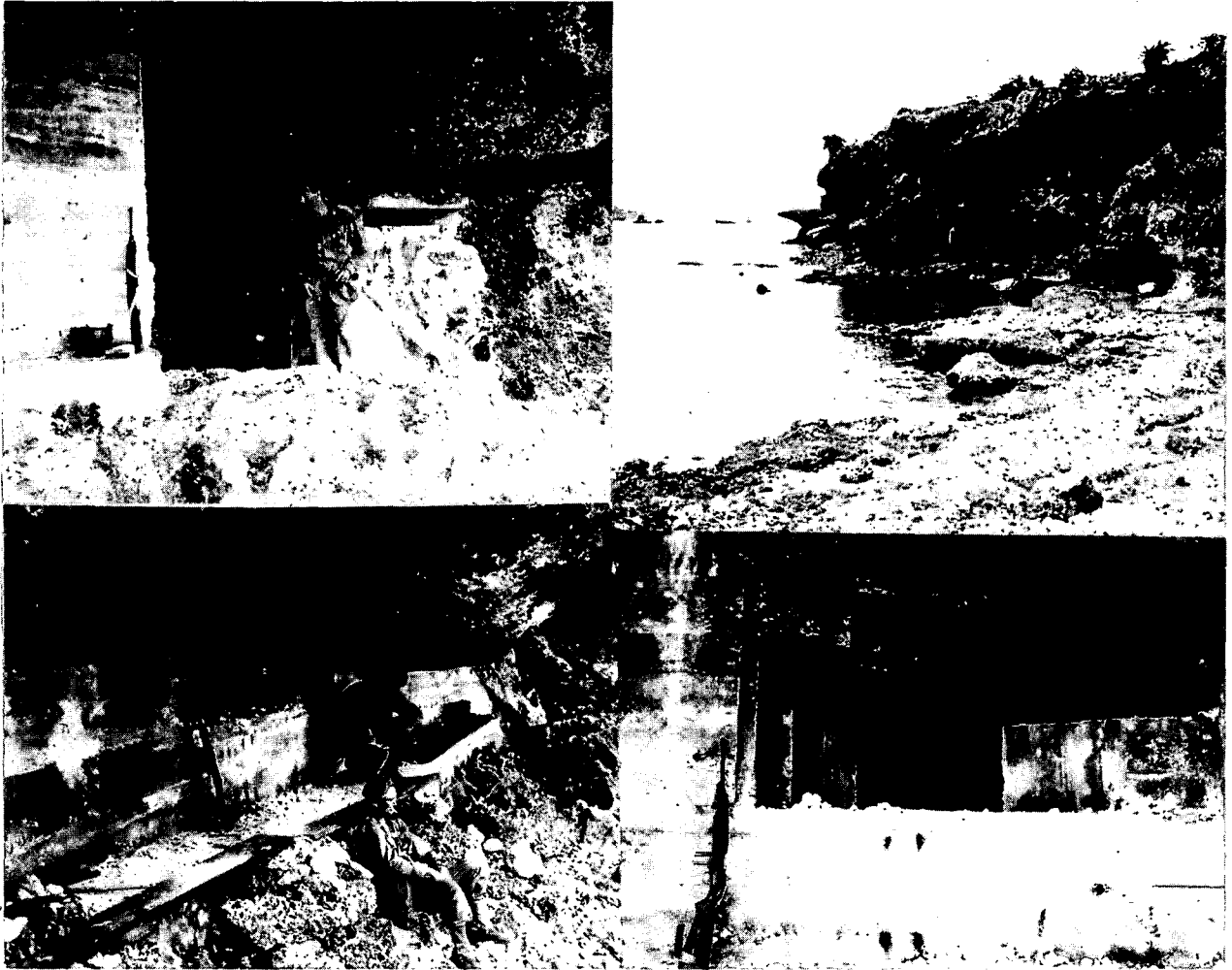
(Upper Left) Main entrance and small machine-gun port. (Upper Right) Coral cliff extending seaward in which the strongpoint was constructed. (Lower Left) View of the anti-boat gun port showing the overhanging cliff. (Lower Right) The anti-boat gun port - constructed of concrete and affording the maximum in observation and protection for the gunners.
