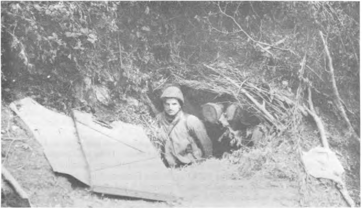
GERMAN SHELTER near Villiers-Fossard with heavy log roof for added protection. The enemy had had time to prepare such defenses in considerable depth along the whole front facing the XIX Corps.
