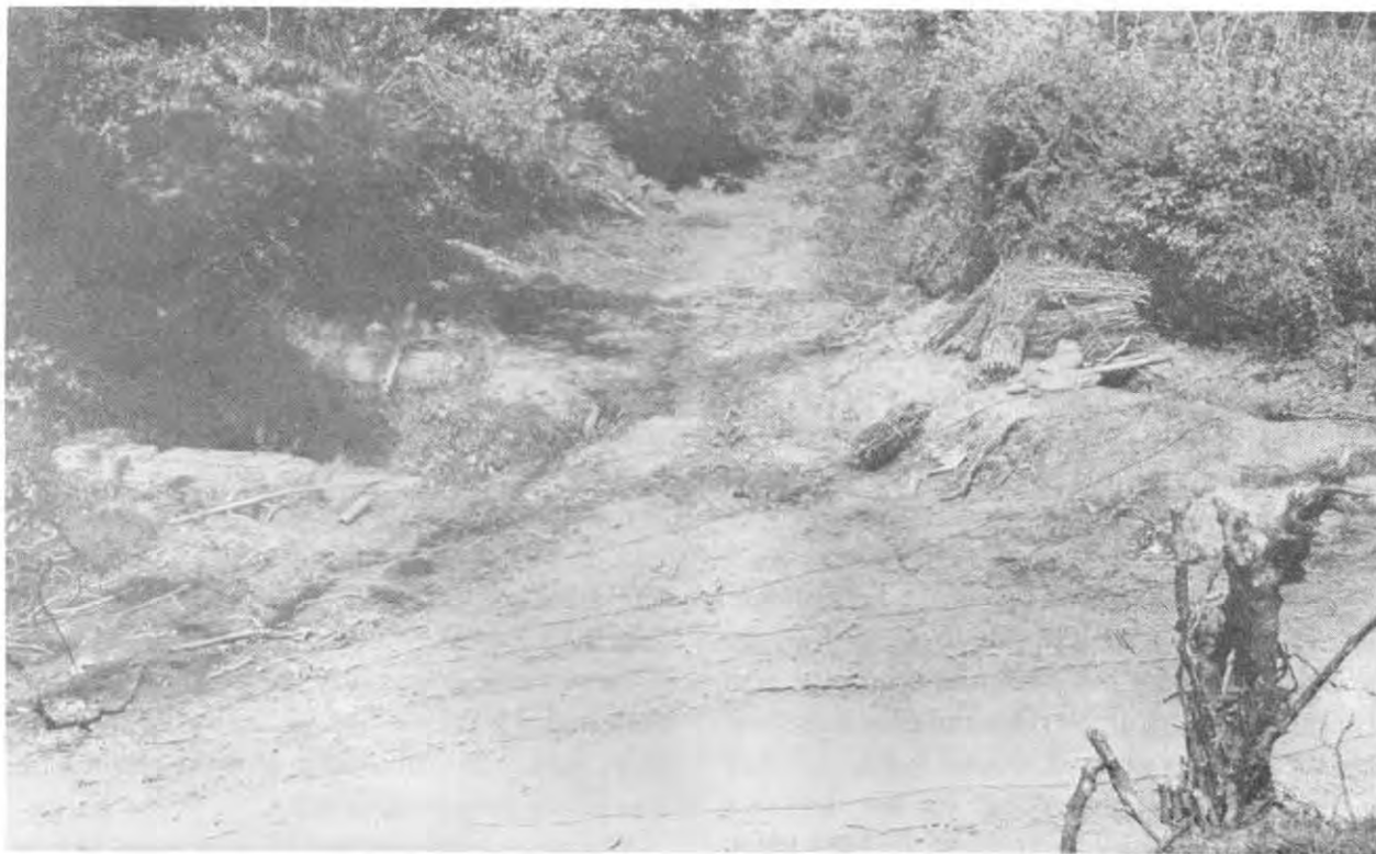
A DEFENDED LANE near Martinville village, with shelter holes on both sides, covered in places by bundles of brush against shell bursts.
