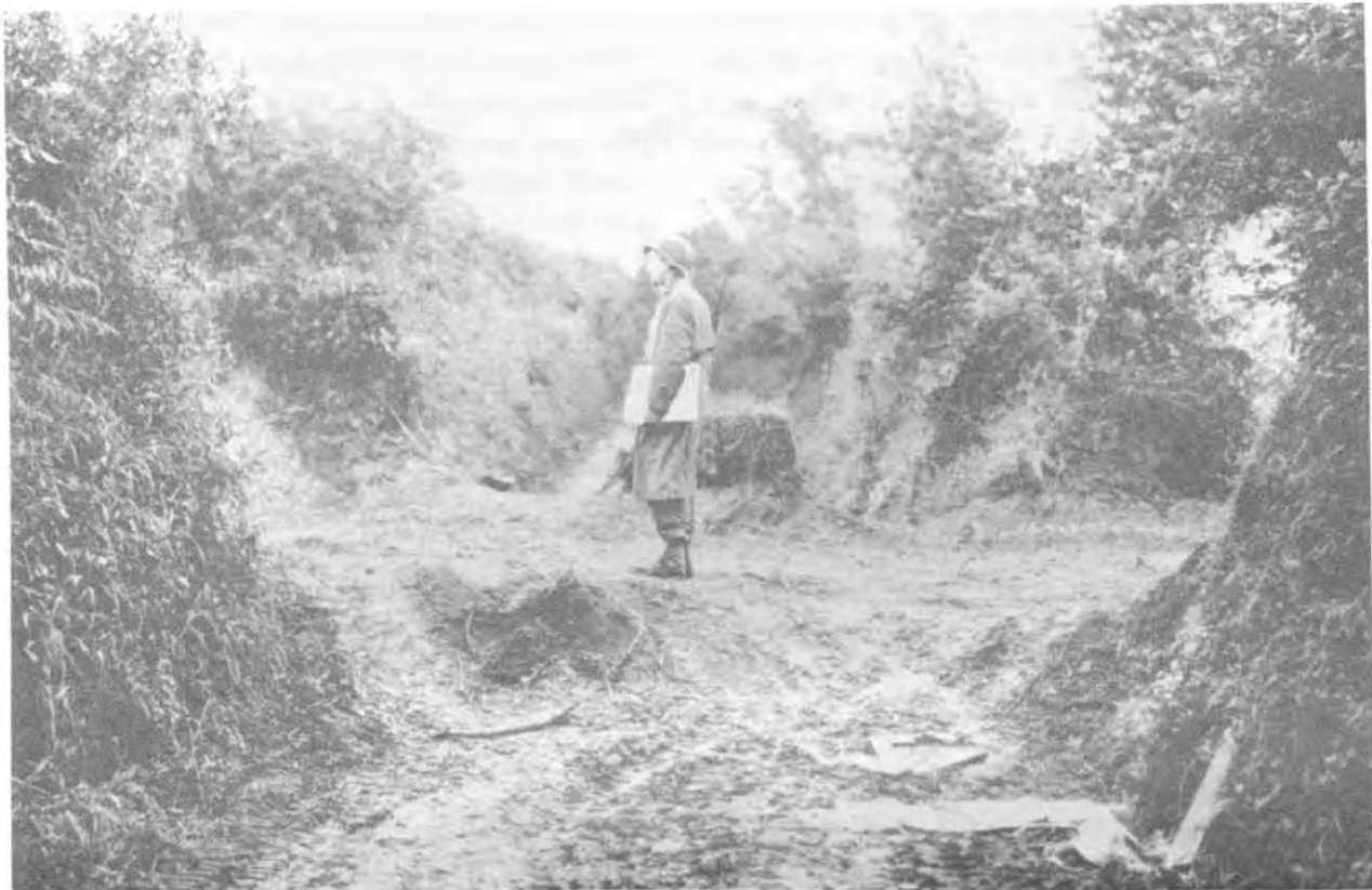
FIELD INTERSECTION, near Villiers-Fossard, giving some idea of the scale of embankments. Beyond the soldier is a narrow lane, flanked by hedgerows. Bulldozers have cut a trail through the field corners in the direction toward which the man is looking.
