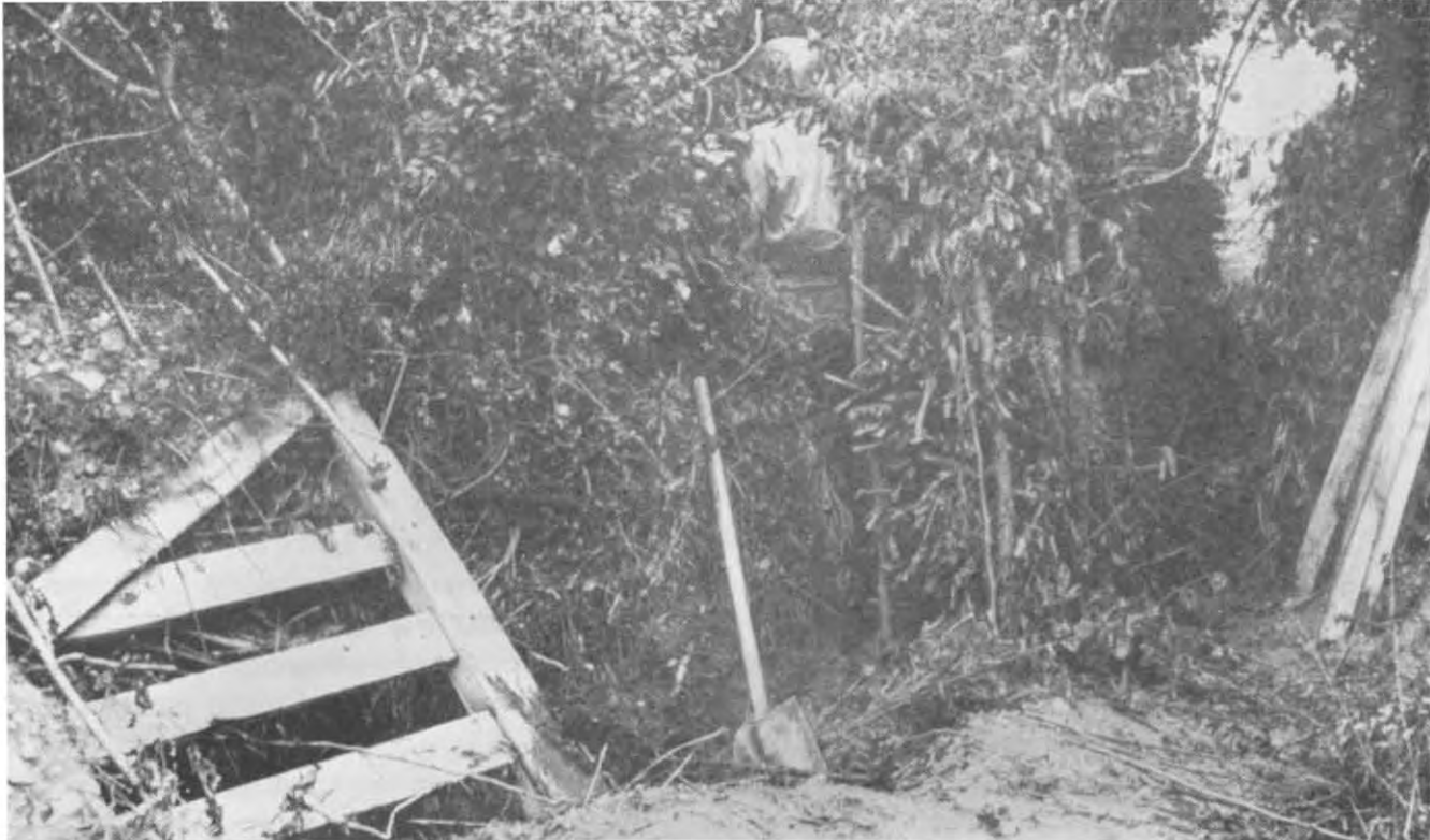
HEDGEROW DEFENSES in the salient near le Carillon. Here is a typical combination: at lower left, a dugout shelter for several men; center, a firing position for machine gun; right, gap for communication into next field, where rifle pits are cut in the bank.
