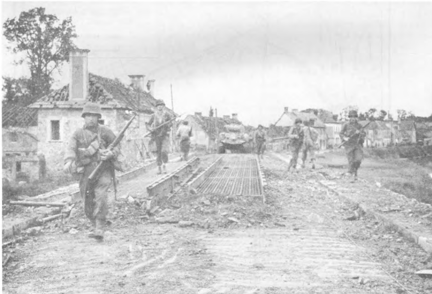
BRIDGE AT ST-FROMOND over the Vire River is being used on 8 July by elements of the 3d Armored Division. The Germans failed to destroy this bridge, repaired here with treadway.
