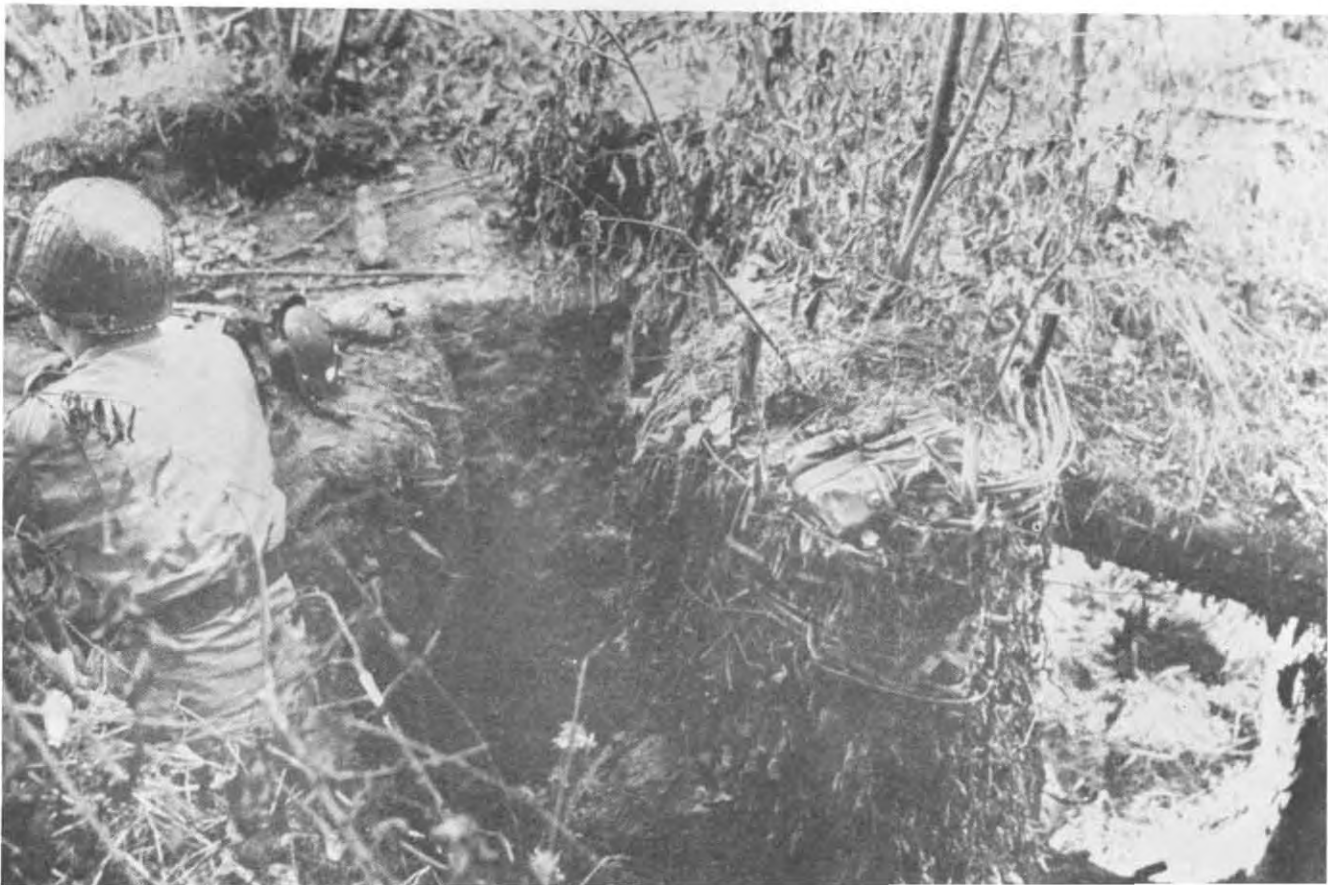
GERMAN MACHINE-GUN POSITION near le Carillon. At the right is the entrance to the shelter for use during artillery fire.
