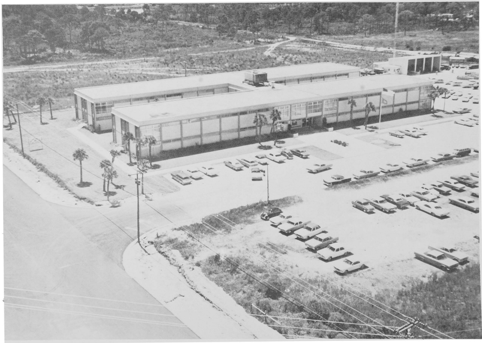
New Canaveral District, Corps of Engineers, occupied this busy Headquarters, constructed under a lease-build arrangement on Merritt Island, south of NASA's Kennedy Space Center operations.
