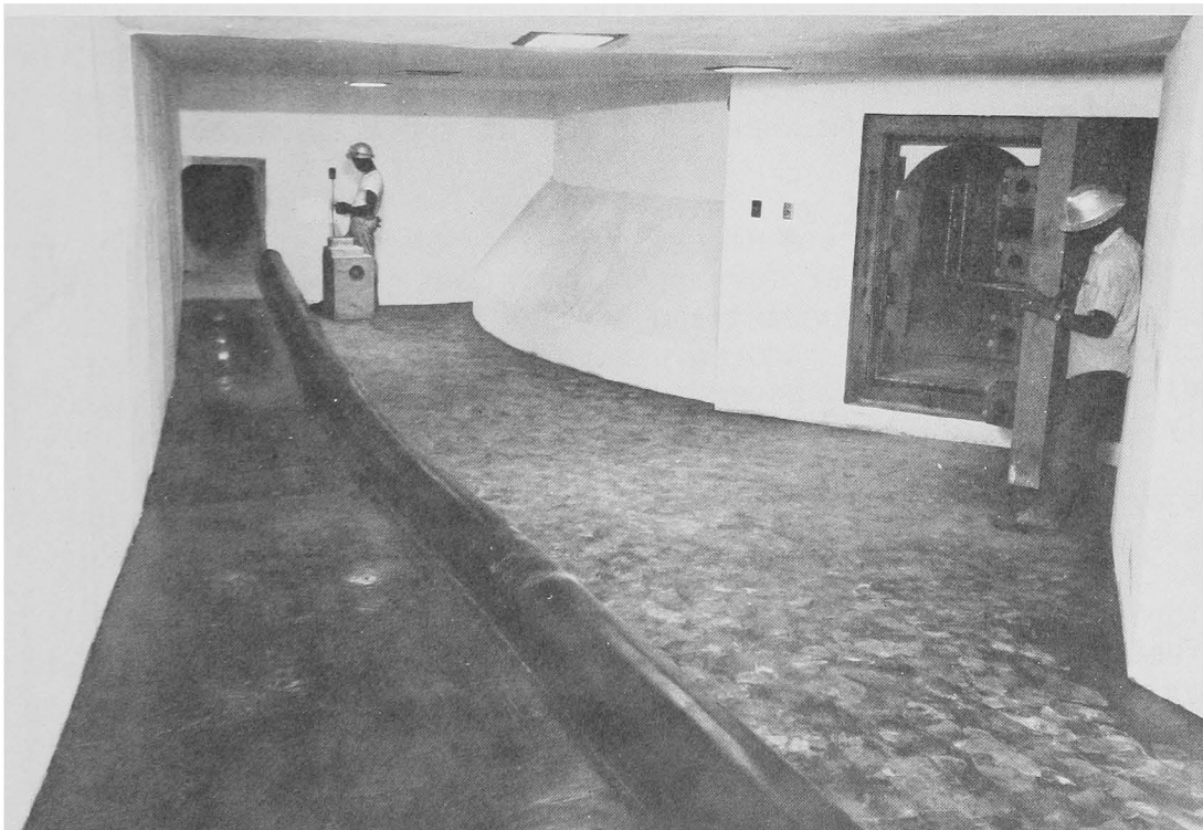
Bottom of egress chute in termination room and door to blast resistant room.
