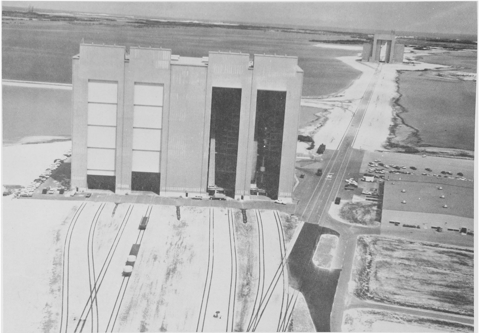
Dual-track railroad terminates at each assembly bay of Titan's Vertical Integrated Building, to give it multiple assembly and movement capability. Dual-track rails then move easily through center bay of Solid Motor Assembly Building. Concept also embodies two launch pads farther east. Eight-hour reaction time was military objective.
