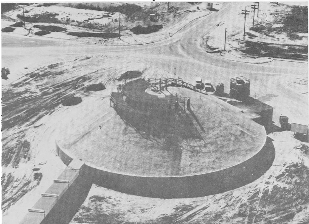
Blockhouse, Complex 34 - Saturn I CCMTA, Patrick AFB, Florida
