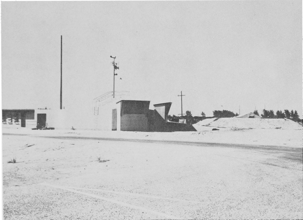
First blockhouse (above) with two launch rooms facing Pads 1 & 2, is contrasted to a typical dome-shaped structure which later became standard blockhouse configuration. (below)
