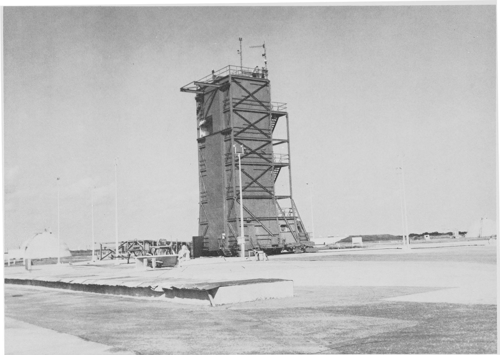
Minuteman Service Tower was the first fully enclosed structure of its kind built by Corps at Cape. Others were of steel-framework open Gantry type. Note beehive blockhouses at left and right of photo. Corps built two silos, two flat surface pads for MINUTEMAN.
