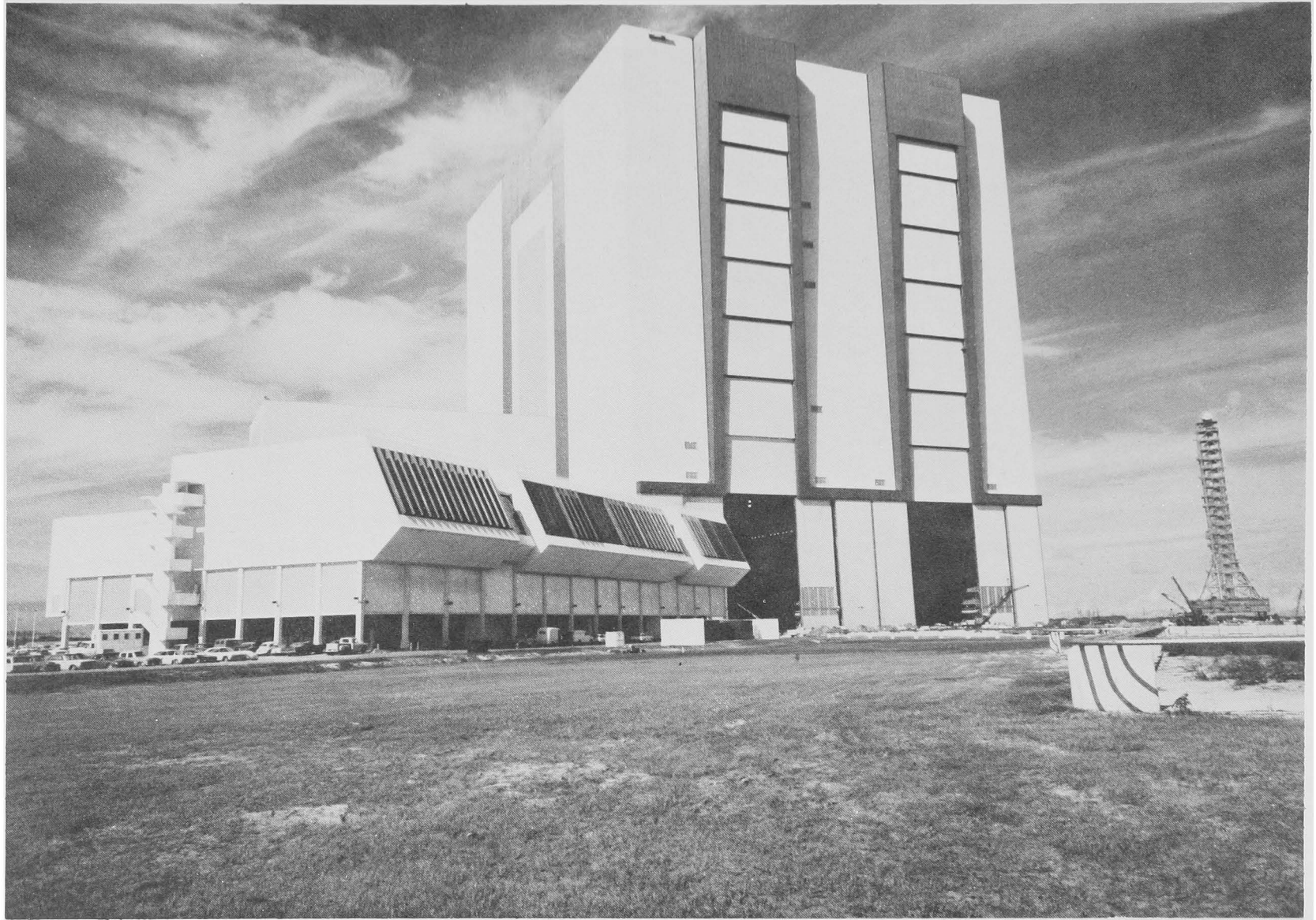
Launch Control Center (left foreground) showing window louvers. Vehicle Assembly Building in background.
