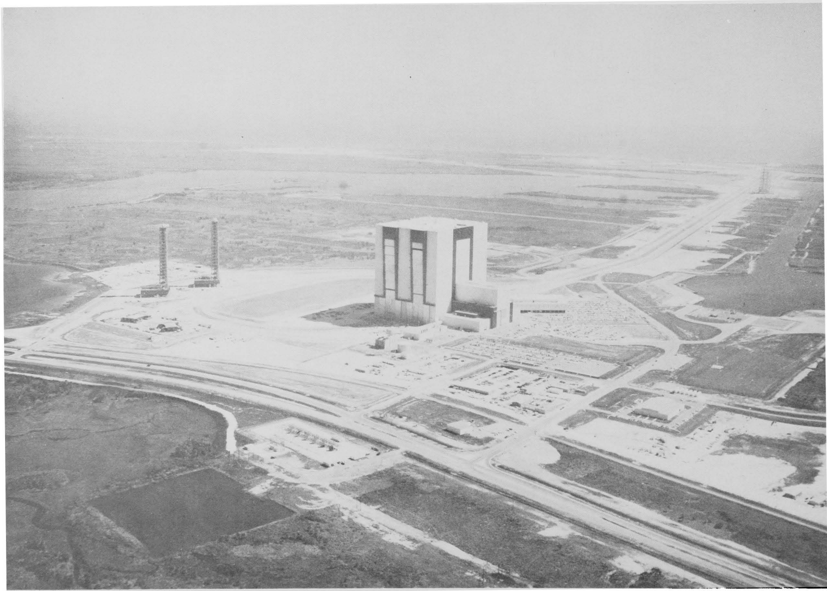
Vehicle Assembly Building dominates moon Launch Complex 39 at NASA's Kennedy Space Center. Towers at left are Mobile Launchers, on which the Apollo-Saturn V will be erected in the VAB and then be taken over the Crawlerway (right of center) to the launch pads in the background. Dock area, where rocket stages arrive, is at right.
