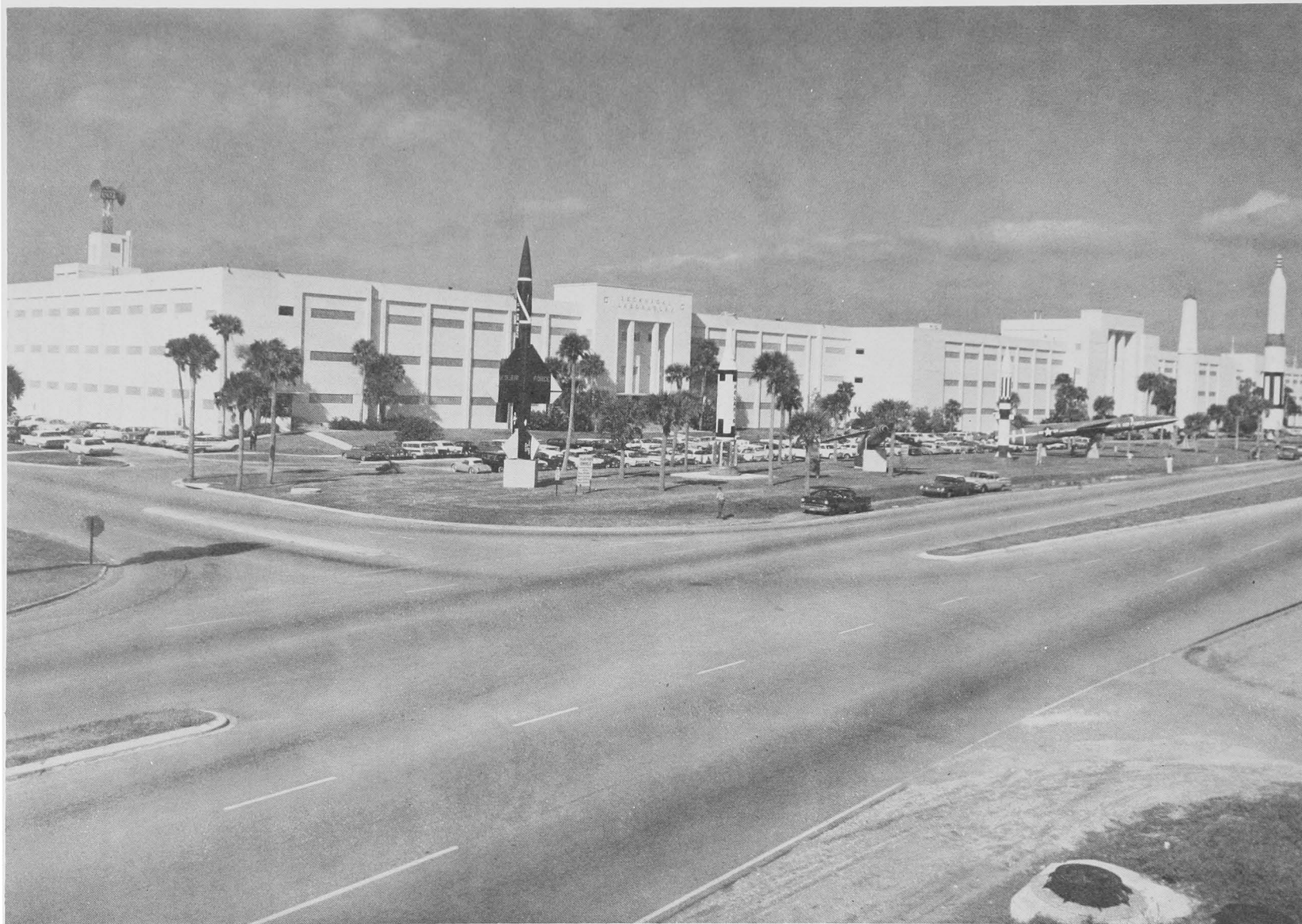
Giant Technical Laboratory built by Corps for Air Force at Patrick AFB. Building houses computer complex and related instrumentation and is main hub of data collection for Eastern Test Range.
