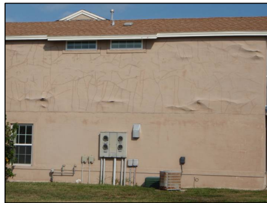
Evidence of damaged stucco on residential unit.
