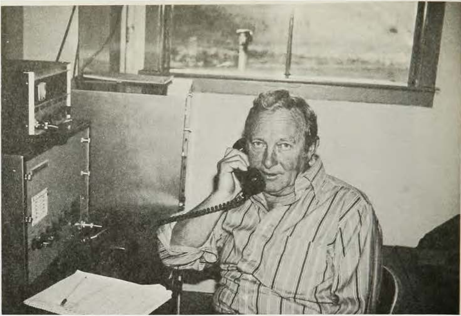
Francis J. Hogan, clerk and principal radio operator. Lower transceiver is a model CA-27B made by Communications Associates; upper unit is a model SBA-310M made by Sideband Associates.
