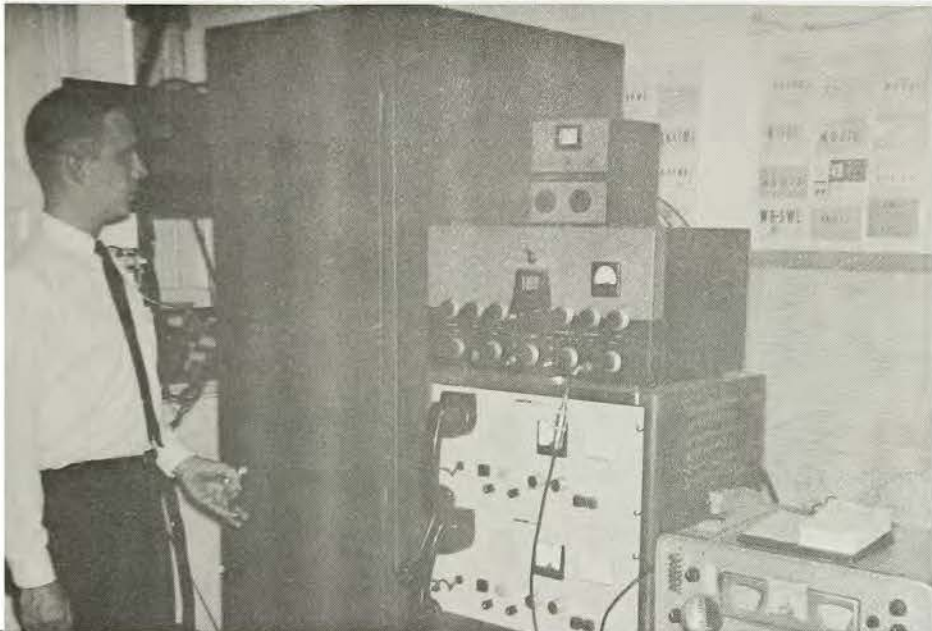
In this 1964 photo R. A. (Dick) Wilkinson (K3DVR) is shown examining the new Westrex single sideband equipment. Above the Westrex control unit are the old Johnson Viking II AM transmitter and VFO which were kept for use on AM nets. The Hammarlund HQ-180 receiver is at extreme right.
