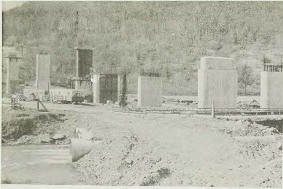
Before the dams could be built, U. S. 15 had to be relocated. These piers, shown under construction in May 1974, will carry highway across Mill Creek.
