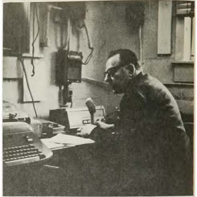
Edward F. Kerns, construction inspector, is here shown at the console of the VHF base station. Through a repeater system this station can communicate with District boats on Chesapeake Bay or the Potomac River.
