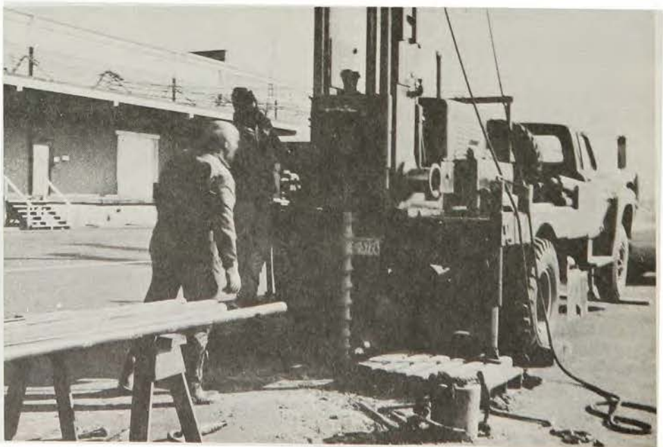
Auger boring to get samples of foundation material.
