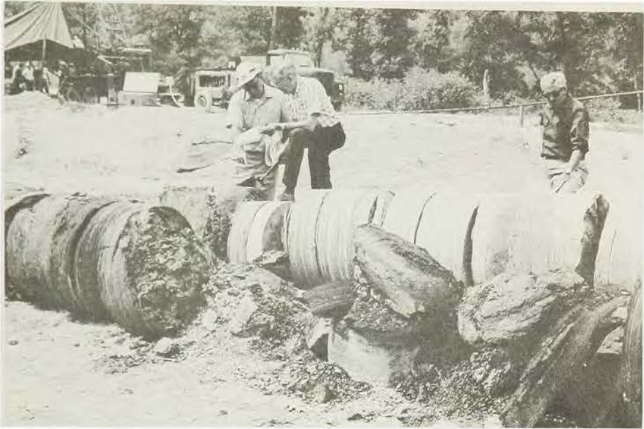
Above: Sandstone and shale core removed from one of two 36-inch-diameter calyx holes drilled to investigate foundation for spillway at the Bloomington project.
