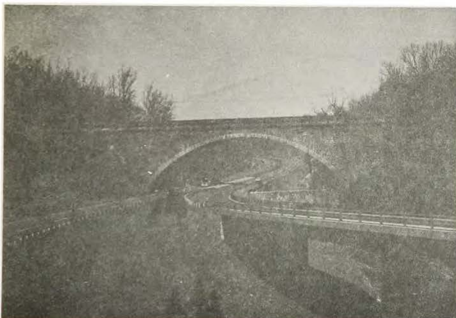
Six miles downstream from the intake the Cabin John Bridge carries the gravity conduit across a valley. This pipeline, completed in 1863, is still a major part of Washington's water-supply system.
