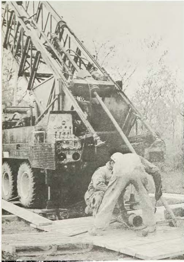
Above: Drilling 6-inch-diameter rock core at 52-degree angle to get samples for testing of clay seams at Tioga-Hammond Dams.
