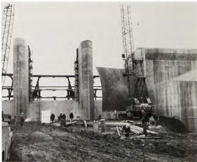
One of the three 45 x 49 foot Tainter gates being installed in the spillway section of the Shelbyville Dam.
