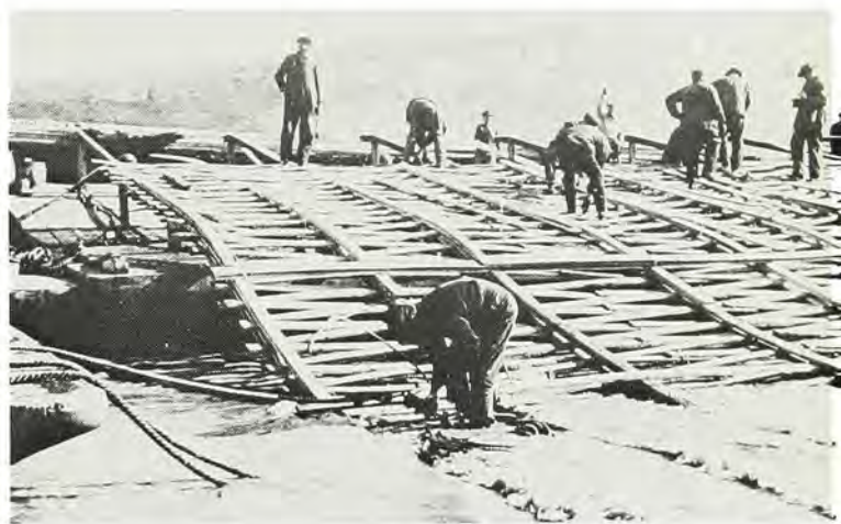
Engineer employees laying a lumber mattress revetment.
