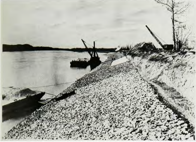
Rip-rap being placed on banks to prevent erosion. In earlier days, rip-rap was placed by hand.
