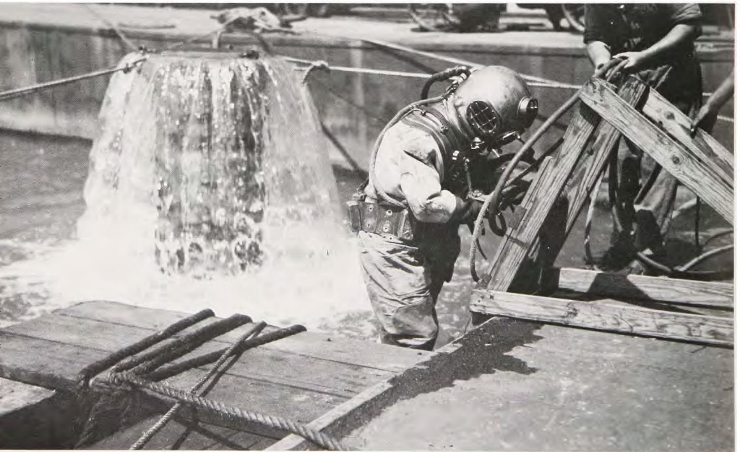
Almost from the beginning, Lock #26 experienced problems. Here a diver descends to investigate a section of the dam where an unusual discharge was indicated.
