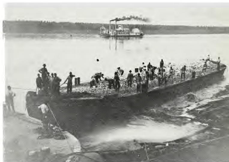
Mattress revetment was sunk into place by the use of large rocks, as shown in the picture.
