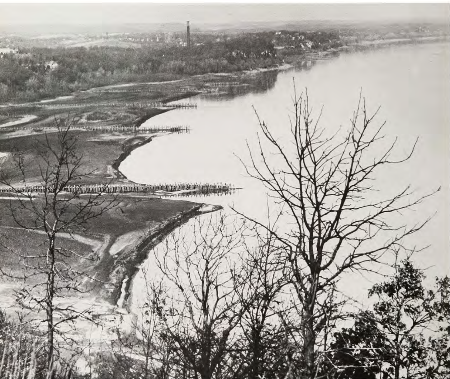
Dikes that function properly, causing accretion of sand and restricting the channel of the river. Herculaneum, Missouri, is in the background.
