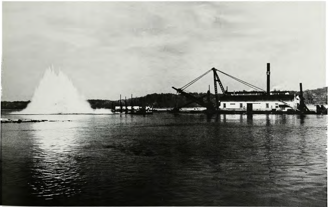
Modern river work includes the use of dynamite to remove rocks, as pictured here in the Thebes, Illinois—Commerce, Missouri, area. The dredge Keokuk is seen working at right.
