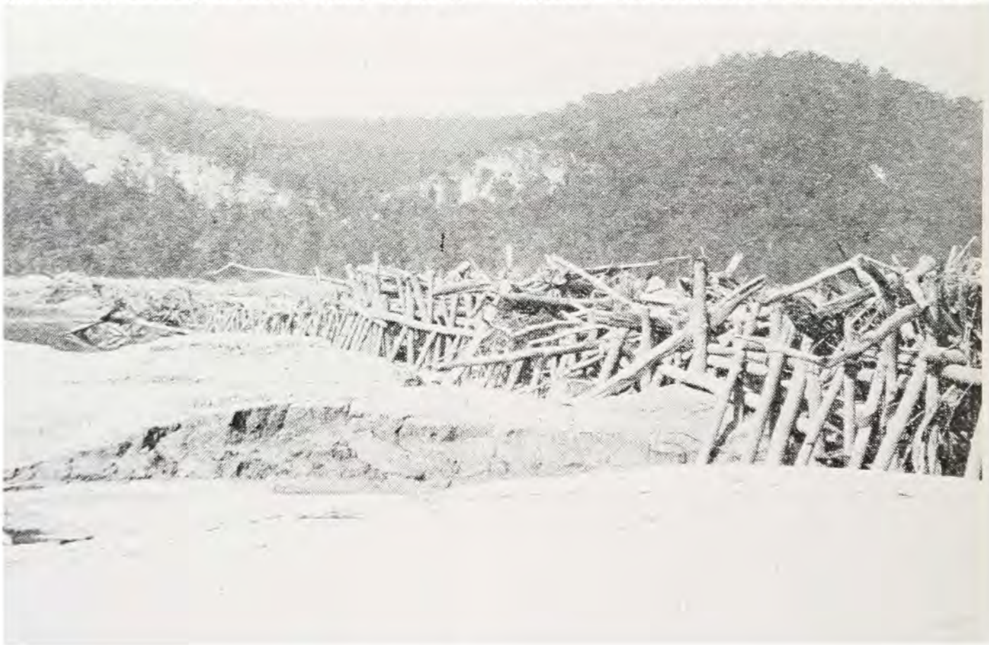
The results of an effective hurdle or piling dike is an accumulation of drift above the hurdle and a deposit of sand below.
