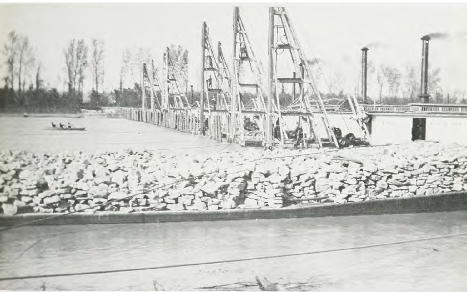
Piling dike or hurdle being constructed.
