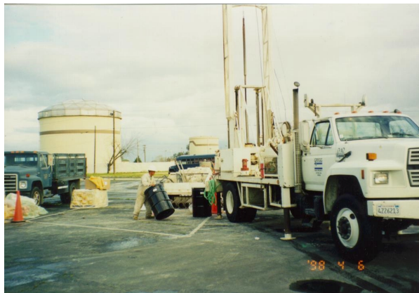
Photo 3. Mobilization of support equipment.
