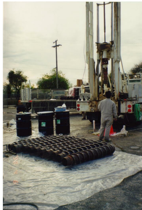
Photo 2. Setup of drill rig.
