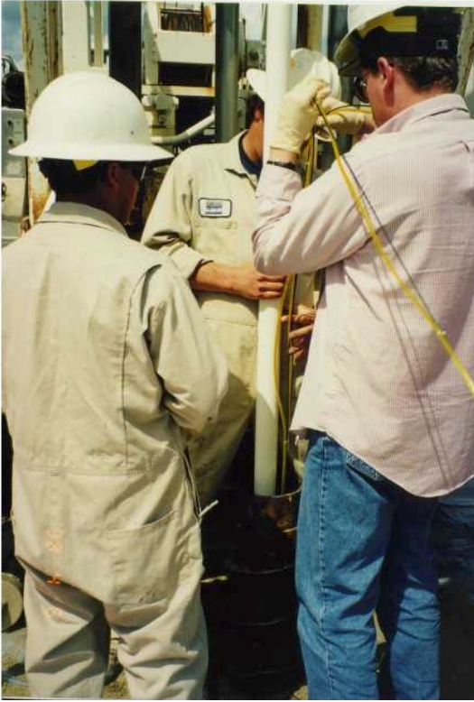
Photo 6. Installation of sensor through hollow stem auger.
