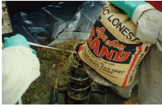
Photo 7. Placement of sand filter pack.
