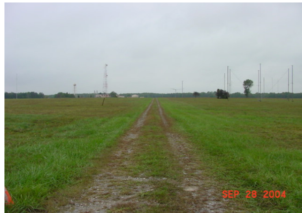
Access Road from Central Building Facility
