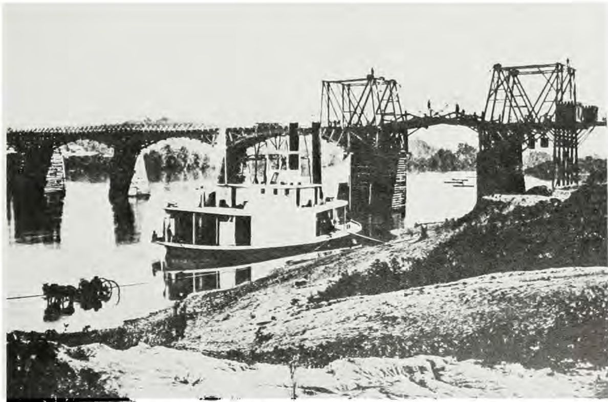
The wooden bridge, complete with draw span, built by Union Army Engineers at Chattanooga in 1865 was destroyed by the record flood of 1867.
