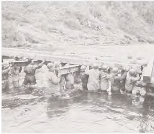
Combat Engineers build a bridge in Korea, 1951. Note the log crib pier.
