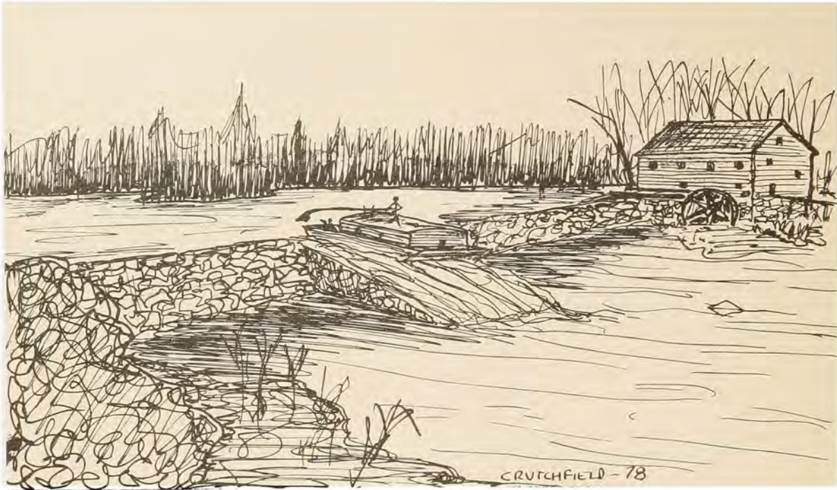
Navigation laws required mill dams to have sluices for flatboats.
