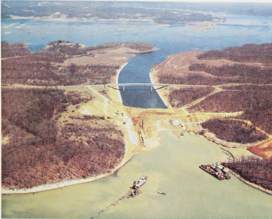
Barkley Canal under construction on March 31, 1966. Dredges are removing the canal plug.
