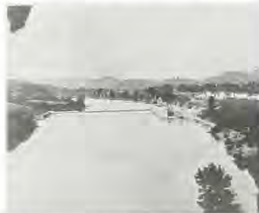
Lock 7, Cumberland River, on September 28, 1914. The District was raising the walls of the lock three feet at this time.
