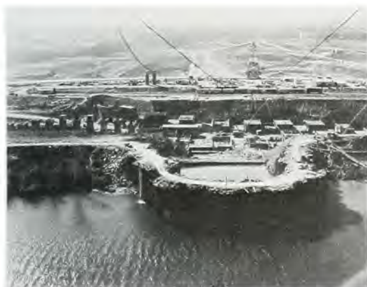
Construction inside the cellular cofferdam at the Old Hickory project on the Cumberland River.
