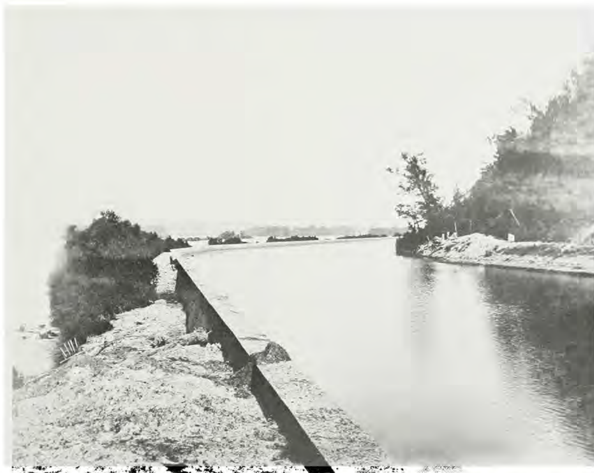
A sharp turn in the Colbert Shoals Canal, Tennessee River, about 1900. Inspectors are standing on the concrete wall next to the waste weir. Colbert Shoals are in the background.
