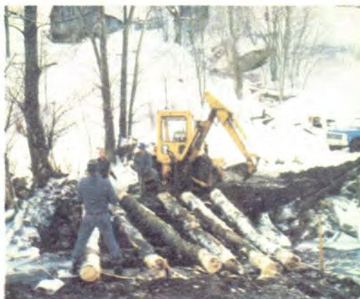
Building a temporary access bridge in North Carolina, winter of 1977-78.
