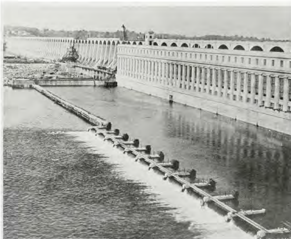
Wilson Dam and powerhouse on September 25, 1925. 280,000 horsepower electrical generators were installed in the powerhouse.
