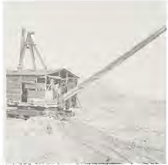
Steam powered crane used in 1895 during construction of Colbert Shoals Canal, Tennessee River.
