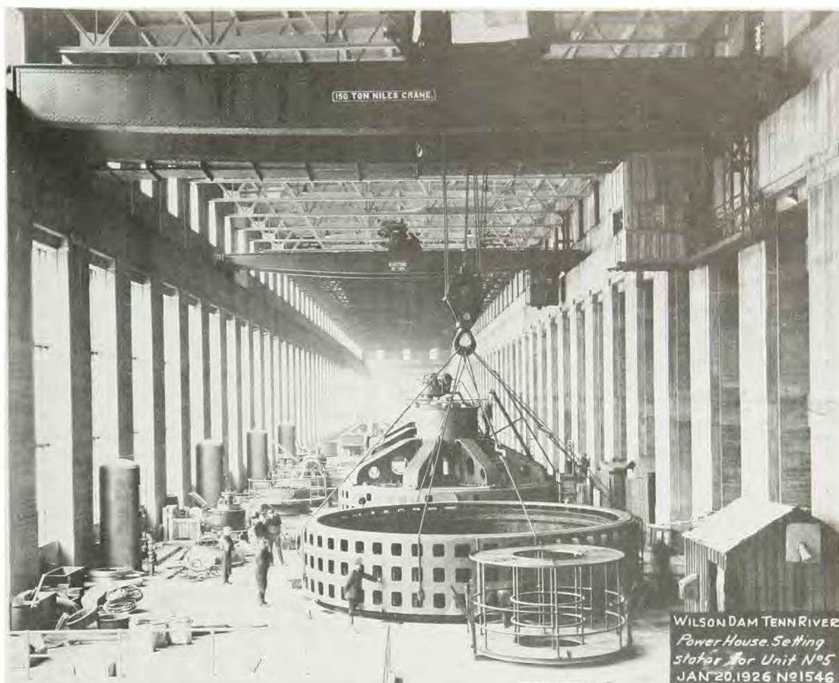
Installing the Wilson Dam power generators, 1926.
