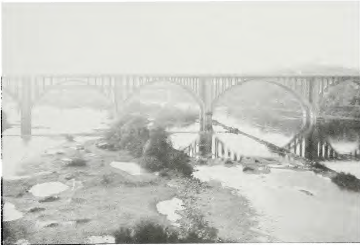
Tennessee River at Knoxville before multipurpose development. Note the riprap dikes confining river flow to a well defined channel.
