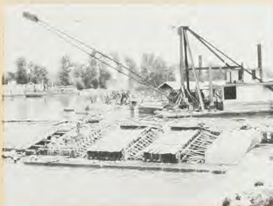
Placing concrete caps atop the old timber-crib dams on the Cumberland about 1935.
