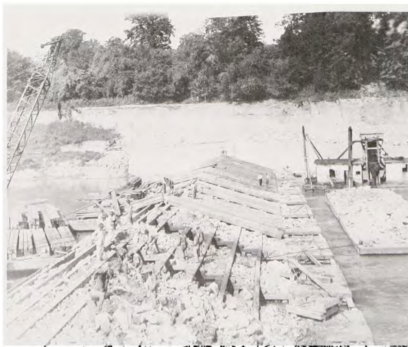
Capping the timber-crib Dam No. 8, Cumberland River, about 1921.
