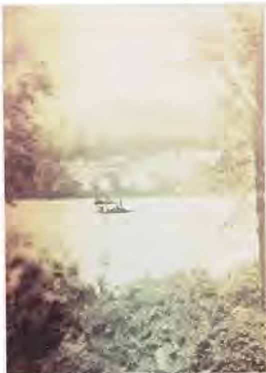
Engineer drillboats were exploring the foundation of Wilson Dam in this 1916 picture.
