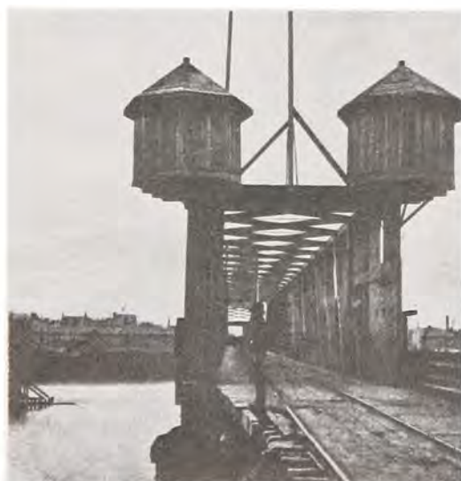
Union Army Engineers repaired and fortified the railroad bridge over the Cumberland at Nashville.
