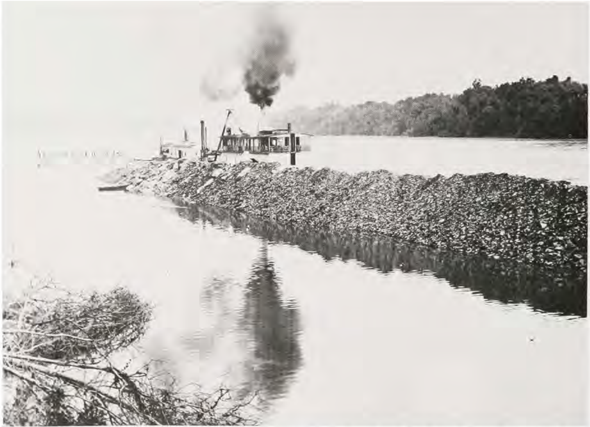
Engineer dredges and drill raft constructing riprap dam to concentrate river flow at Big Bend Shoals, Tennessee River, 1913.
