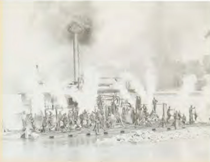
Thacher drill raft in operation at Big Bend Shoals, Tennessee River, about 1910. After holes were drilled in the rock, it was blasted and removed. Note the work force is almost entirely black.
