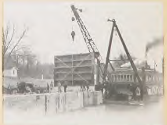
Derrick boat raising lock gate for repairs at Lock A, Cumberland River.
