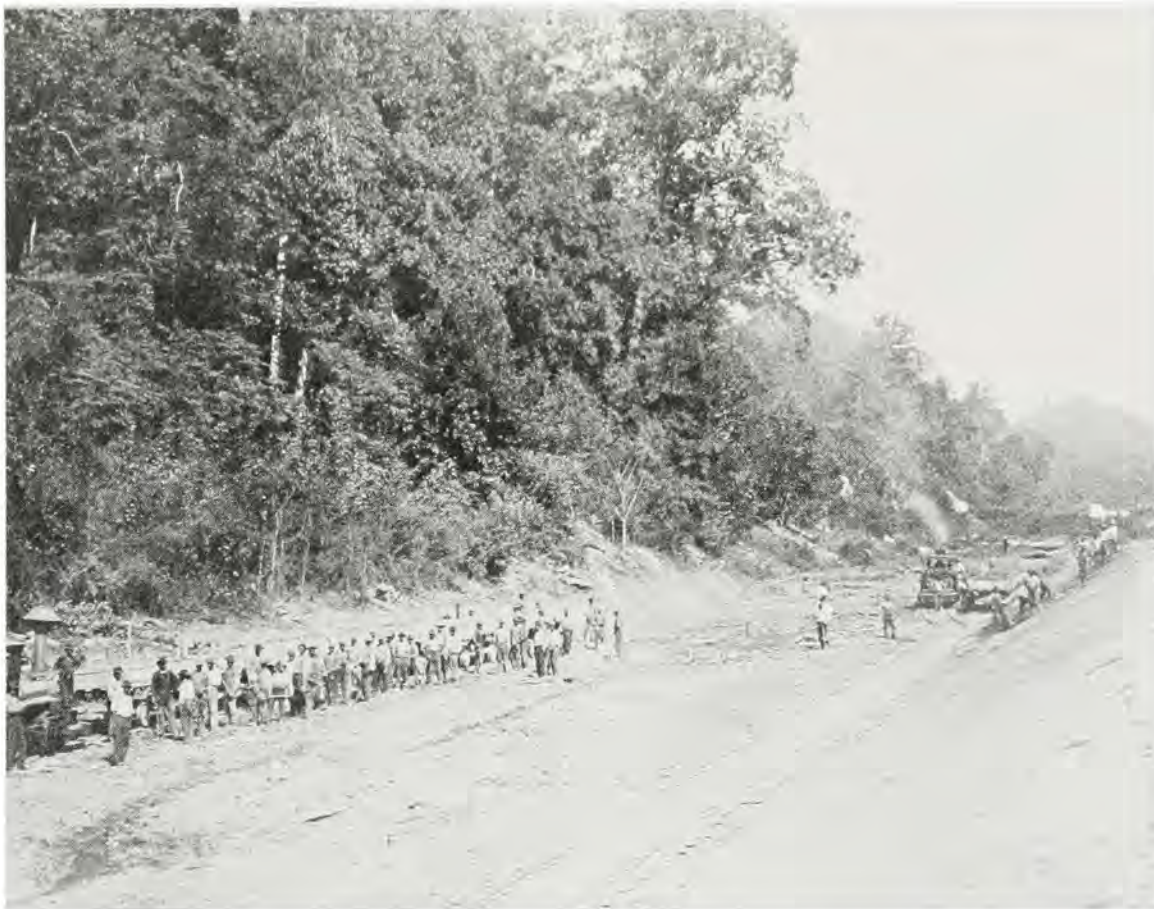
Excavation of Muscle Shoals Canal in August 1881. Spoil was shoveled into railcars running on temporary track laid on bottom of canal section. The work force was almost entirely black.
