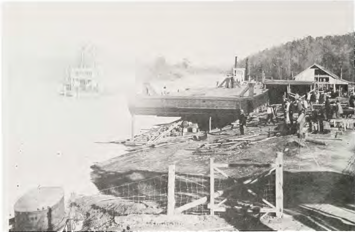
Engineer dock and repair shop on Colbert Shoals Canal about 1905. Engineer steamer Colbert moored on opposite bank. The barge in foreground is under construction or repair, with an unidentified steamer behind it.
