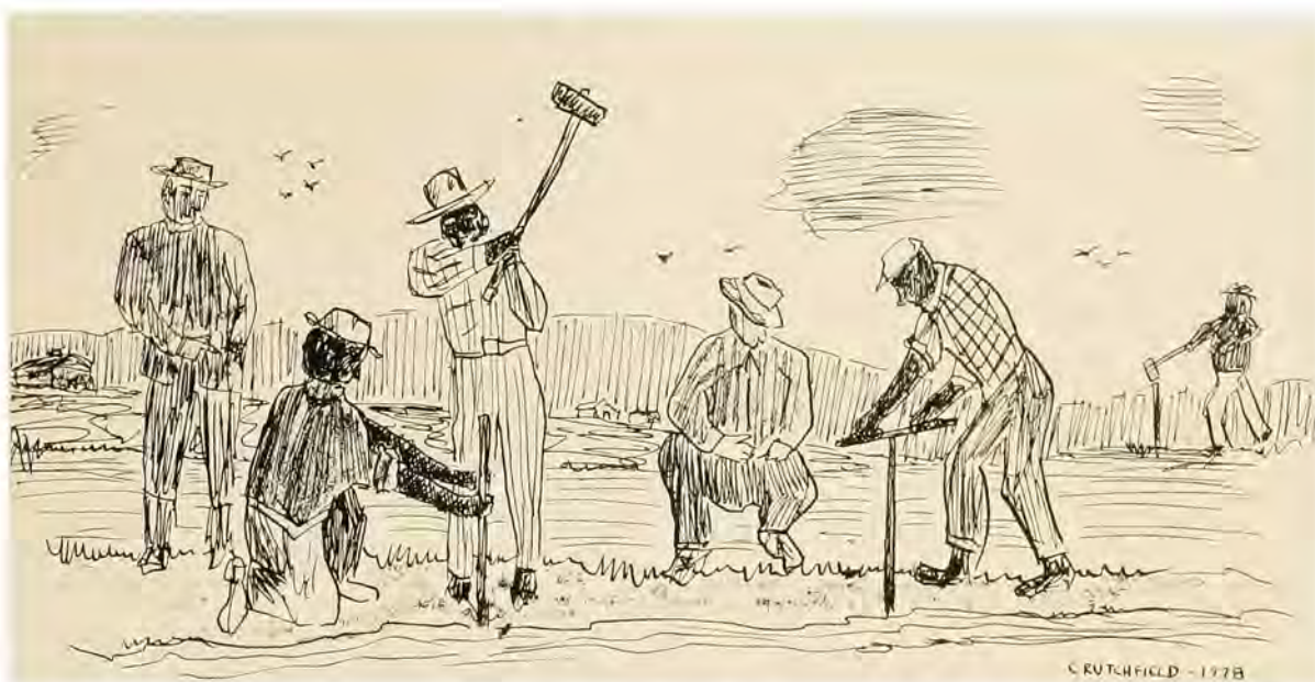
Until about 1890, rock was drilled for blasting by hand.
