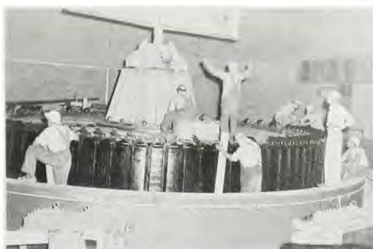
On September 4, 1957, Unit 4 rotor was lowered into place for power production in the generator room of the Old Hickory Dam power plant.
