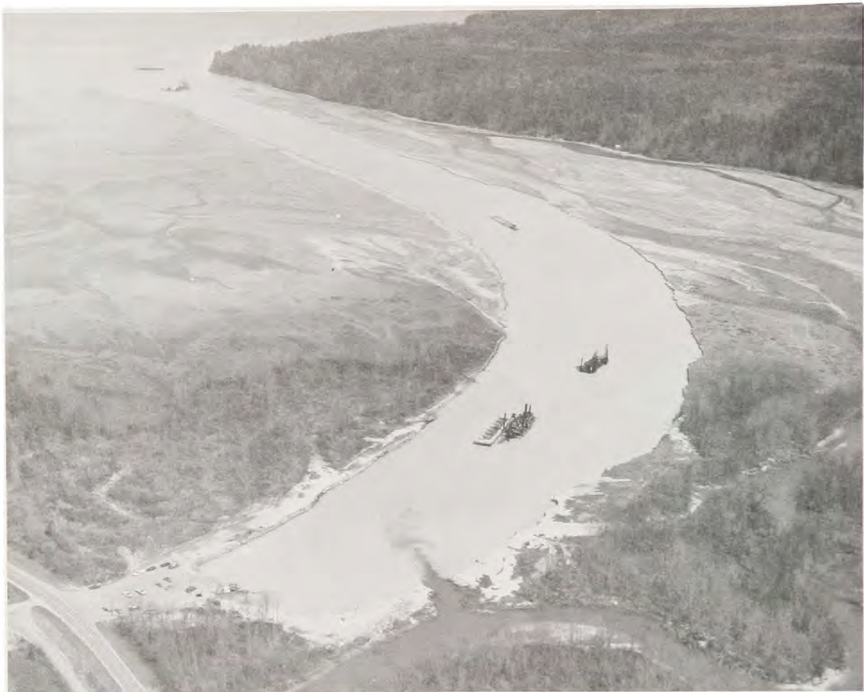
Construction of the Tennessee-Tombigbee Waterway: dredging Yellow Creek embayment at Highway 25 in 1976.
