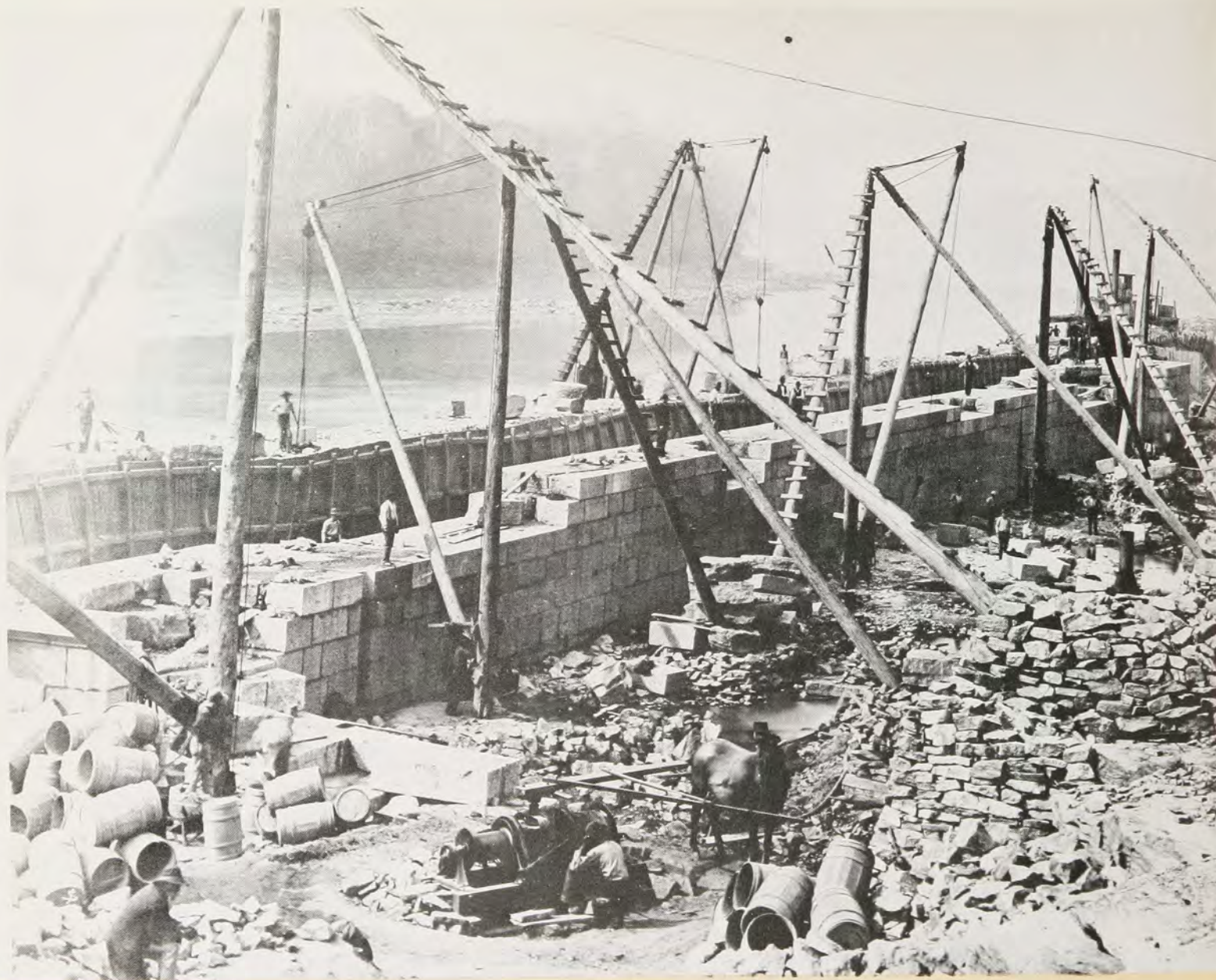
Construction of Lock 1, Cumberland River, on October 31, 1891. The barrels may have contained cement; the horse turned the drum winding cables to raise the cut stone into place.
