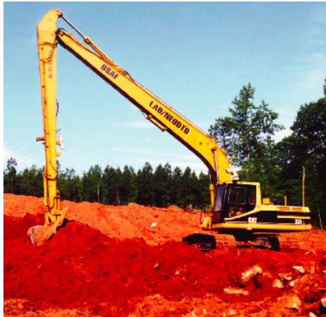
Figure 9-1. The A-AOE robotic system, a modified Caterpillar 325L excavator.
