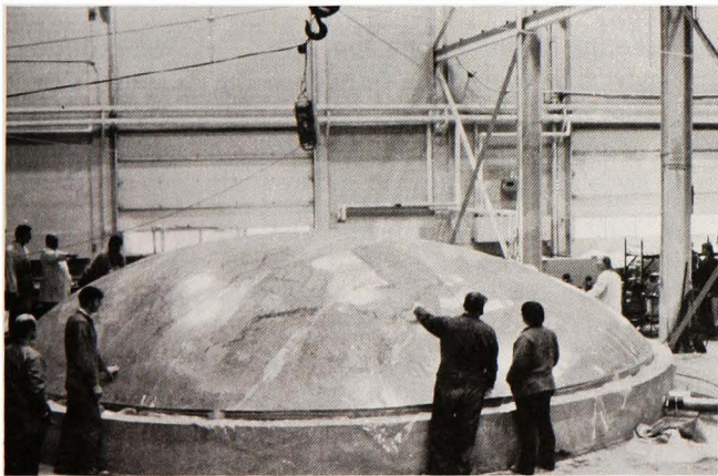
Inflation Forming of a Dome
