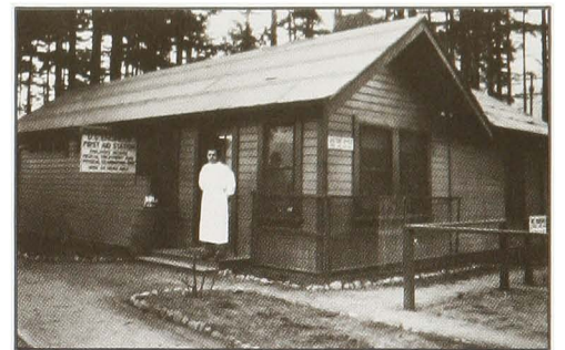
First aid station for Bonneville project workers.
