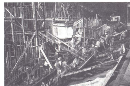
Pouring concrete in powerhouse substructure.
