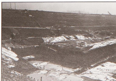
Placing concrete foundation for 2nd powerhouse.
