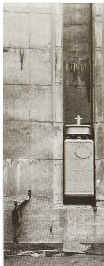
Floating mooring bit installed in lock sidewall.
