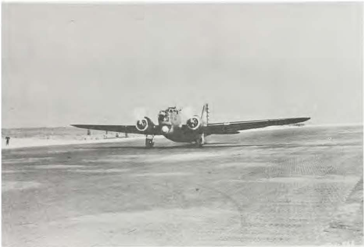
Mat-surfaced runway (PSP)
