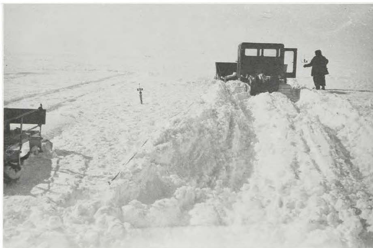
Deep ruts left by standard D-7 Caterpillar tractor after 40 trips in same path on polar ice cap
