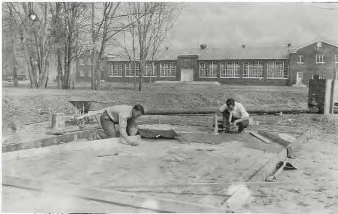
Construction of Bonnet Carré model
