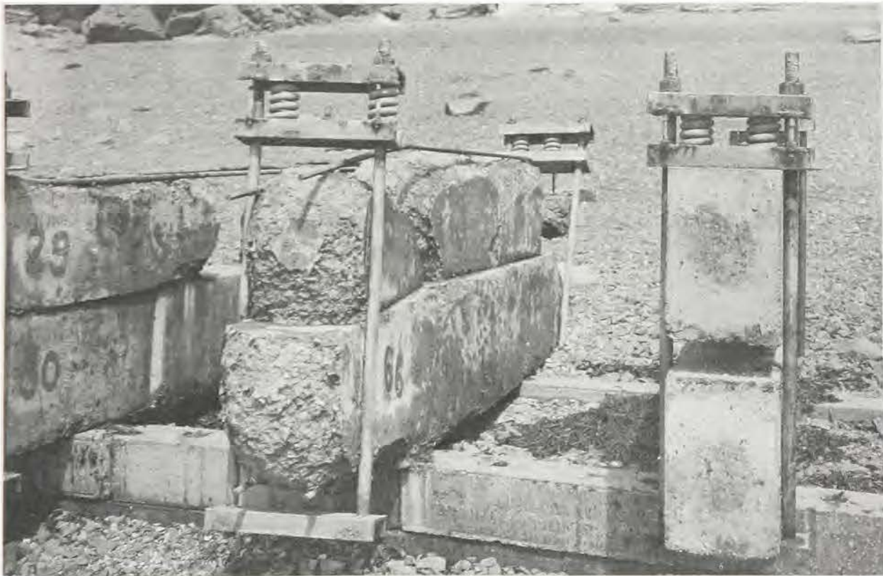
Condition of concrete beams after 1-1/2 years of freezing and thawing cycles and tidal inundation at Treat Island, Maine, weathering station
