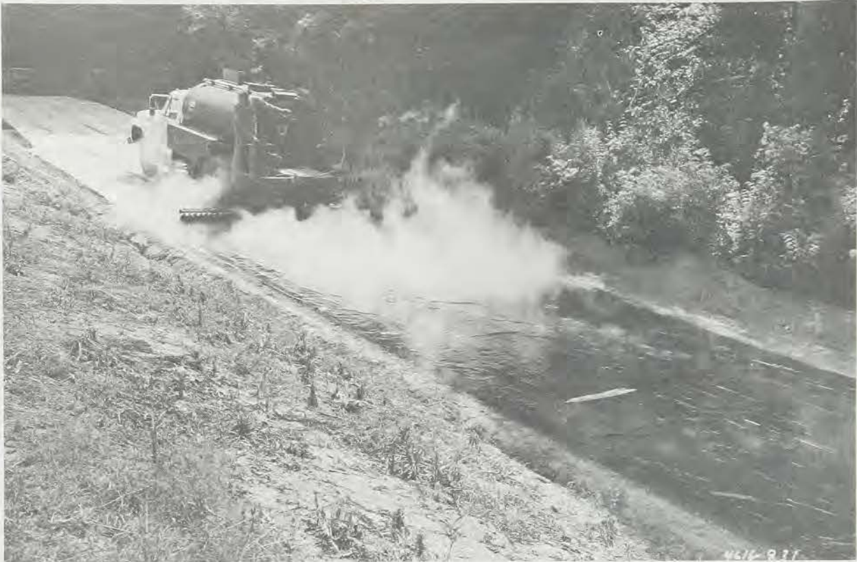
Final application of asphalt over polypropylene on experimental road at WES
