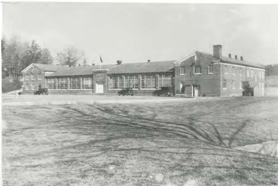
Completed original building
