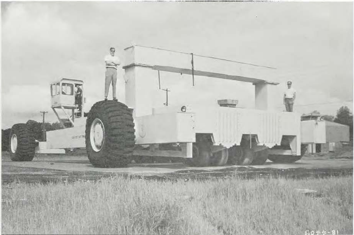
Large test load cart used in designing C-5A landing gear configuration
