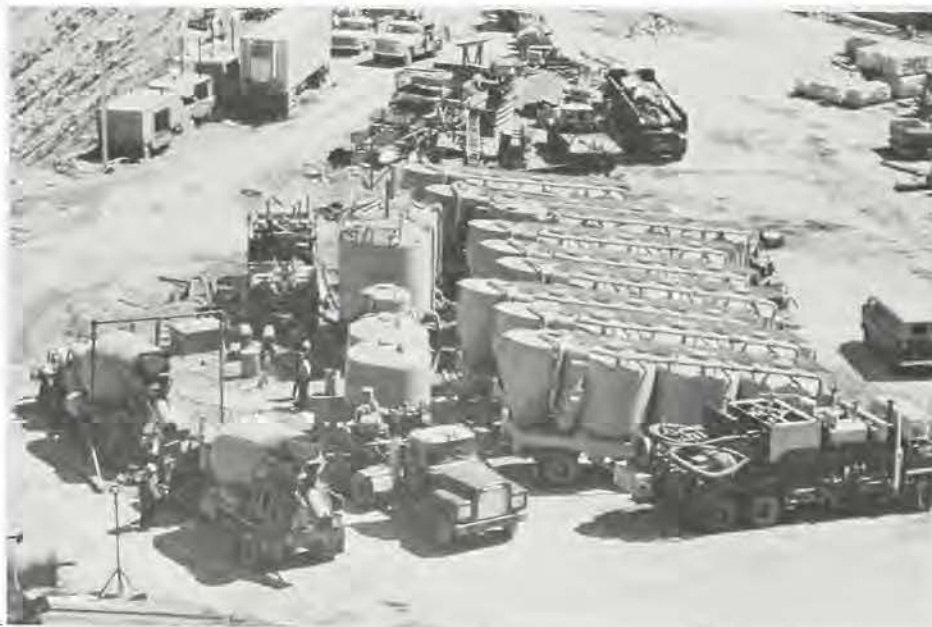
Grouting equipment at Nevada Test Site in support of weapons testing
