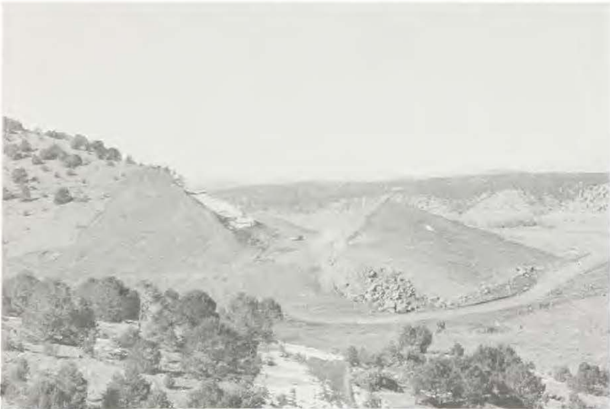
Railroad cut made by explosives
