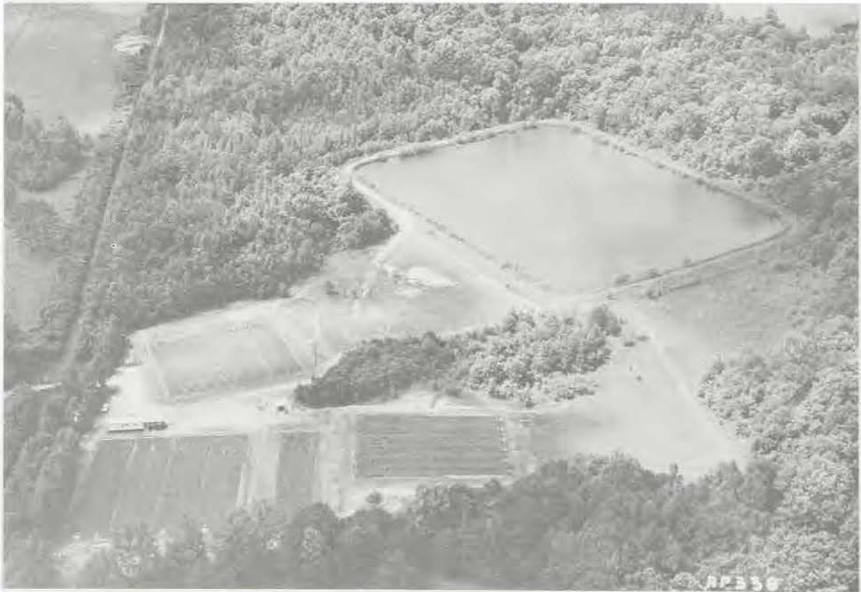
Overland flow treatment of wastewater, Utica, Miss.
