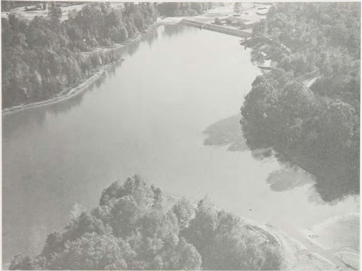
Early photograph of WES dam and lake
