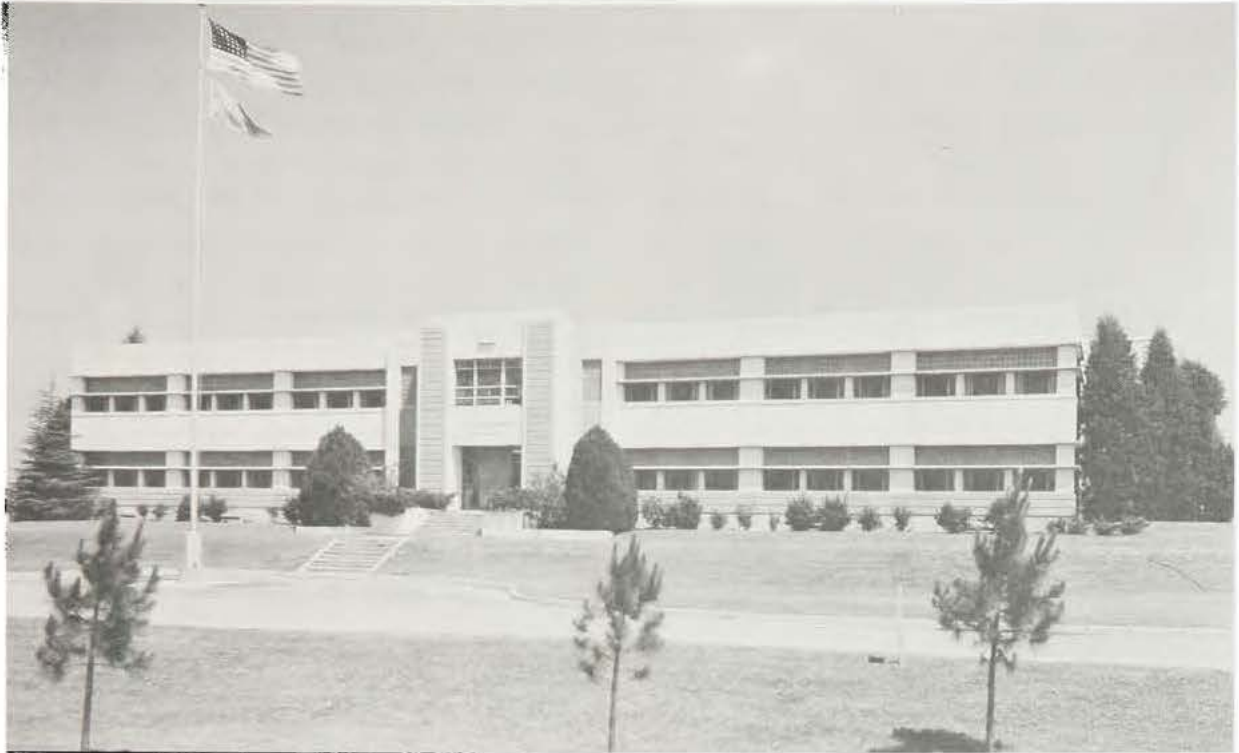
Concrete Division office and laboratory building, Jackson Reservation, 1946
