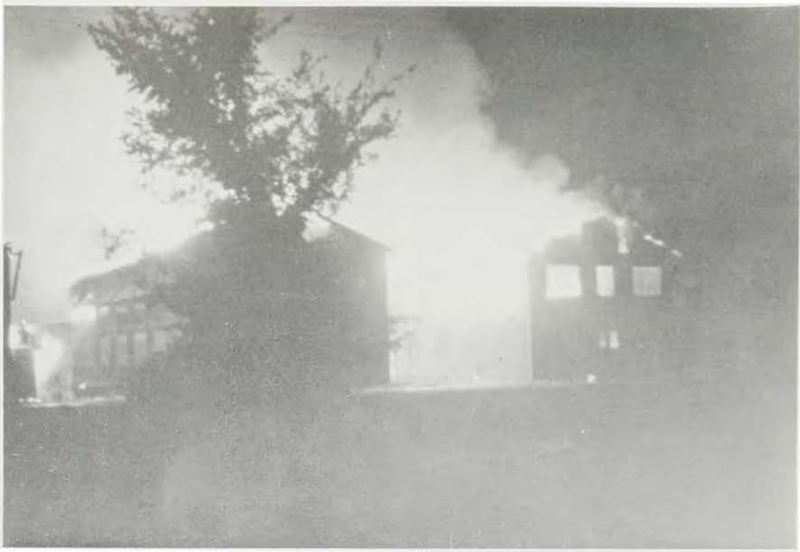
Back of burning Administration Building
