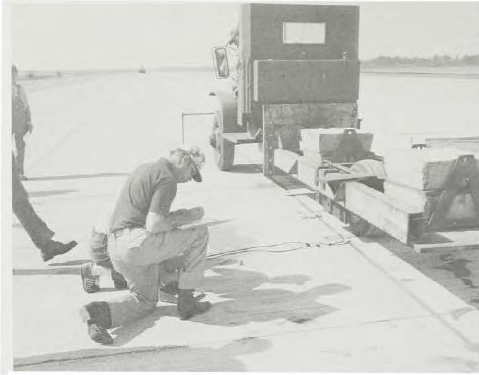
Instrumentation testing of dowel joint performance in airport pavements
