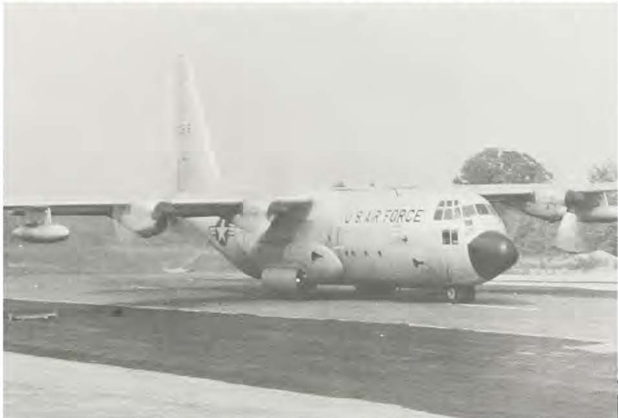
C-130 aircraft operating on membrane-surfaced runway
