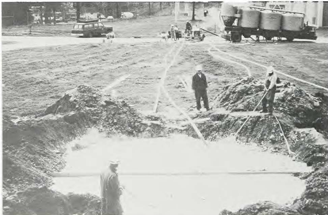
Placement of foam concrete
