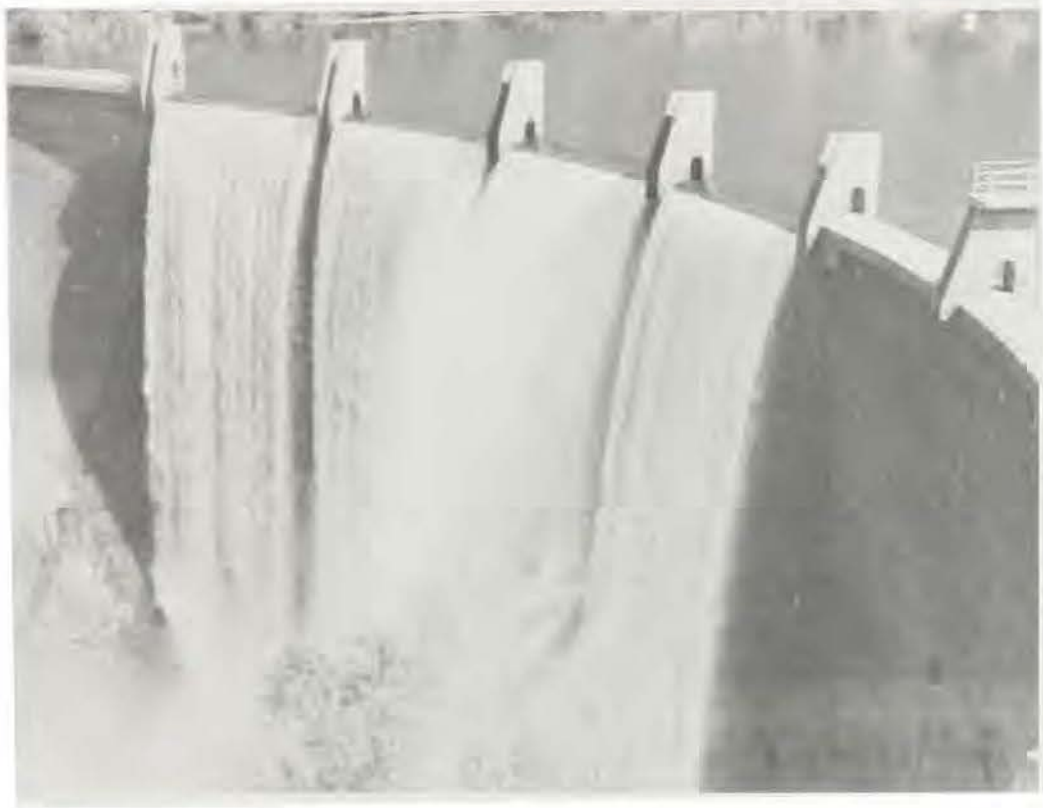
North Fork Dam, prototype
