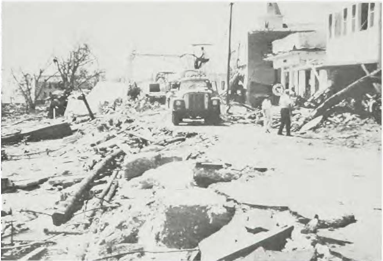
Hurricane Camille damage
