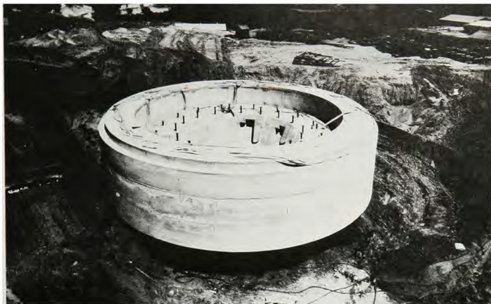
Gun block No. 1 during backfilling and tamping – Battery Davis – April 1937.
