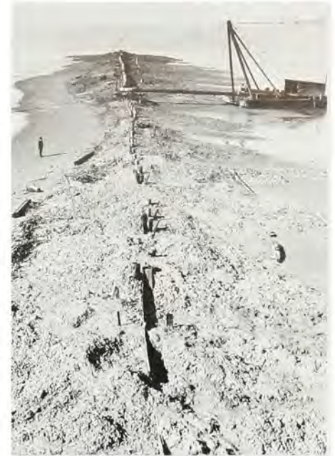
Richmond Harbor – September 1922. Discharge end of pipe is about 200 feet from shore.
