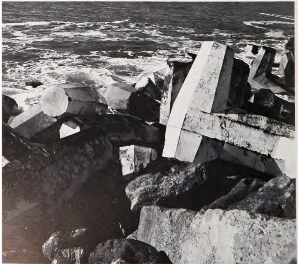
Dolosse armor units were placed on top of the rock and tetrapods placed earlier.
