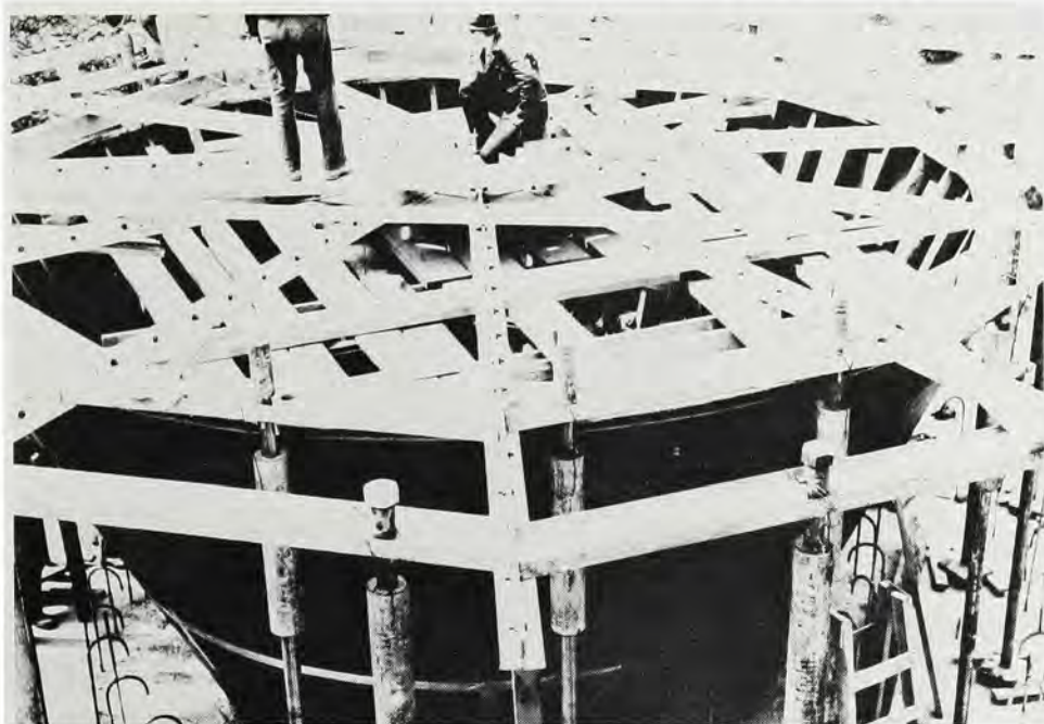
Anchor bolts go into place at Battery Townsley – April, 1939.
