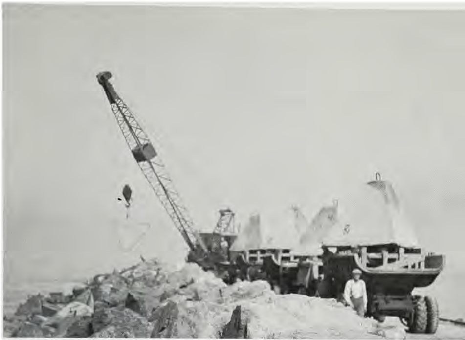
South Jetty, Humboldt Bay. Placing tetrahedrons on south slope – September 25, 1939.
