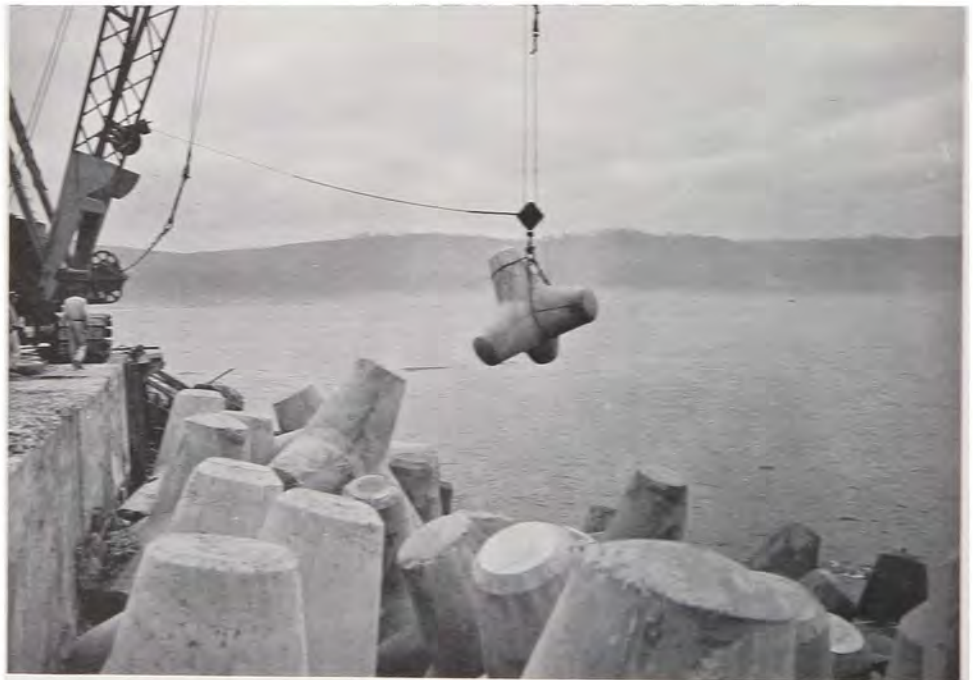
Broken tetrapods show the effects of damage suffered during 1964 Christmas storms.
