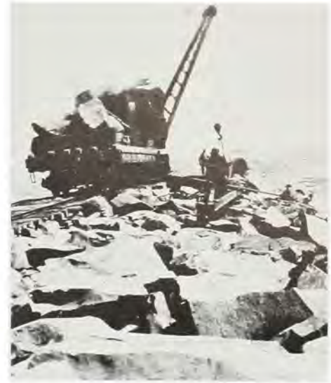
Placing stone on the breakwater – July 1921.
