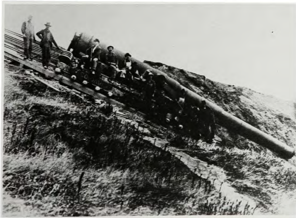
A large gun, mounted on a modified rail carriage, is moved into place at Battery Mendell.
