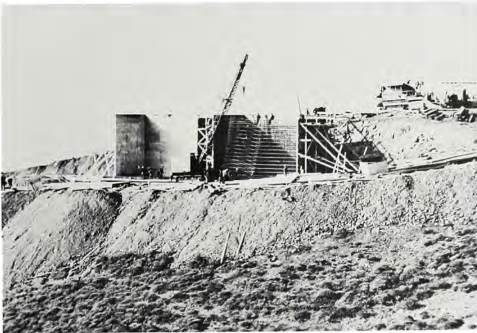
Forms are shown partially complete for the large caliber test — December, 1941.
