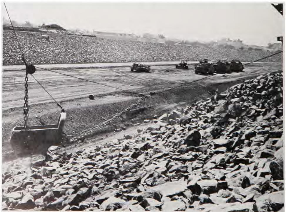
Rock being placed along Alameda Creek for flood protection.
