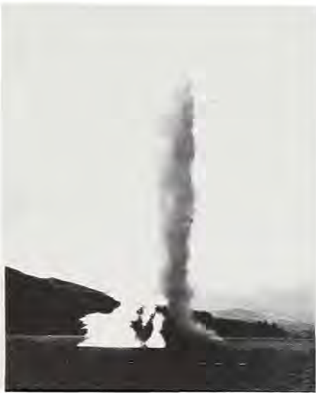
Explosion of surface blast on Shag Rock, No. 2, San Francisco Harbor. September 5th, 1900. Quantity of explosive: 21,169 lbs. of nitro-gelatin. Height of column: 1,120 ft.
