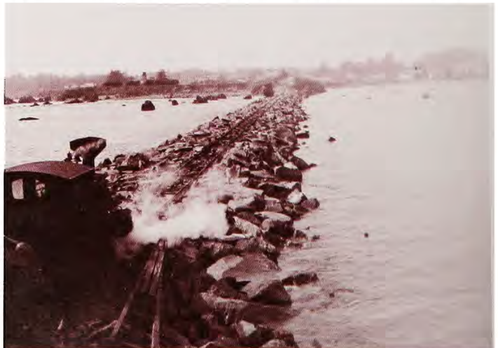
Small work train returns to quarry after delivering stone to the end of the breakwater—July 1922.
