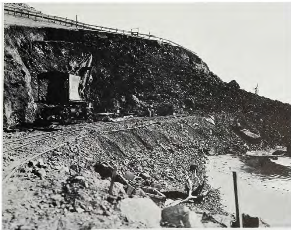
Richmond Harbor – April 1923. The Corps of Engineers' power shovel works in the quarry near the harbor to secure rock material for the training wall.
