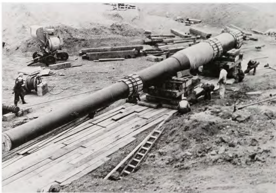
Moving the gun from one place to another required patience and careful placement of timbers and rollers.
