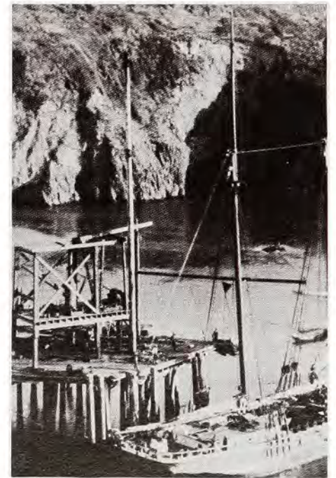
A steam winch is used to load lumber on a schooner headed for San Francisco.
