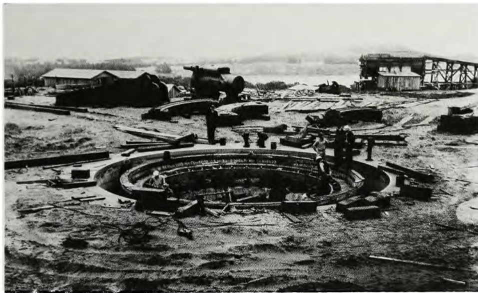
Battery Davis – Fort Funston. No. 1 gun block – placing the base ring, July 1937.
