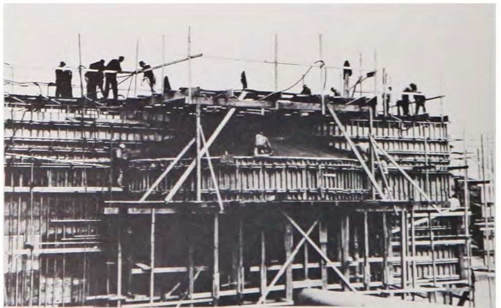
Placing concrete canopy above the big gun of Battery Davis – September 1938.
