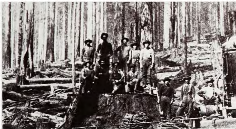
Dolbeer's donkey engine revolutionized the logging industry. Using manila rope and a side-spool, men used the device to snake logs out of the woods.
