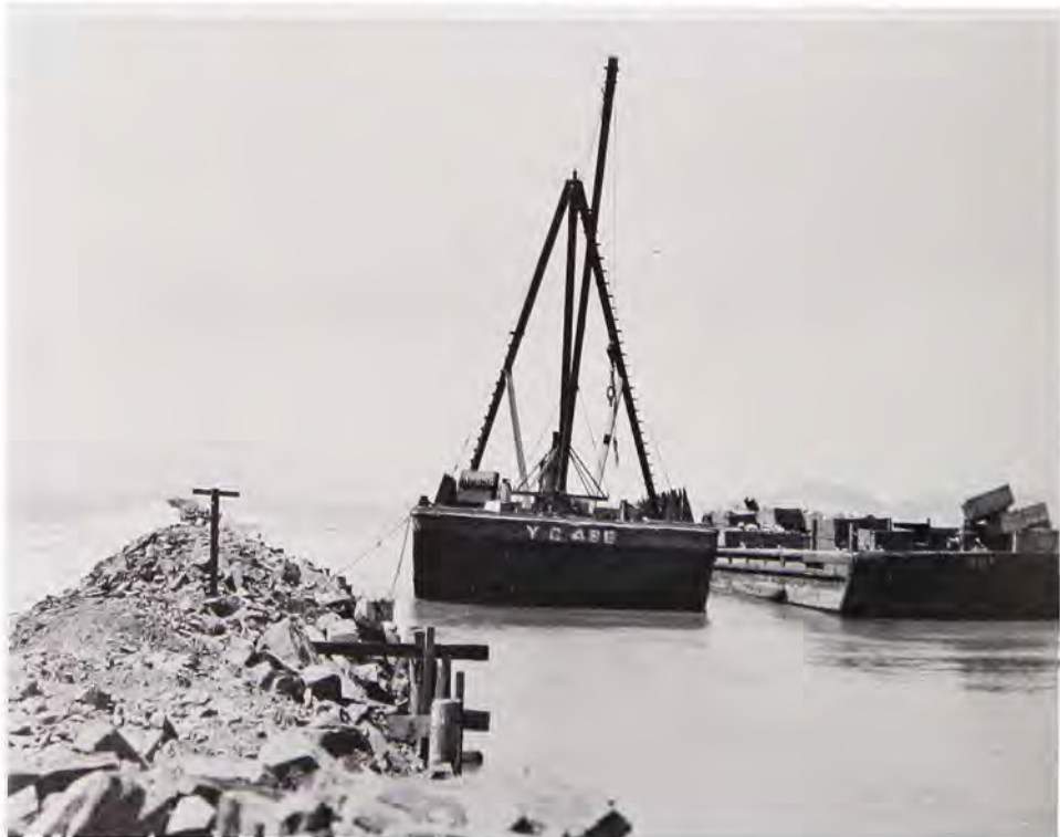
Richmond Harbor – August 1924. A portion of the training wall can be seen with its new covering of rock. A derrick barge and a barge load of rock is tethered alongside. Note the stillness of the water in the harbor.
