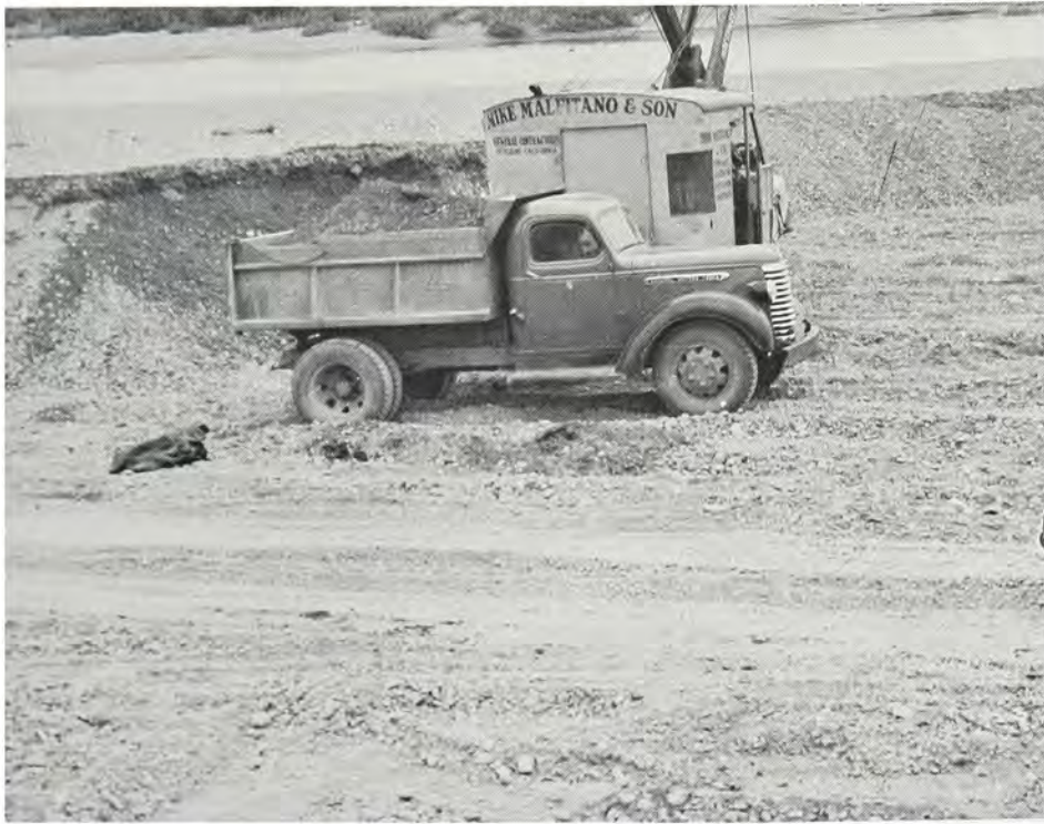
River-run gravel pit located approximately 13 miles from batch plant. Exceptionally clean and well-graded gravel was found. It was conveyed to the batch plant by contractor's fleet of nine trucks which were loaded by a 3/4- yard northwest shovel.
