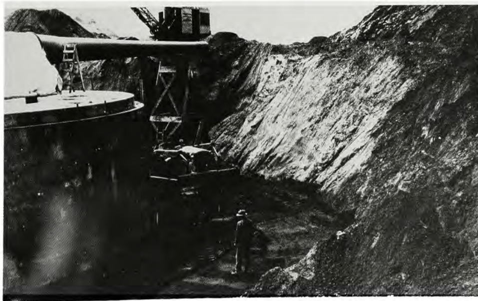
Battery Davis – Fort Funston, 1938 – photograph shows soil stabilization work.
