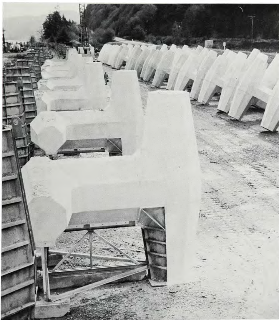
Dolosse ready to be placed on Crescent City breakwater.
