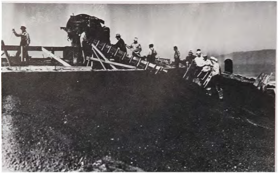
Battery Davis – Fort Funston. Placing concrete in Burster Course, November 25, 1938.
