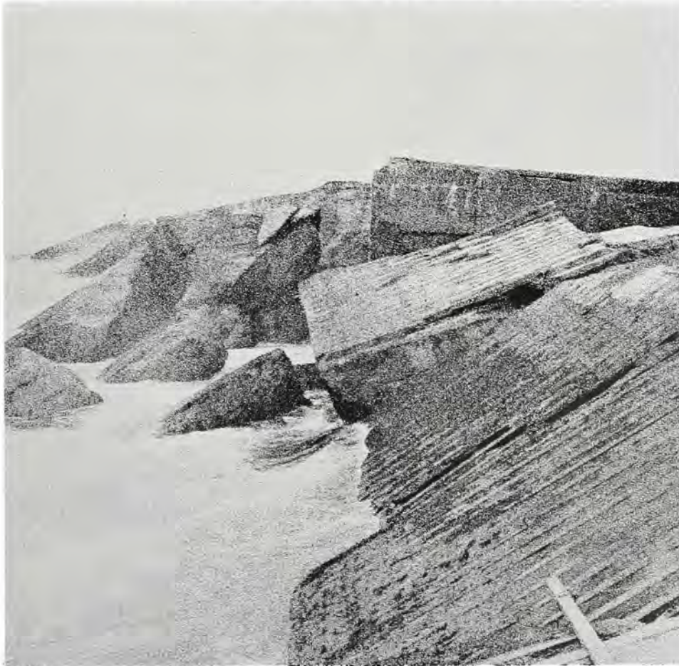
Damage to head end of south jetty before repairs were started.
