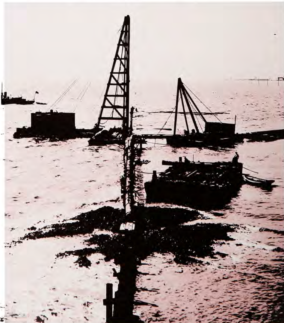
Richmond Harbor work – September 1922. Looking west from Brooks Island, photograph shows fill, pipe line on dike and part of pontoon line. Fill is placed over sheet pile dike to form training wall for the harbor.
