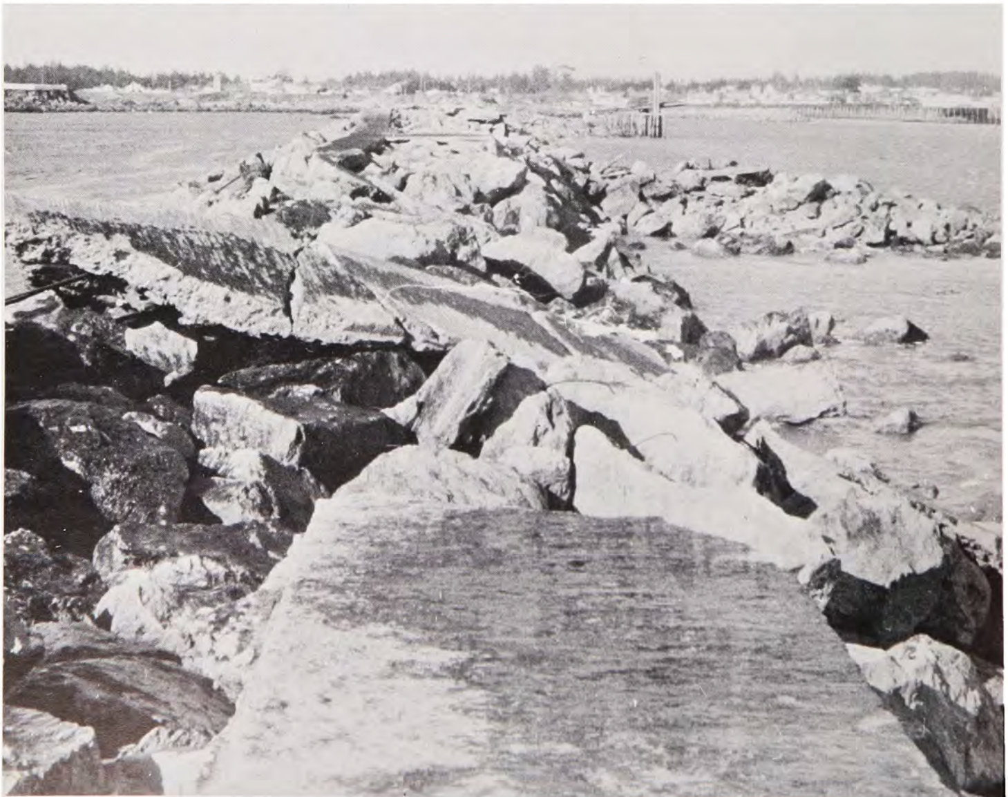
Crescent City Outer Breakwater showing storm damage to barrier during winter 1949-50.
