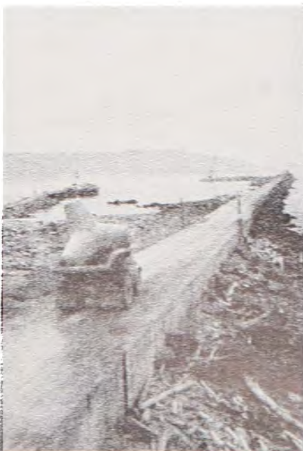
Tetrapod being hauled to placement site on breakwater – Crescent City 1956.
