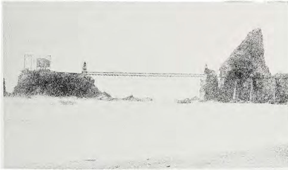
At Rockport, north of Westport, the Rockport Redwood Company constructed a 250-foot iron bridge to a small rocky island so that a ship could load. The bridge lasted but 24 months.
