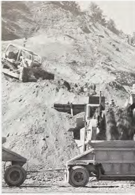
Grading gets underway for the new dam.
