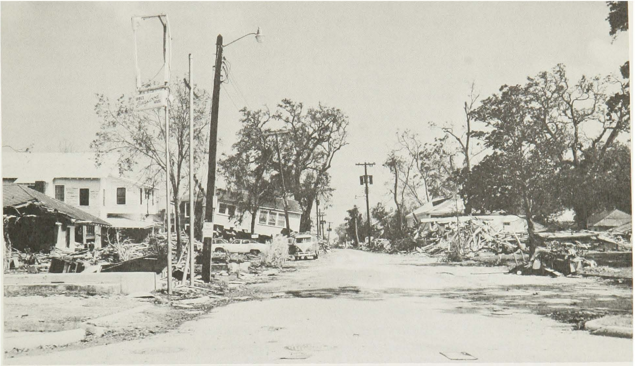
RAVAGED AREA IN GULFPORT AFTER WRECKAGE PUSHED ASIDE FOR ACCESS TO HOMES AND UTILITY INSTALLATIONS BUT BEFORE REMOVAL OF DEBRIS
