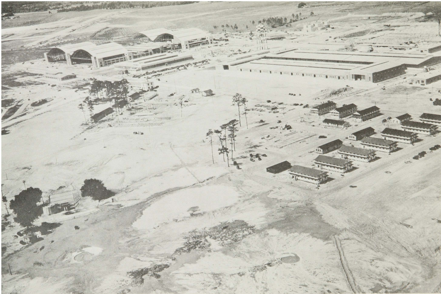
BROOKLEY AIR FORCE BASE UNDER CONSTRUCTION SEPTEMBER 1941
