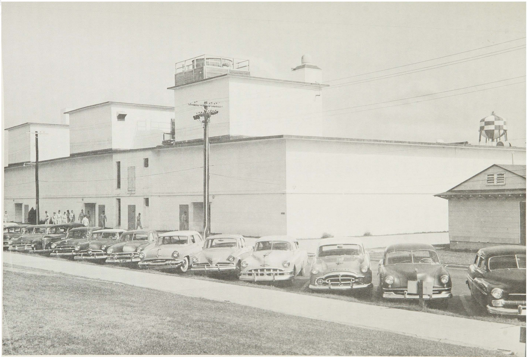
ACADEMIC BUILDING (ELECTRONICS LABORATORY) COMPLETED AT KEESLER AIR FORCE BASE IN 1952
