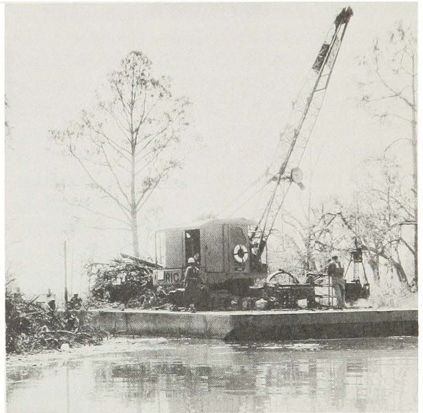
CLEARING STREAM OF DEBRIS
