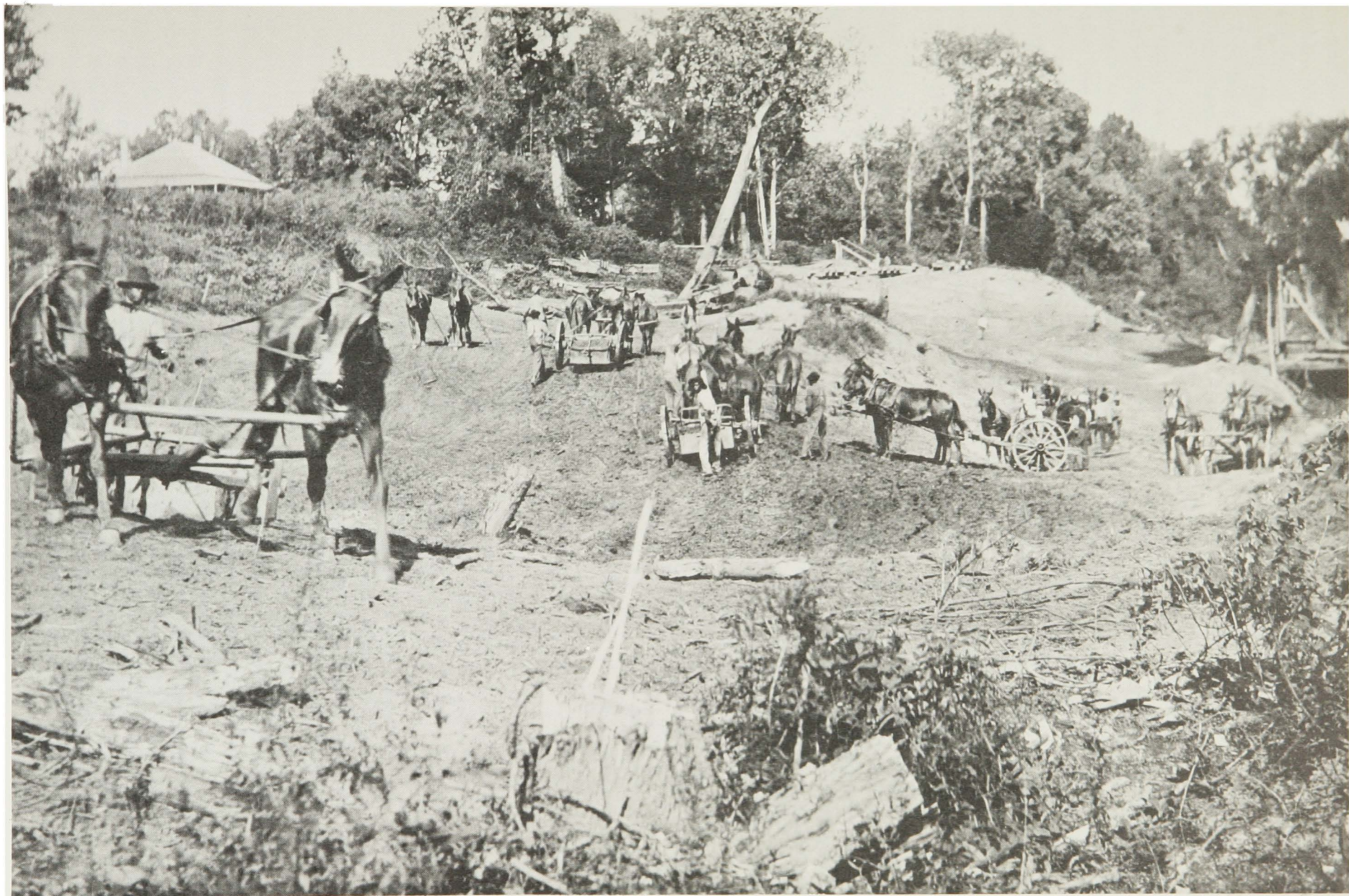
EXCAVATION FOR LOCK 3 ON THE TOMBIGBEE RIVER, AUGUST 1908
