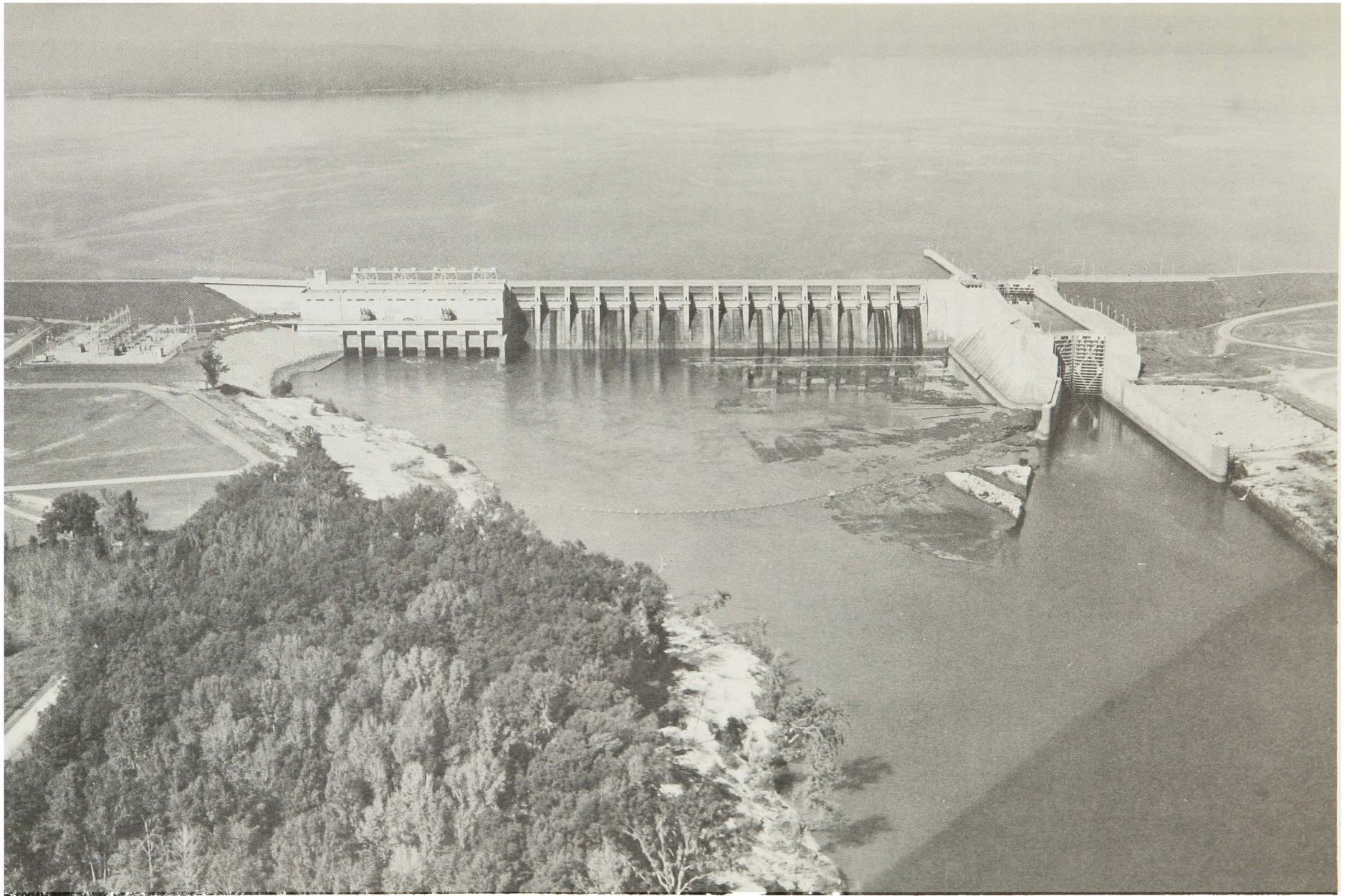
WALTER F. GEORGE LOCK AND DAM, CHATTAHOOCHEE RIVER, ALABAMA AND GEORGIA
