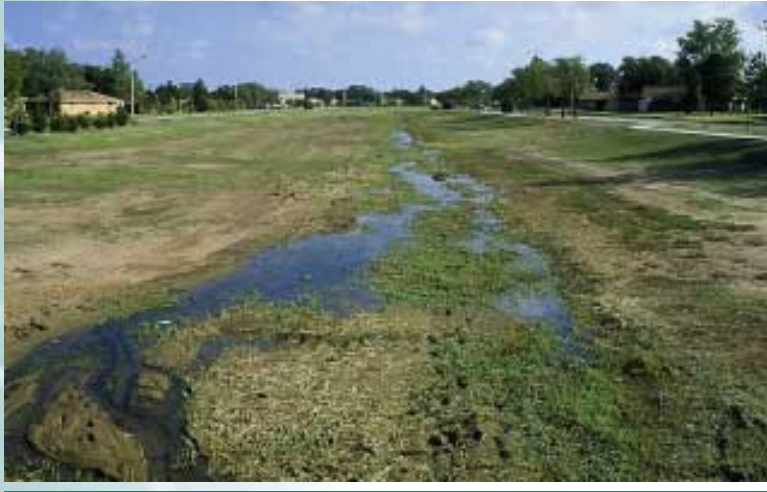
Drainage Way Through Capehart Family Housing Area
