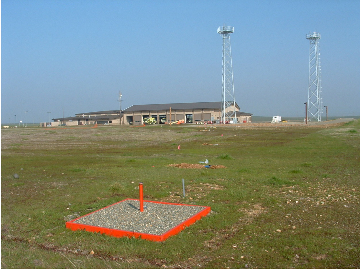
Photo 2 – Line A (northeast view).
