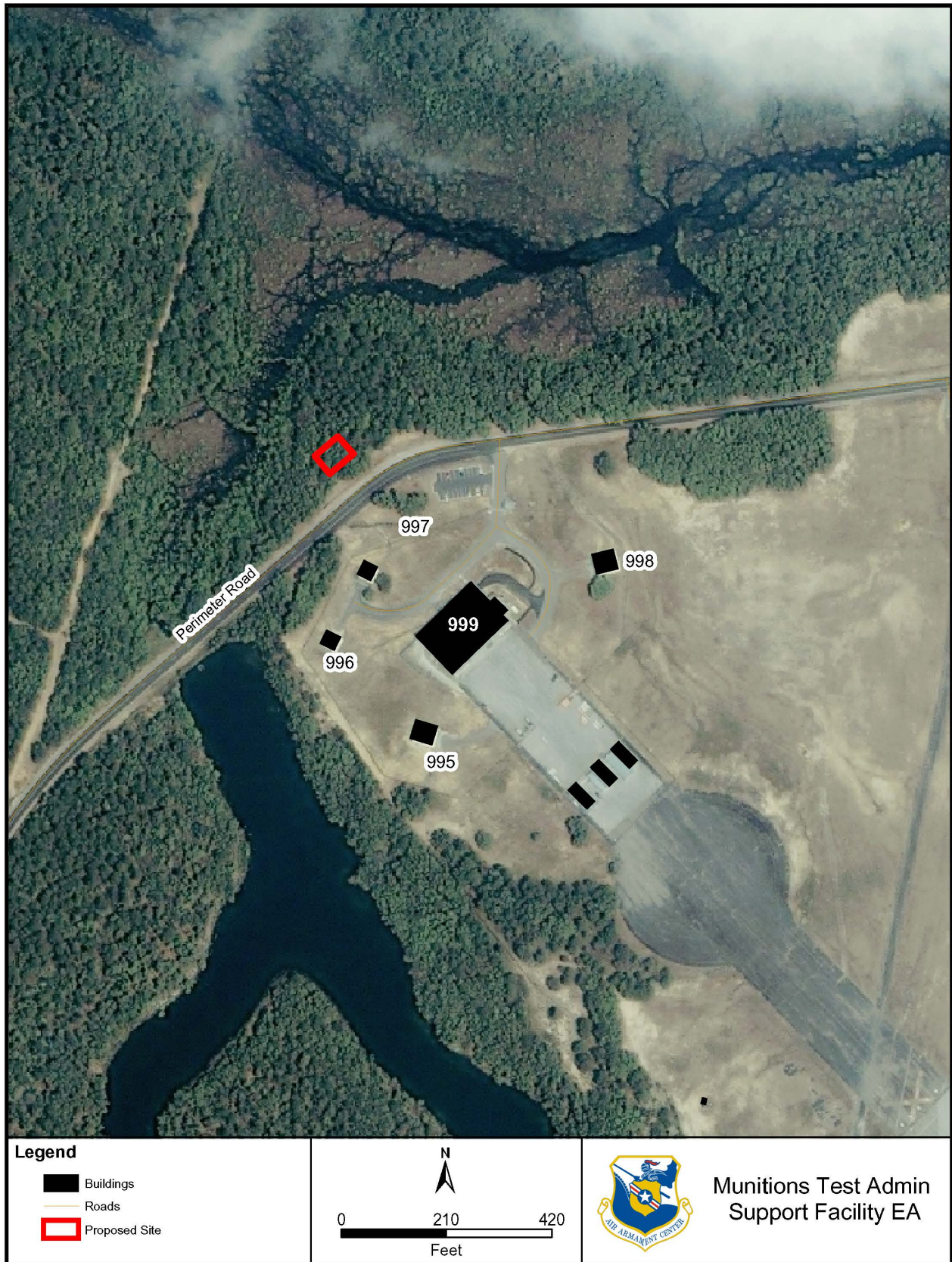
Figure 1-2. Aerial Photograph of Proposed Location
