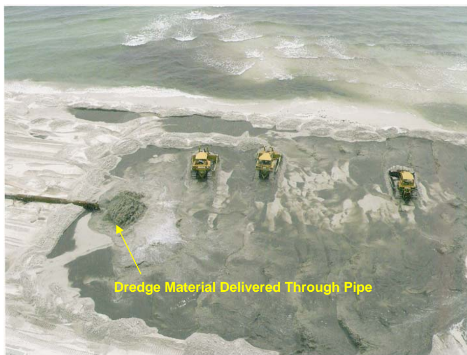
Figure 5-2. Bulldozers Working to Restore the Shoreline in Panama City Beach (Photo Credit: USACE)
