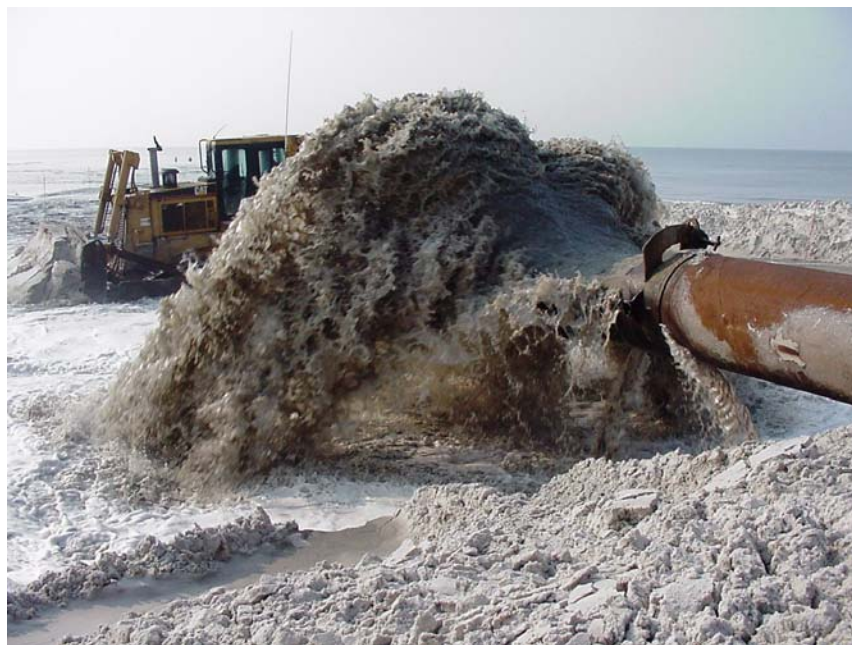
Figure 5-1. Dredged Material Being Delivered to Beach Area (Photo Credit: USACE)
