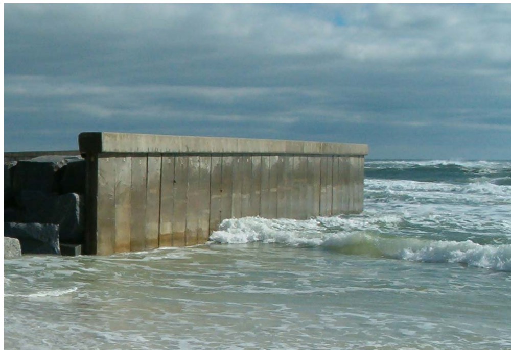
Figure 2-7. Existing Concrete-encased and Capped Sheet Pile Seawall at Test Site A-3
