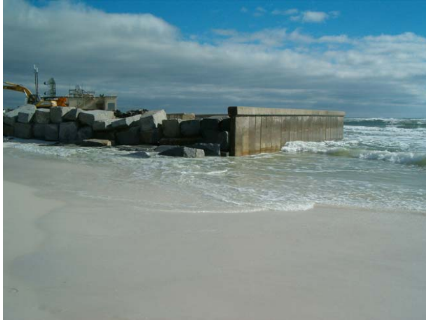
Figure 1-2. Test Site A-3 Seawall and Lack of Beach Area
