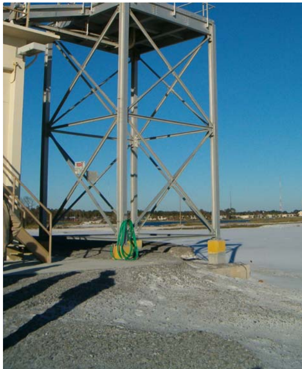
Figure 1-3. Exposed Foundation at Test Site A-6
