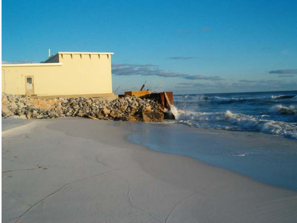
Figure 1-4. Proximity of Test Site A-11 to Waters Edge Illustrating Need for Seawall Extension/Repair
