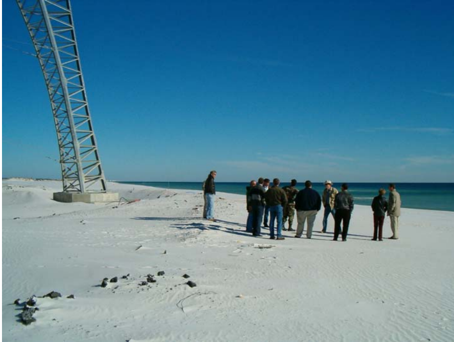
Figure 1-8. South Leg of 300-foot Tower at Test Site A-13B in Proximity to Waters Edge (Illustrates Need for Seawall and Shoreline Restoration)
