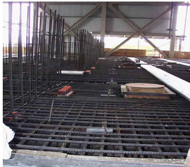
Figure 3. NIF building rebar density in construction.
