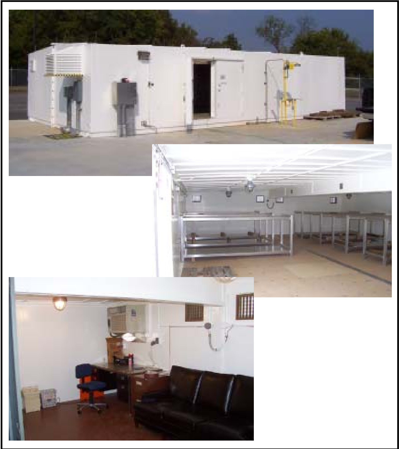
FIGURE 2-1 PROPOSED FACILITY LAYOUT Munitions Maintenance and Inspection Facility at Arnold Air Force Base, Tennessee
