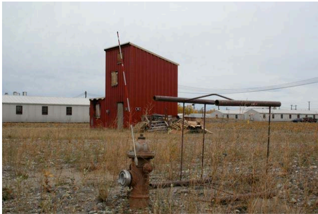
Figure 2. Existing Fire Training Facility, facing southwest.
