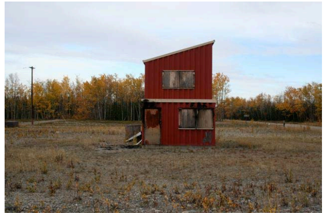
Figure 3. Existing Fire Training Facility, facing north.
