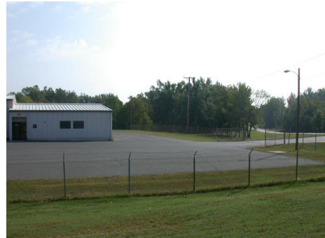
Proposed location for aircraft maintenance hangar. Buildings are scheduled for demolition.
