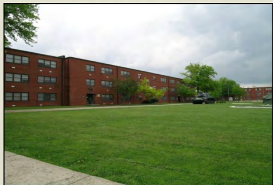
Fort Knox Geothermal Well Field
